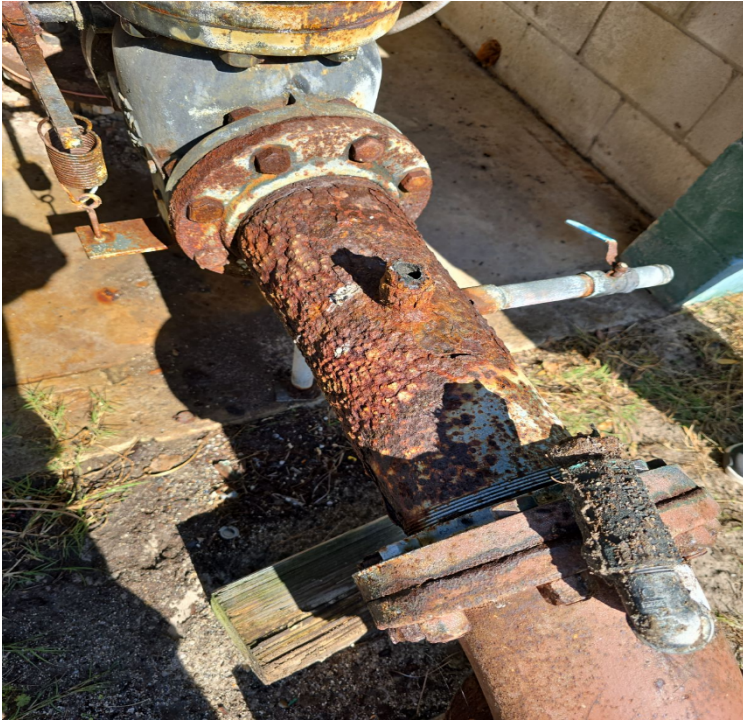
FY27 – 1,200 Foot Deep, 12" Well Rehabilitation ($150,000)
