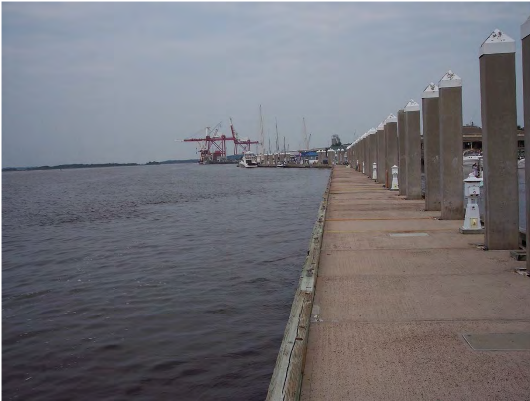
Floating Attenuator Transient Dockage (Offseason)
