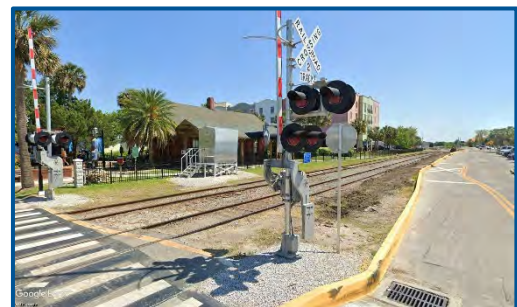
CSX Railroad along Front Street (Source: Google Earth)
