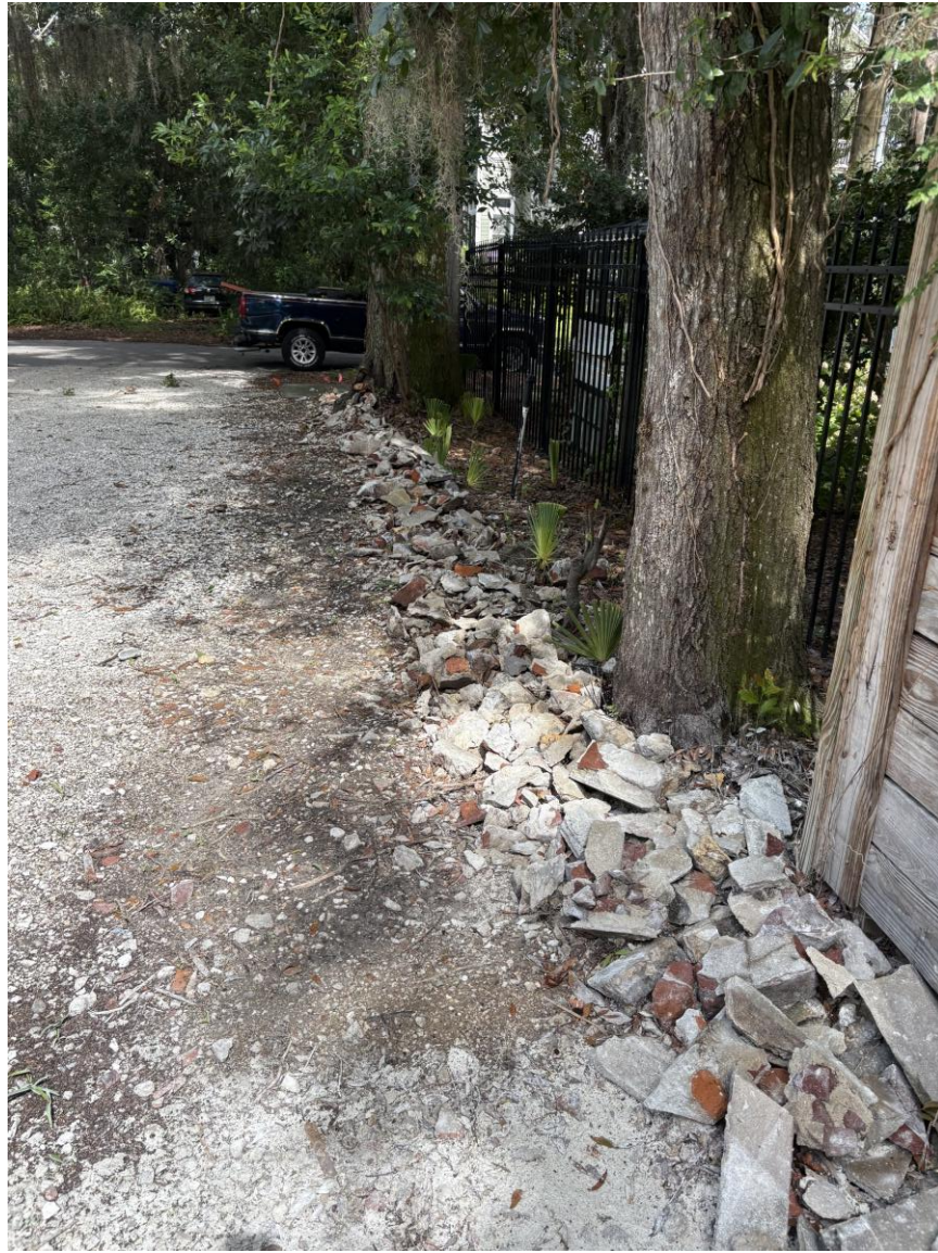
CURB REMOVAL APRIL-MAY 2026
