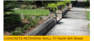
CONCRETE RETAINING WALL 117 North 6th Street
