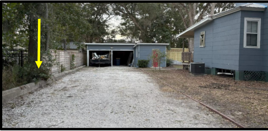
Site wall before demolition:
