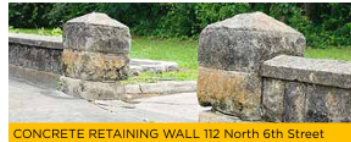
CONCRETE RETAINING WALL 112 North 6th Street
