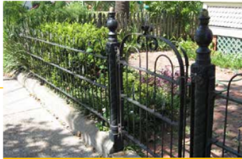
HOOP & DART IRON FENCE 605 Ash Street
