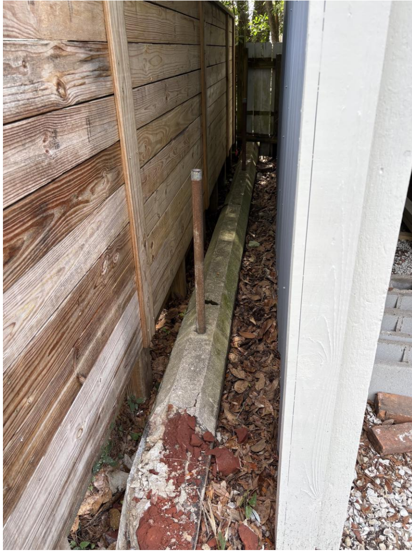
REMAINING NORTH CURB W/ CHAIN LINK POSTS
