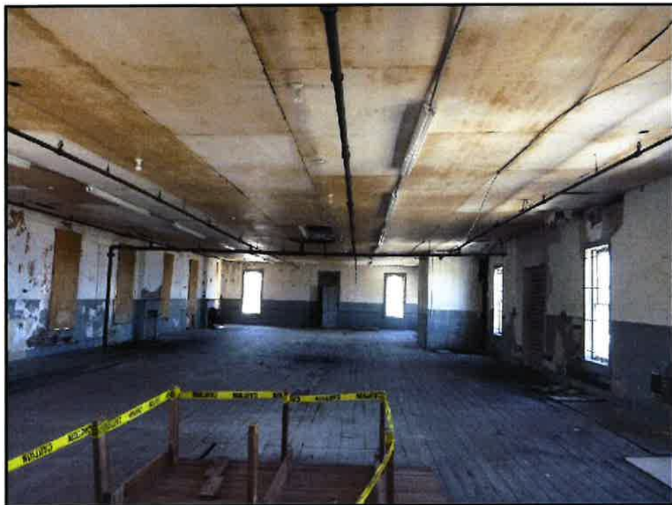
Photo 6 – Wider view of second floor.
