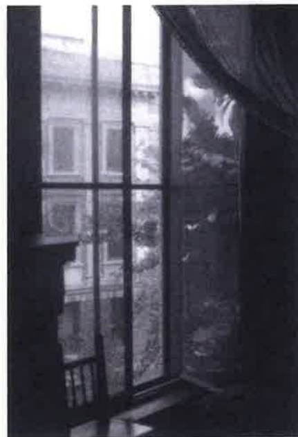
F. Triple glazed windows replaced the originals to control condensation. Photo: © Isabella Stewart Gardner Museum, Boston.
