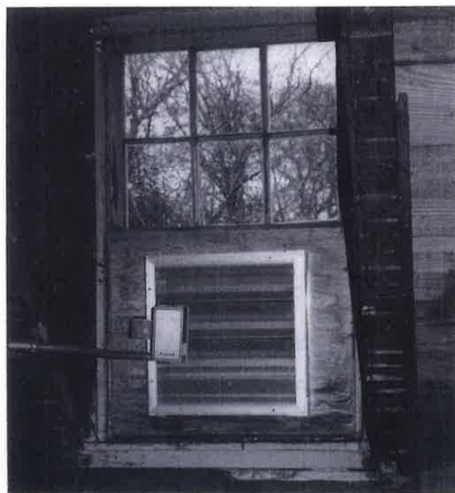
Figure 21. This electric thermostat/humidistat mounted in the attic vent controls a modified ducted air/fan system. The unit uses temporary exposed sheet metal ducts to pull air through the building and exhaust it out of the basement. For over ten years this fan system in combination with 18" x 18" preformed louvers in selective windows has kept the interior dry and with good air exchanges.
