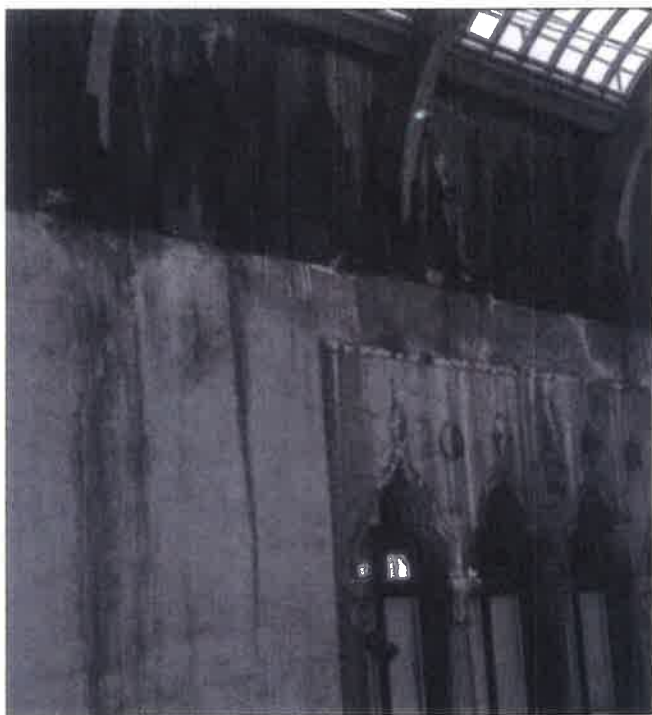
Fig. 7. Condensation dripping from the large overhead courtyard skylight was damaging the masonry in this museum. A new skylight with thermal glazing was installed, replacing the deteriorated single-glazed unit. A new climate control system monitors interior temperature and humidity. Photo: © Isabella Stewart Gardner Museum, Boston.
