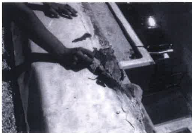
Fig. 1. Moisture problems, if not properly corrected, will increase damage to historic buildings. This waterproof coating trapped moisture from the leaking roof, causing portions of the masonry parapet to fail. Photo: NPS Files.
