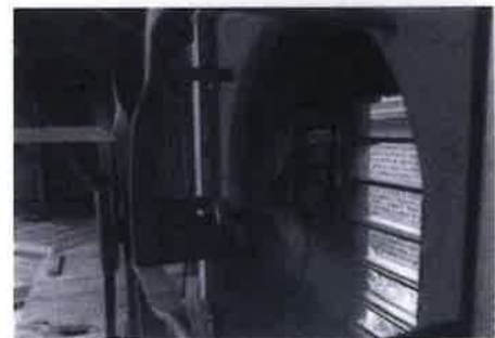
D. Install ventilating fans when additional air circulation will improve damp conditions in buildings or reduce cooling loads. Photo: Ernest A. Conrad, P. E.
