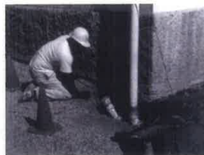
C. Cleaning out gutters and downspouts should be done at least twice a year. Photo: WPTC, NPS.
