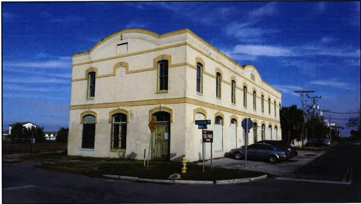
Photo 1 – Southeast corner of building.
