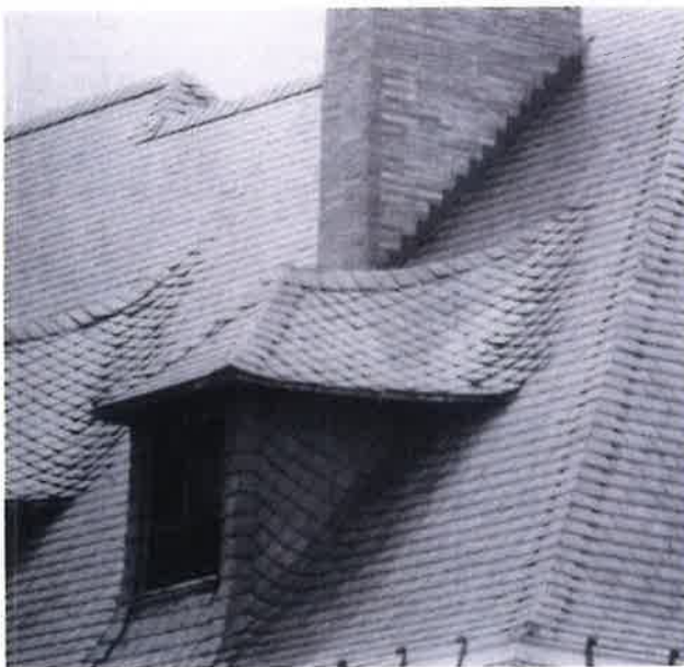
Because of the roof's visibility, the slate detailing around the dormers is important to the character of this structure. Note how the slates swirl from a horizontal pattern on the main roof to a diamond pattern on the dormer roofs and side walls. (18th and Que Streets, NW, Washington, D.C.)
