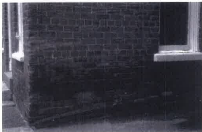
Fig. 11. Capillary rise of moisture in masonry is often accompanied with a horizontal tide-mark line several feet above the grade, as seen here. Removing or redirecting as much ground moisture as possible usually helps reduce moisture within a wall. Photo: NPS Files.
