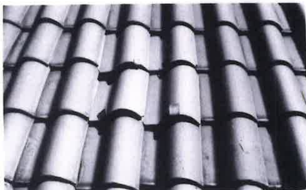
Repairs on this pantile roof were made with new tiles held in place with metal hangers. (Main Building, Ellis Island, New York)
