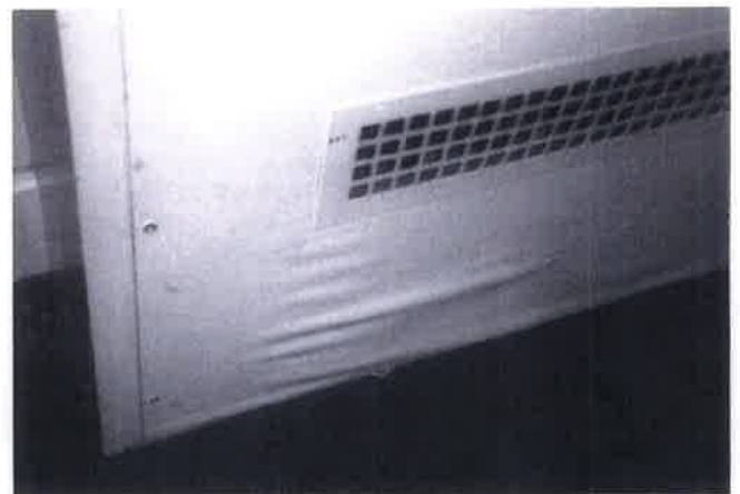
Fig. 3. The deterioration of this wooden cover was a sign that water was leaking from the fan coil unit behind. Photo: author.
