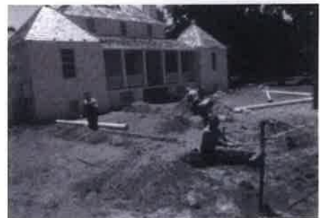
C. Develop new drainage systems for roof run-off that remove moisture from the base of the building. Photo: WPTC, NPS.
