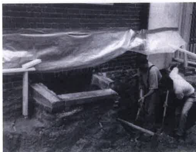
Fig. 5. Excavating this foundation revealed that the downspout pipe had corroded at the "u-trap" and was leaking moisture into the soil. Openings around the horizontal water supply line and cracks in the wall allowed moisture to penetrate the basement in multiple locations. Photo: author.
