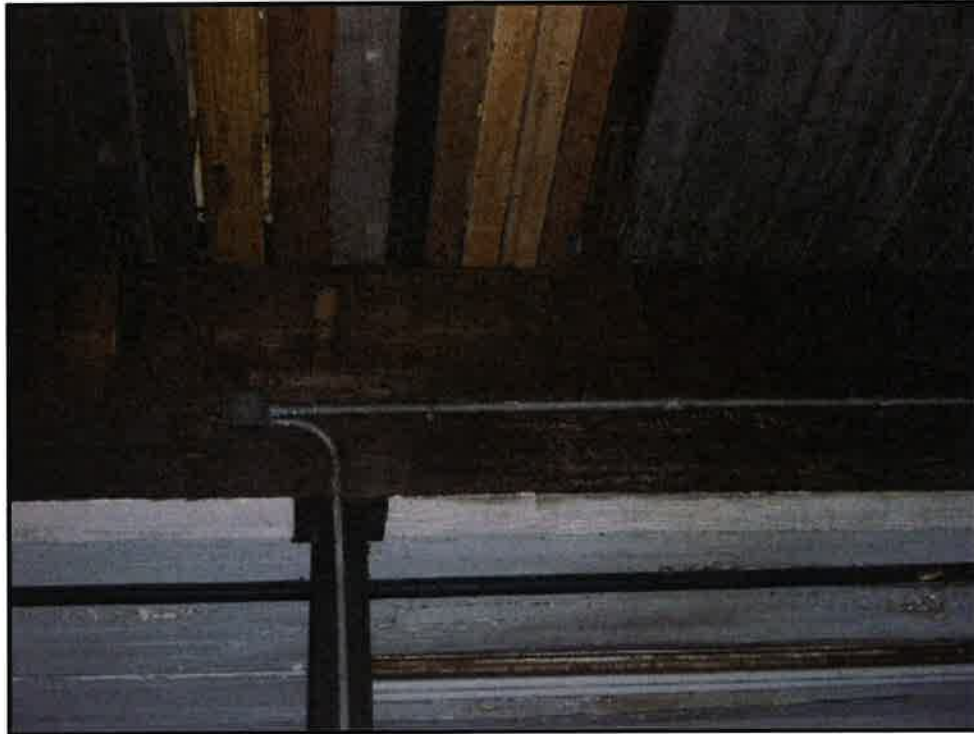
Photo 3 – Wood beam above first floor still in good condition.
