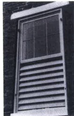
Figure 18. Heavy duty wooden slated louvers were custom fabricated to replace the deteriorated lower sash. The upper sash were rebuilt to retain the historic appearance and to allow light into this vacant historic building. Refer back to Fig. 1 for a view of the building. Photo: Charles E. Fisher, NPS. Drawing by Thomas Vitanza.
