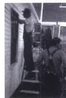
B. Repair exterior surfaces, paint, and recaulk as needed. Photo: Williamsport Preservation Training Center (WPTC), NPS.
