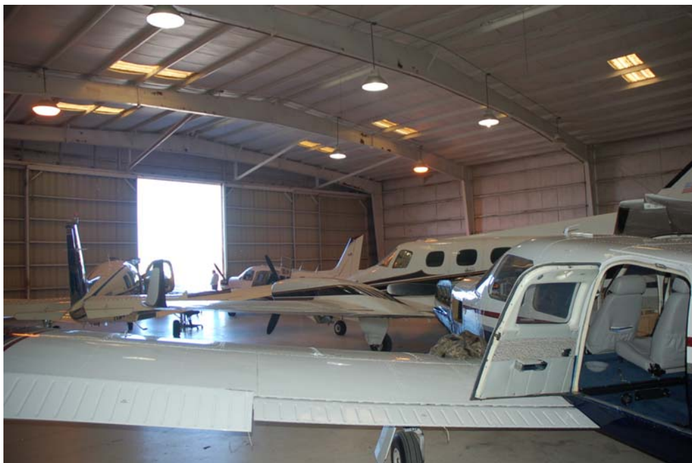
Interior view of the hangar.
