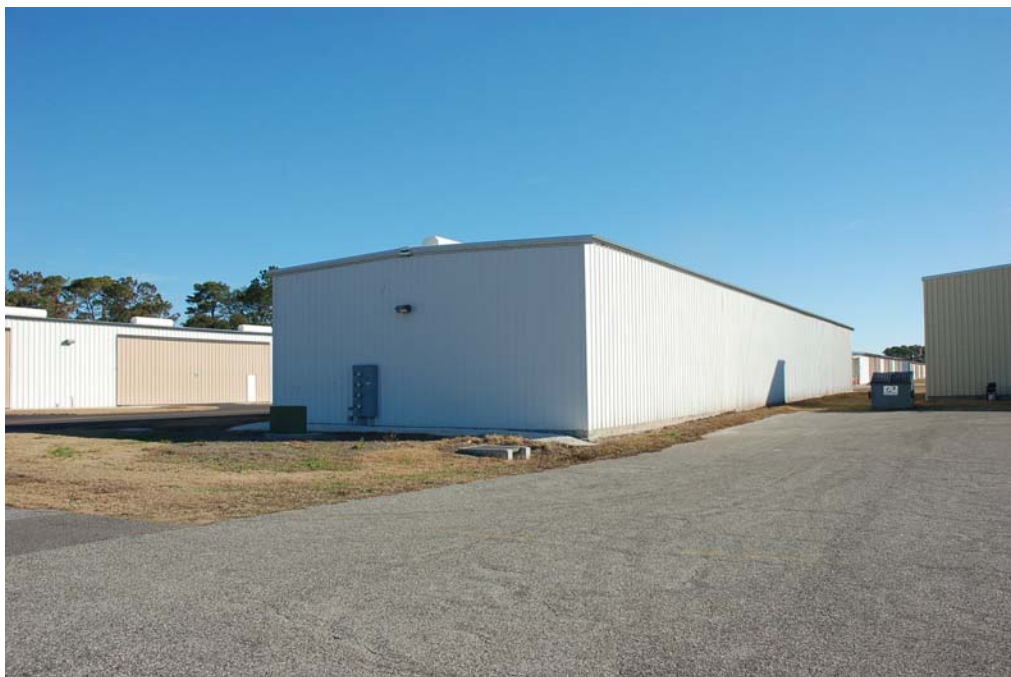
View of the south and west elevations.
