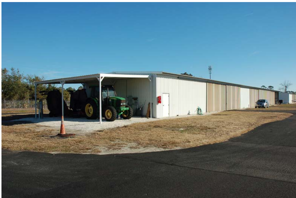
View of the south and west elevations.
