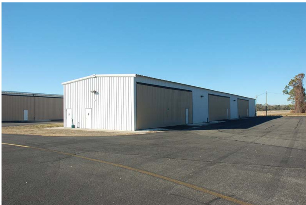
View of the north and east elevations.
