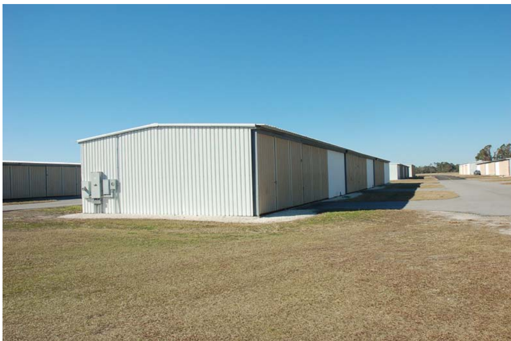
View of the north and east elevations.
