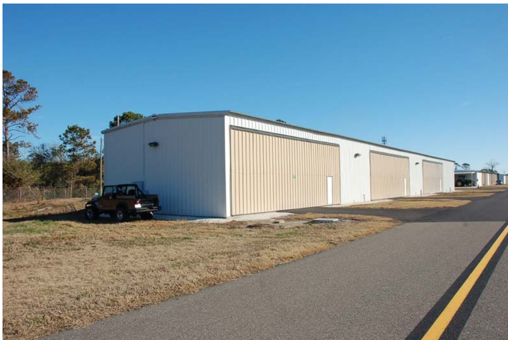
View of the south and west elevations.
