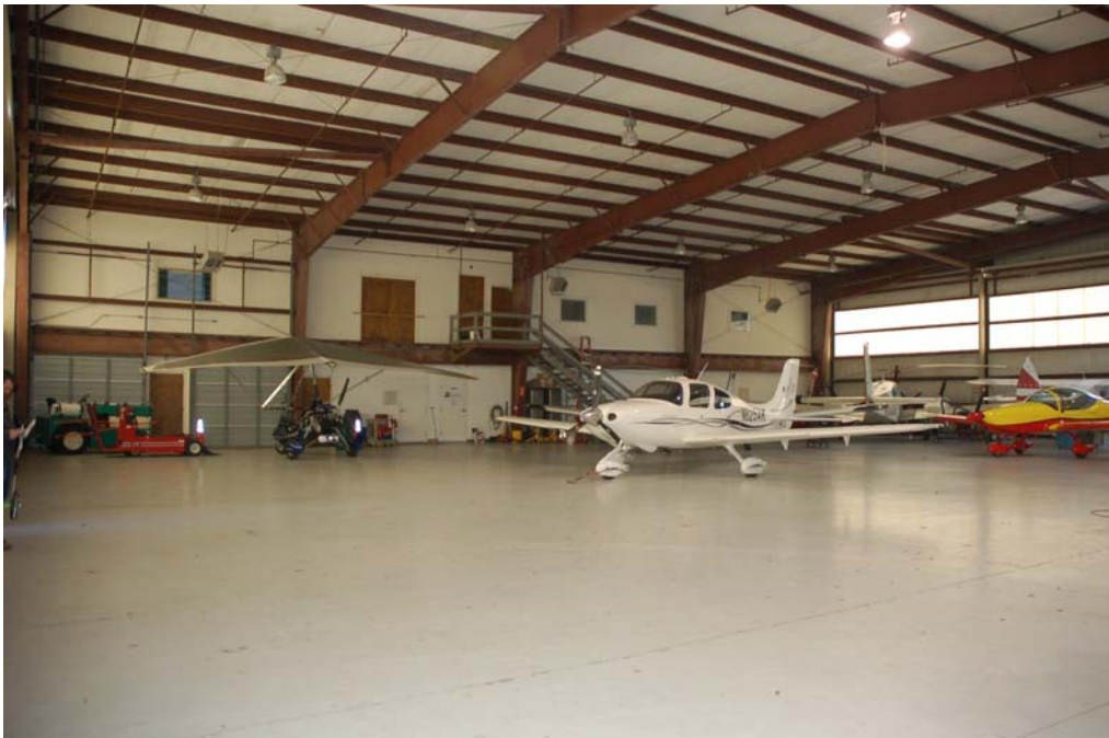
Interior view of the hangar area.
