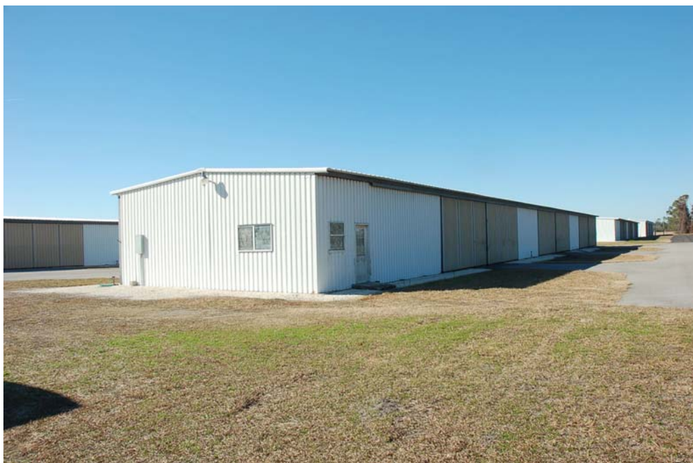
View of the north and east elevations.
