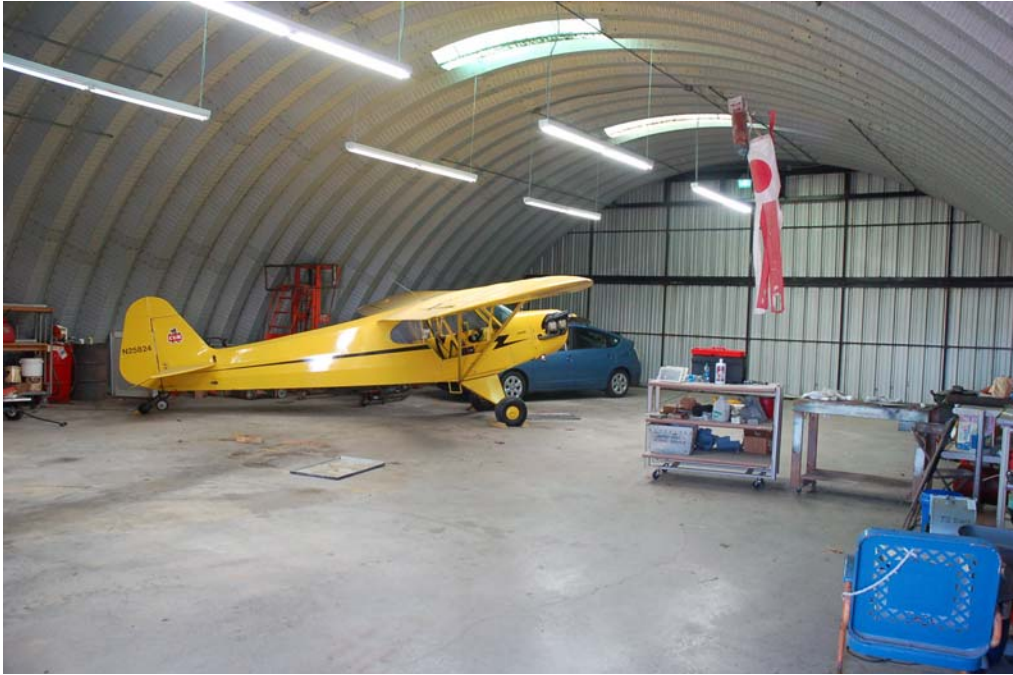
Interior view of the hangar.
