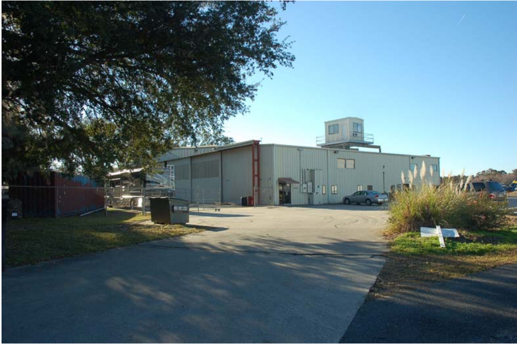
View of the north and east elevations.
