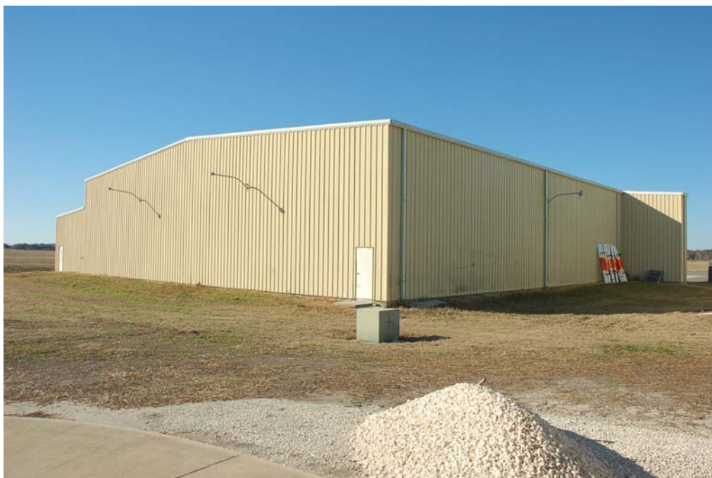
View of the north and east elevations.
