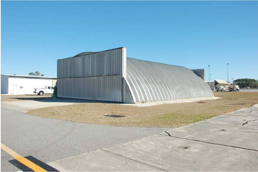
View of the south and west elevations.
