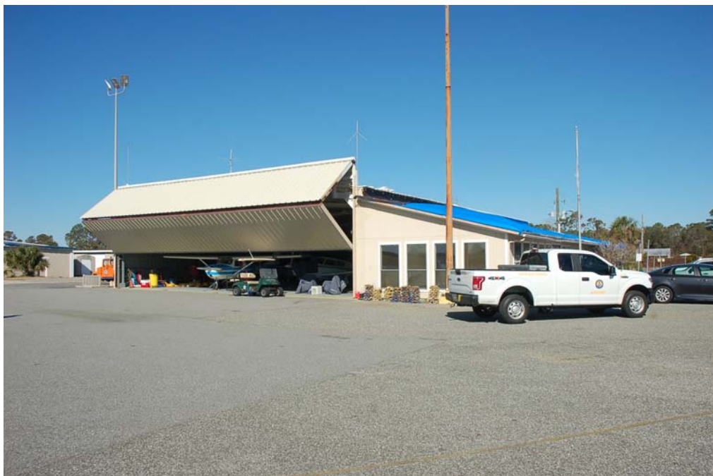
View of the south and east elevations.
