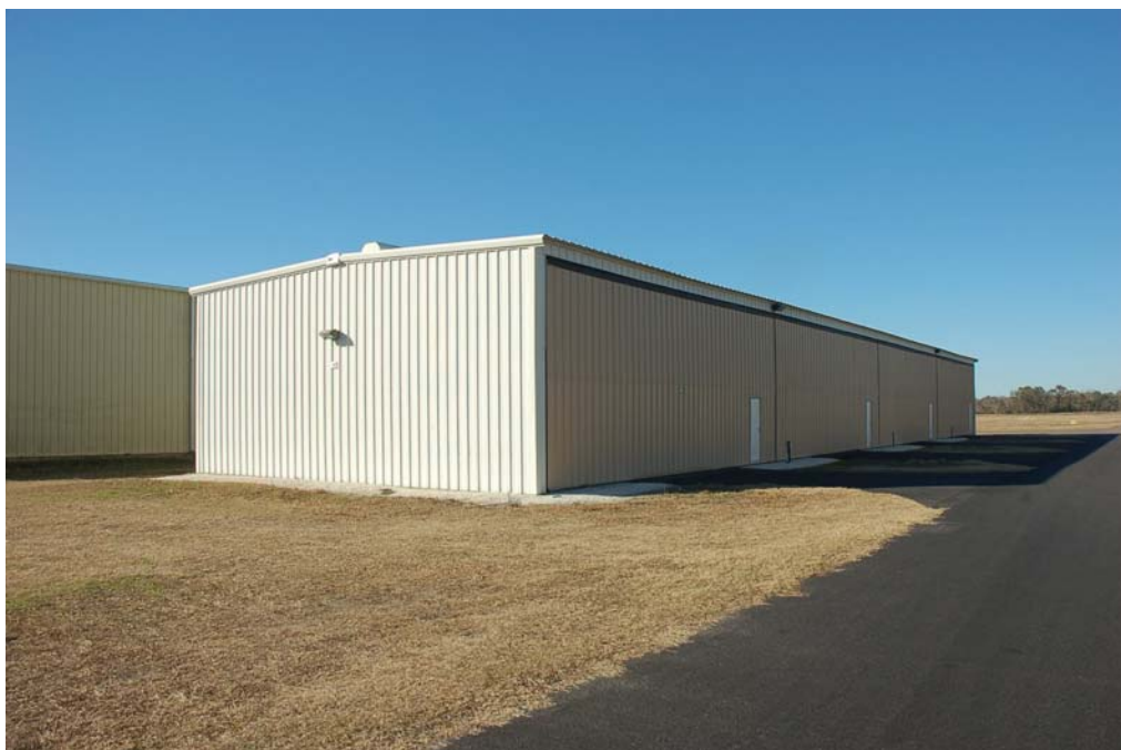
View of the north and east elevations.
