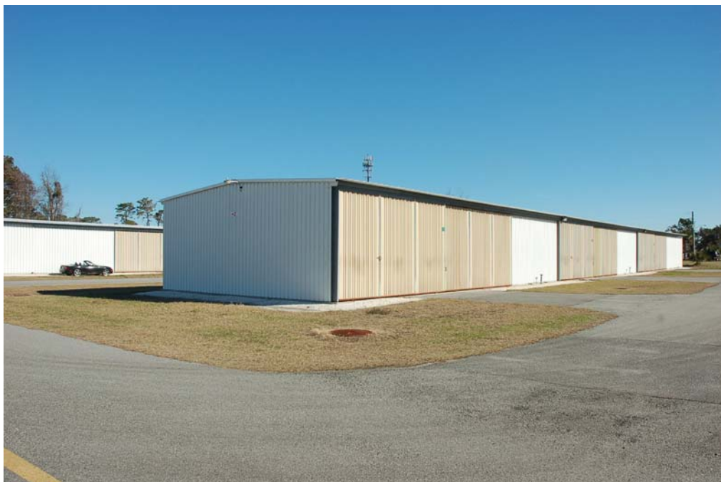
View of the south and west elevations.
