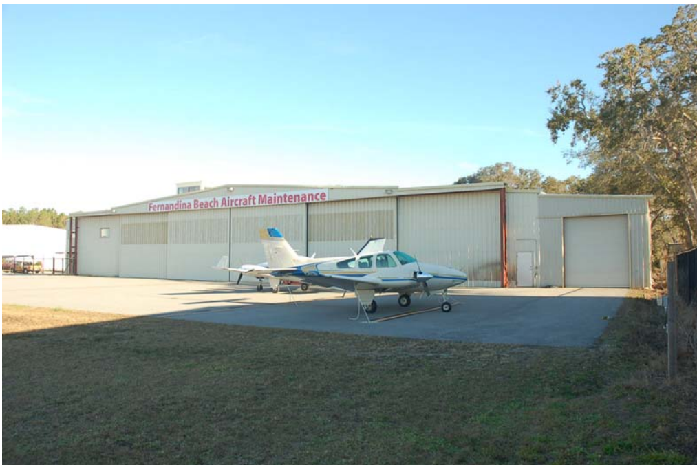
View of the south and west elevations.
