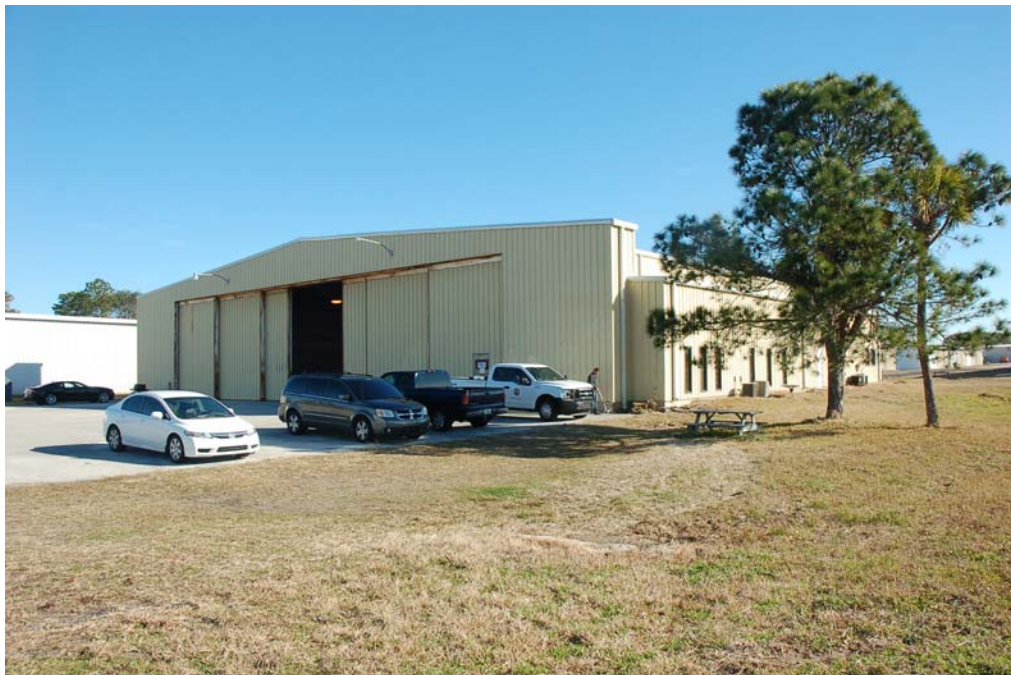
View of the south and west elevations.
