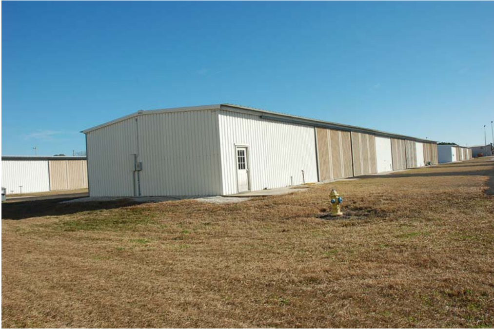
View of the south and west elevations.
