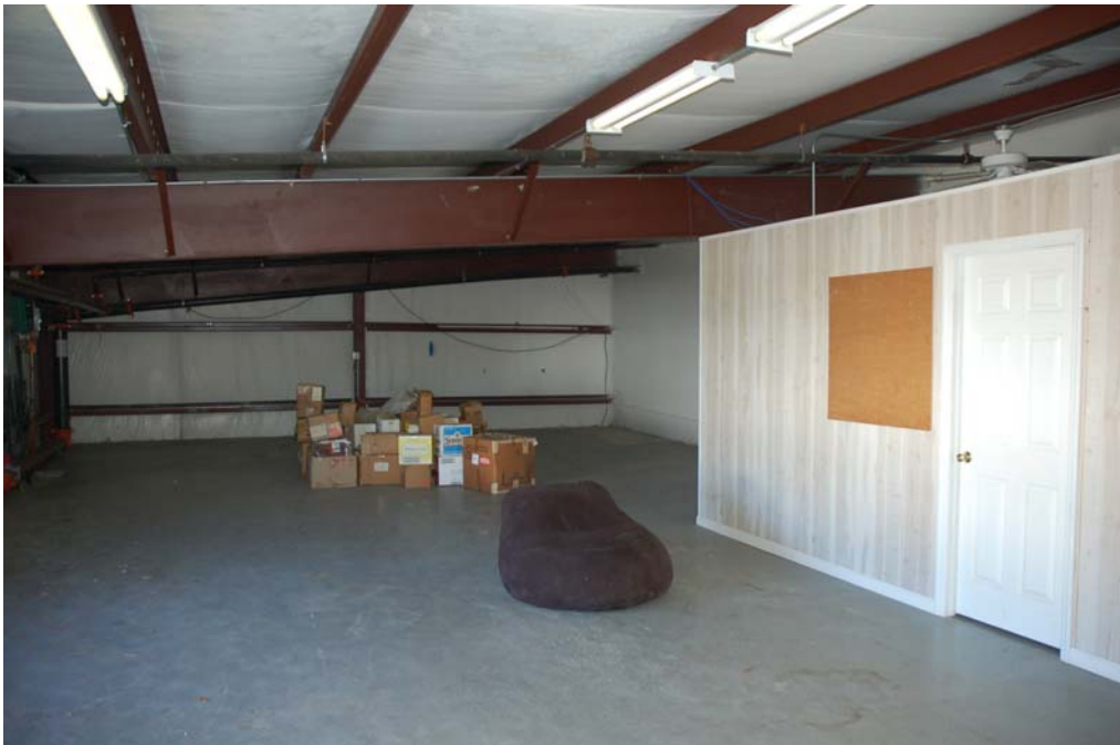
Typical view of storage mezzanine.
