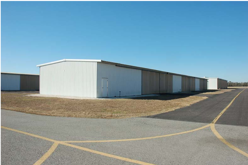
View of the north and east elevations.
