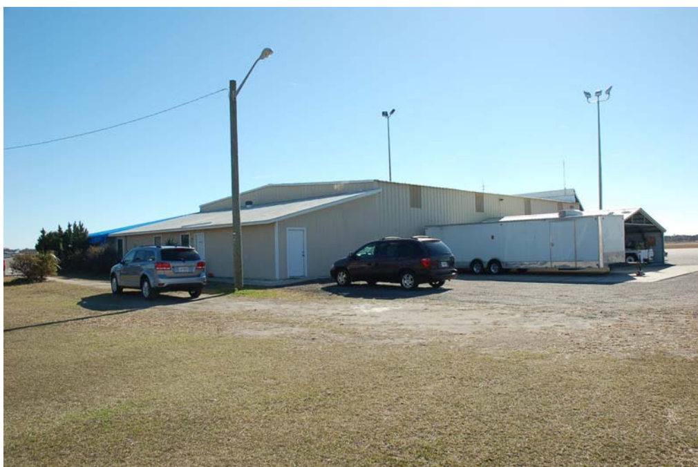
View of the north and west elevations.
