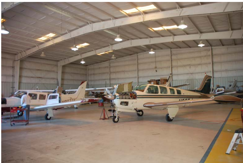
Interior view of the hangar.
