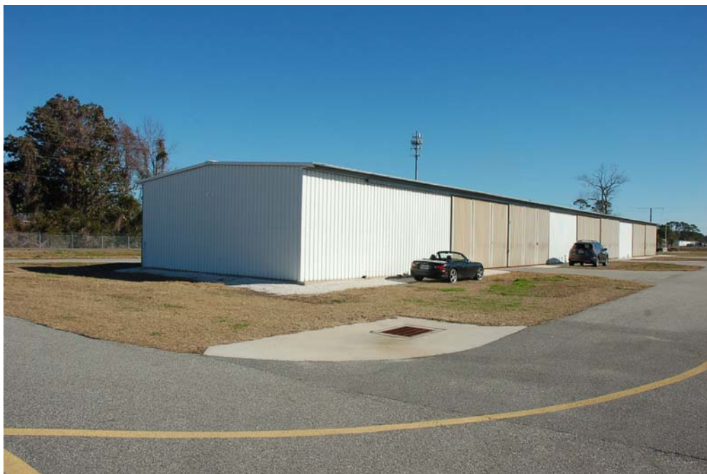
View of the south and west elevations.
