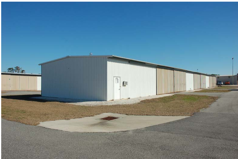
View of the south and west elevations.
