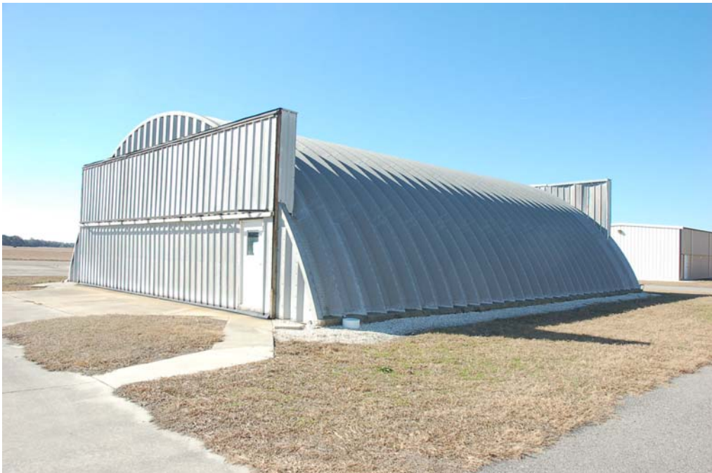
View of the south and west elevations.
