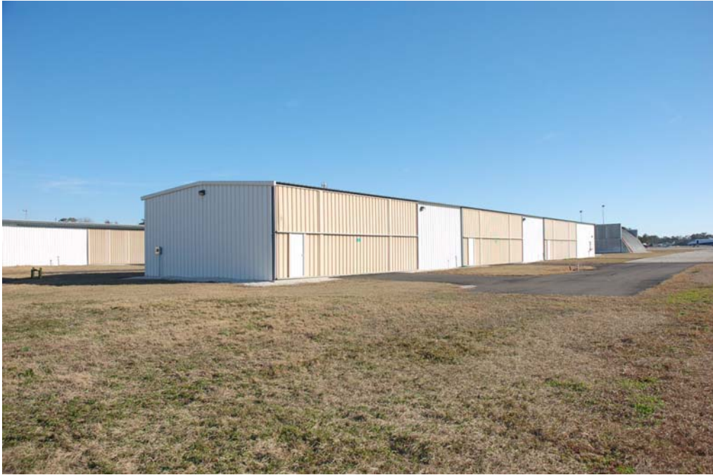
View of the south and west elevations.
