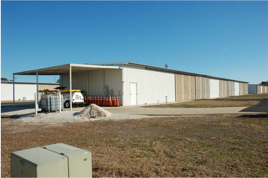
View of the south and west elevations.
