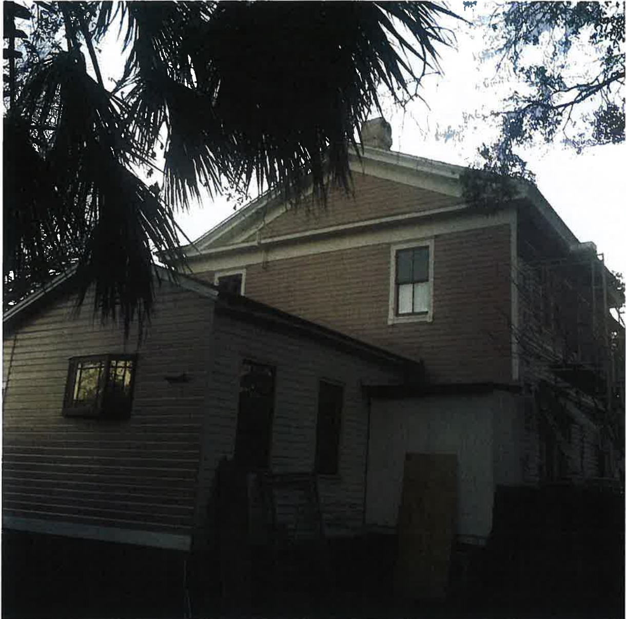
Southwest corner Location of new porch and side entry
