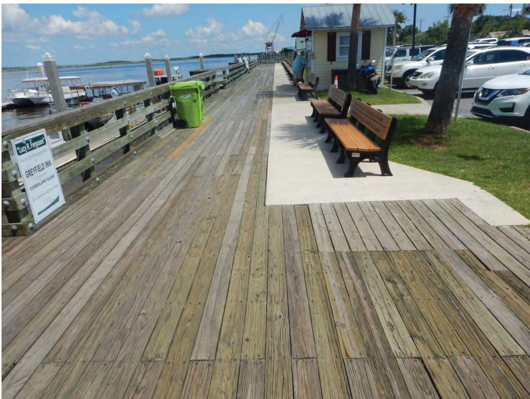
Photo 6 – Begin of Steel Sheet Pile Wall Limits Looking North
