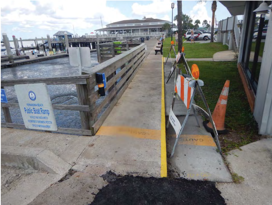
Photo 1 – Begin of Concrete Wall looking North from Boat Ramp
