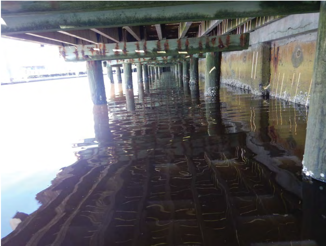
Photo 3 – Typical View of Concrete Wall and Underside of Timber Boardwalk Looking North
