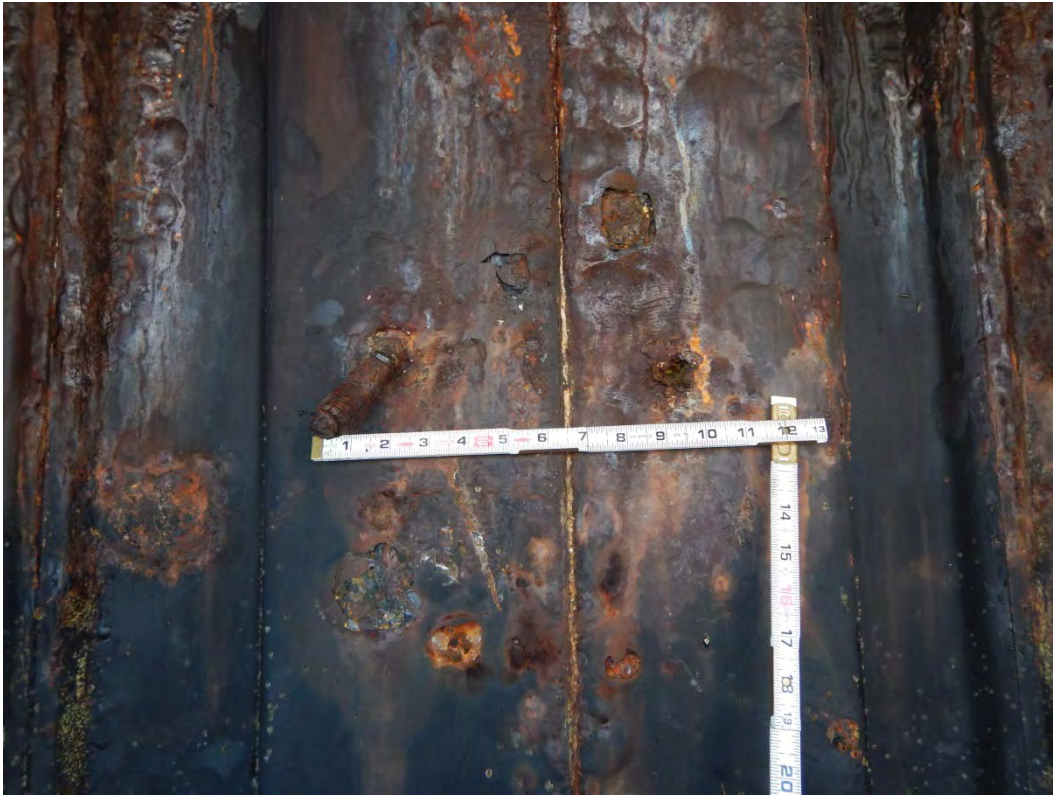
Photo 21 – Typical Partially Sealed Pre-drilled Holes in Steel Sheet Pile Wall
