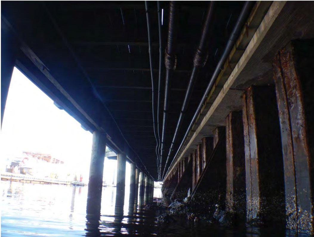
Photo 9 – Typical View of Steel Sheet Pile Wall and Underside of Timber Boardwalk Looking North
