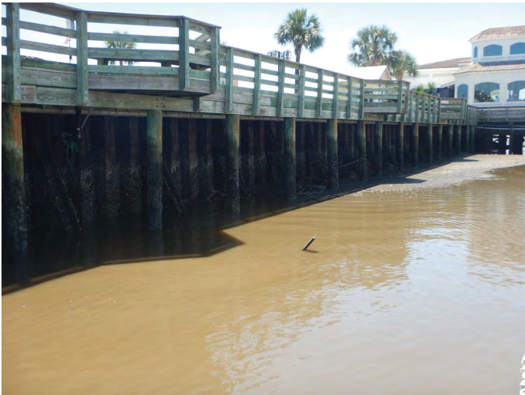
Photo 8 – Typical Steel Sheet Pile Wall Looking South
