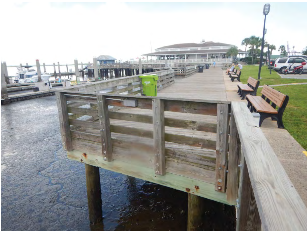
Photo 2 – Begin of Timber Boardwalk at Concrete Wall Looking North
