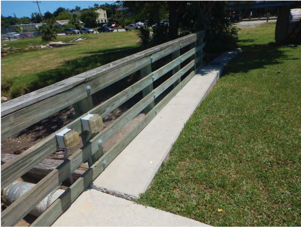
Photo 7 –Steel Sheet Pile Wall Extension Looking East
