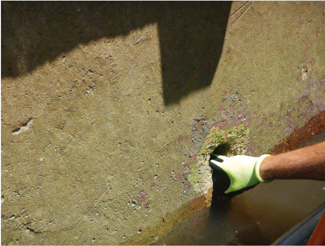
Photo 13 – Typical Open Weephole for Concrete Seawall
