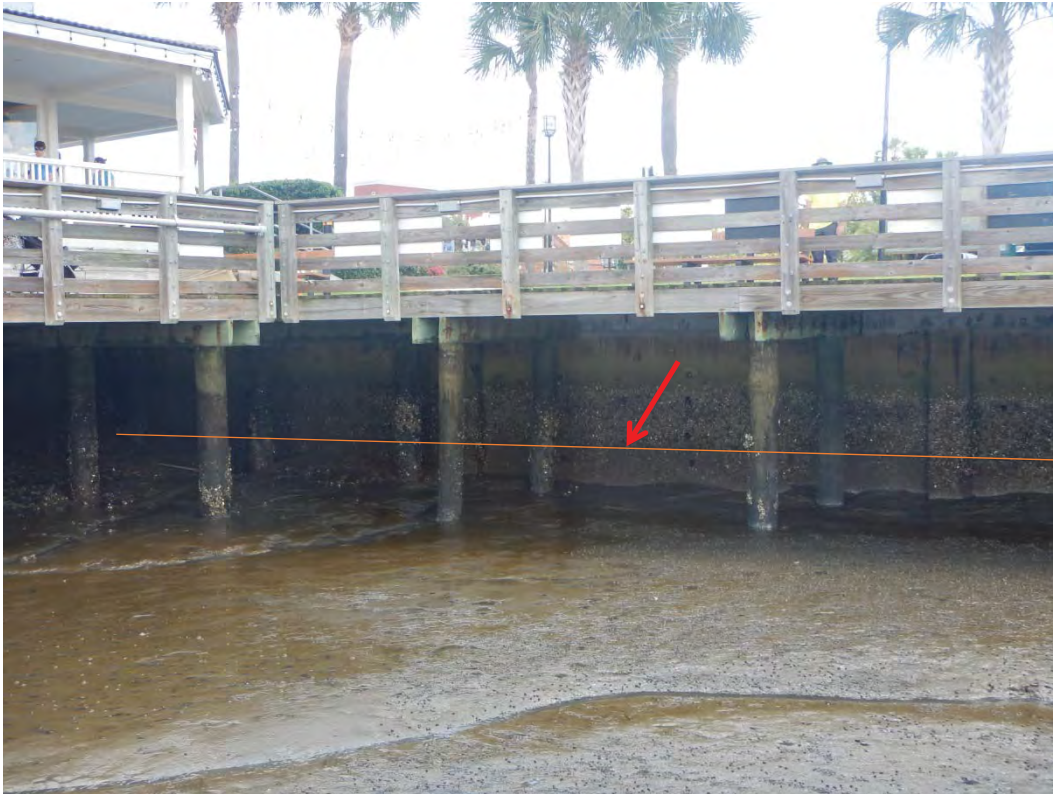
Photo 5 – Typical Concrete Wall showing Horizontal Joints between Precast Sections
