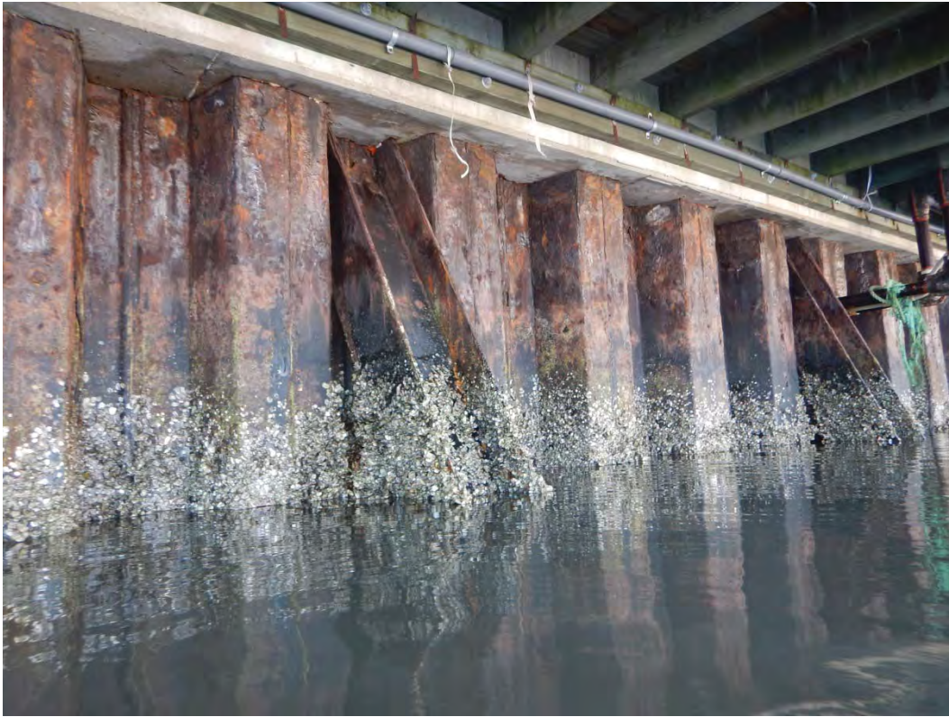
Photo 19 – Typical Condition of Steel Sheet Pile Wall
