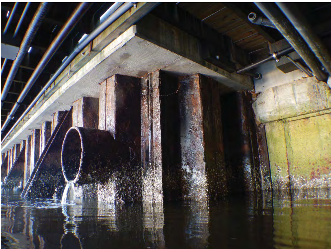
Photo 10 – Begin of Steel Sheet Pile Wall and Drainage Pipe Penetration
