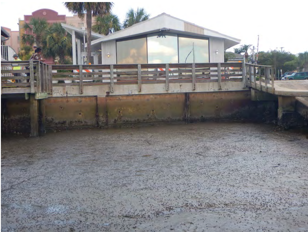
Photo 4 – Typical Concrete Wall Looking East. Photo Taken During Low Tide
