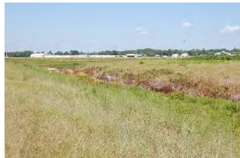
Photo 2B. Drainage ditch on FHB. Lacking proper maintenance with ample vegetation to provide cover.
