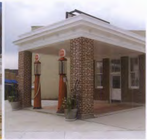
Figures 18. The canopy of the 1920s Spruce Street Station in Ogallala, NE, was an important feature that contributed to the building's character (left). When recently purchased for rehabilitation the canopy had long since disappeared (center). Using photographic and physical evidence, the canopy was reconstructed to match the building's original appearance (right). The station currently functions as a Main Street program office, a visitor center (on Nebraska's Western Trails Historic and Scenic Byway as well as Lincoln Highway Scenic Byway), meeting room, and public restroom facility. Photo: Ogallala Main Street.
