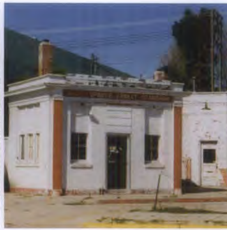
Figures 18. The canopy of the 1920s Spruce Street Station in Ogallala, NE, was an important feature that contributed to the building's character (left). When recently purchased for rehabilitation the canopy had long since disappeared (center). Using photographic and physical evidence, the canopy was reconstructed to match the building's original appearance (right). The station currently functions as a Main Street program office, a visitor center (on Nebraska's Western Trails Historic and Scenic Byway as well as Lincoln Highway Scenic Byway), meeting room, and public restroom facility. Photo: Ogallala Main Street.
