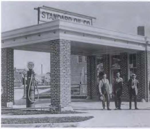
Figures 18. The canopy of the 1920s Spruce Street Station in Ogallala, NE, was an important feature that contributed to the building's character (left). When recently purchased for rehabilitation the canopy had long since disappeared (center). Using photographic and physical evidence, the canopy was reconstructed to match the building's original appearance (right). The station currently functions as a Main Street program office, a visitor center (on Nebraska's Western Trails Historic and Scenic Byway as well as Lincoln Highway Scenic Byway), meeting room, and public restroom facility. Photo: Ogallala Main Street.
