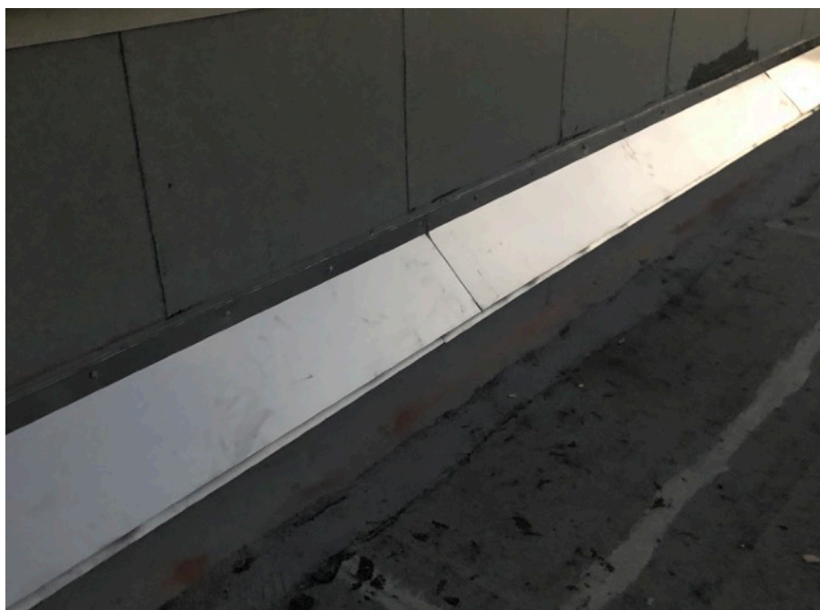
Overview of two-two-piece metal expansion joint.
