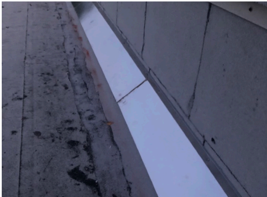
Overview of two-piece metal expansion joint.
