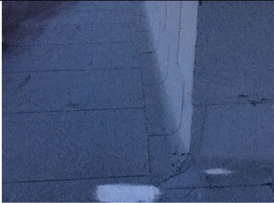
Overview of existing transition.
