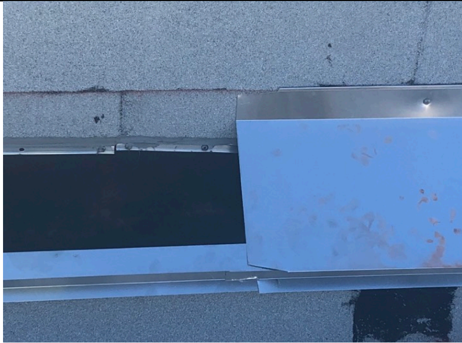
Overview of two-piece metal expansion joint.
