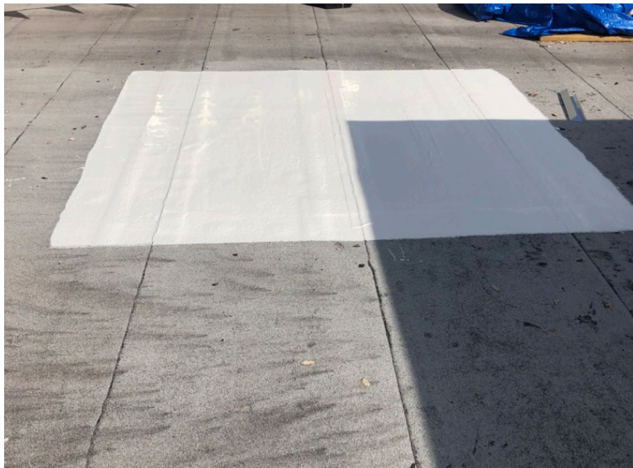
Overview of completed Alphaguard BIO Top Coat.
