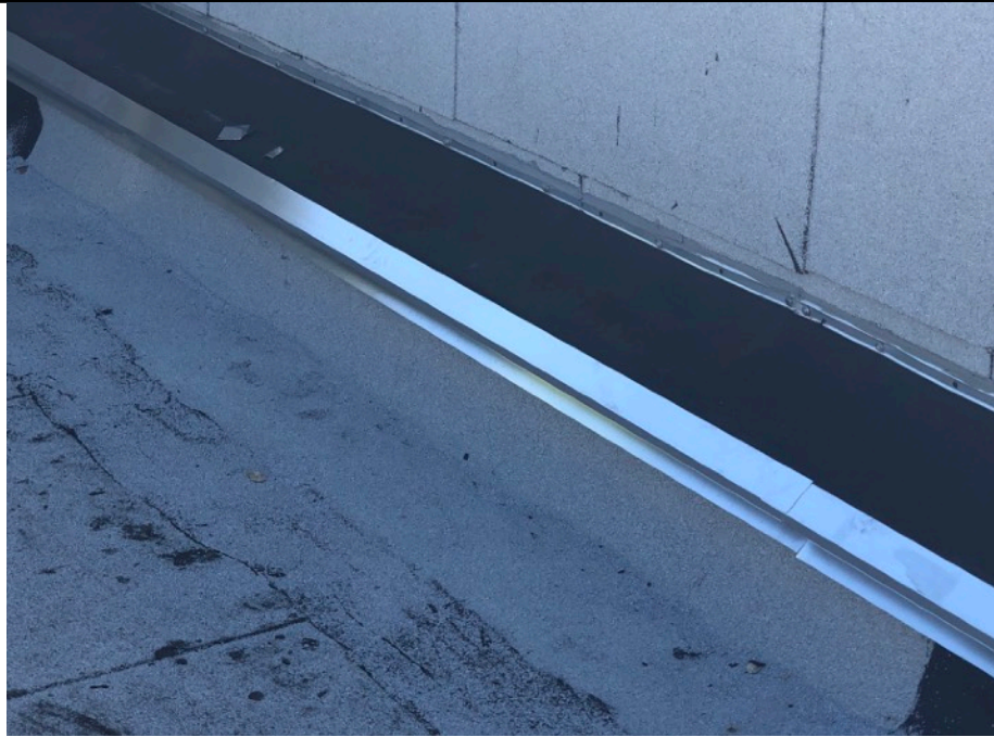
Sheet metal cleat installed 12" on center.
