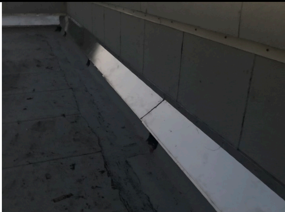
Overview of two-piece metal expansion joint.
