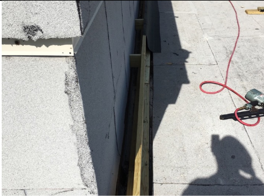
Wood nailer fastened to masonry wall.
