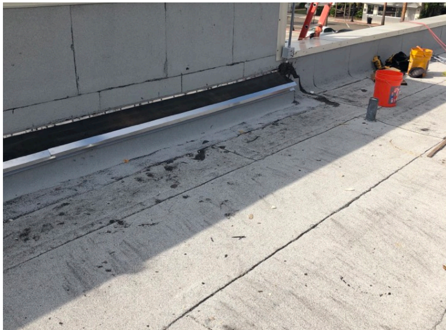
Overview of sheet metal cleat.
