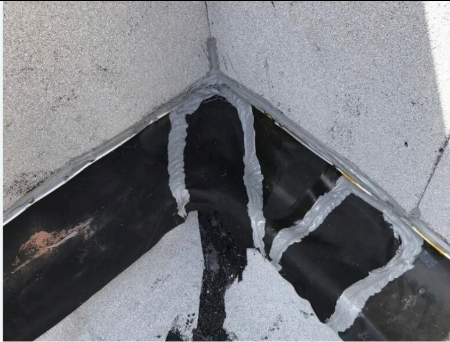
TremSeal PRO applied to transition over rubber seal.
