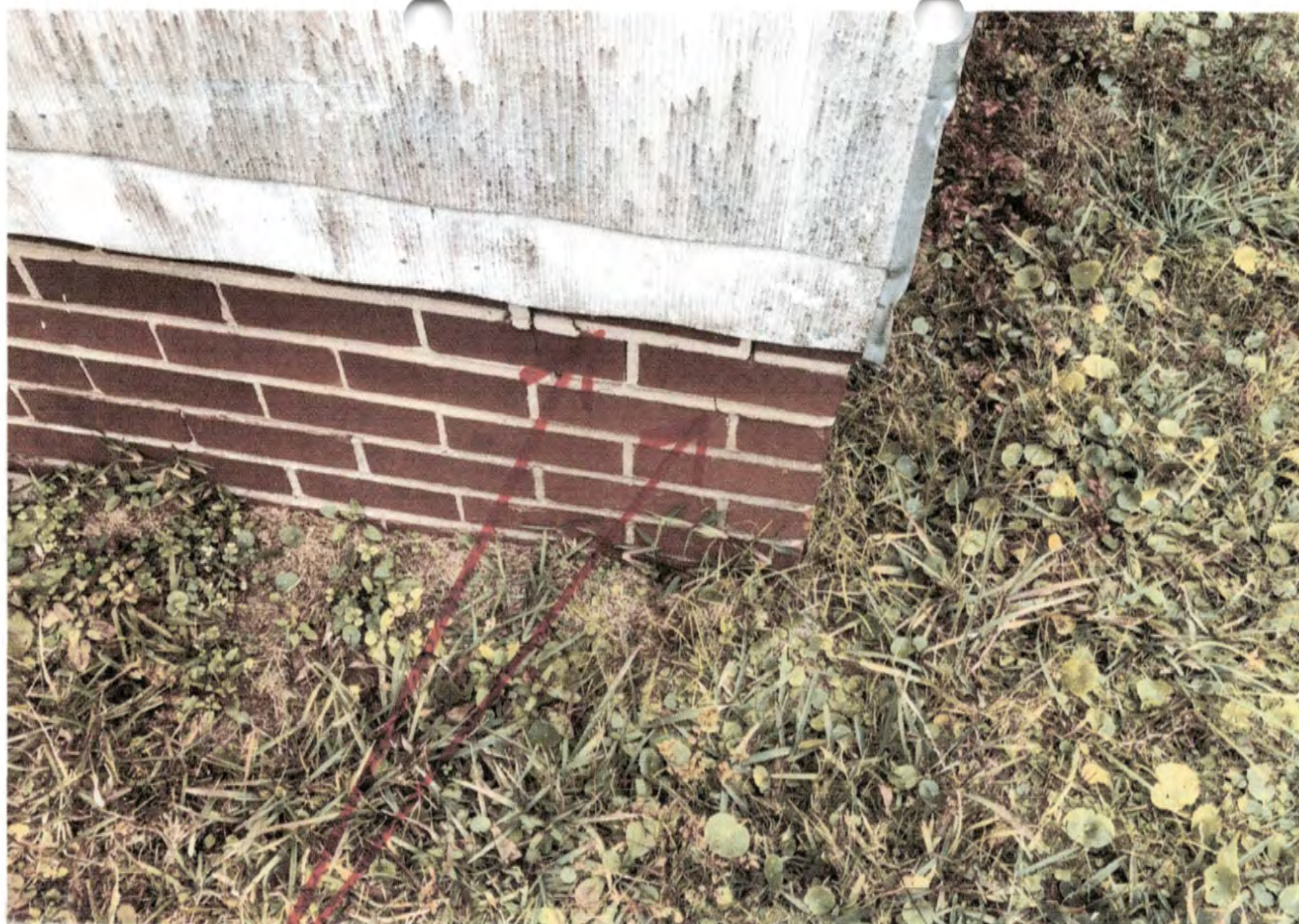
Cracked & Buckled Brick stem wall
