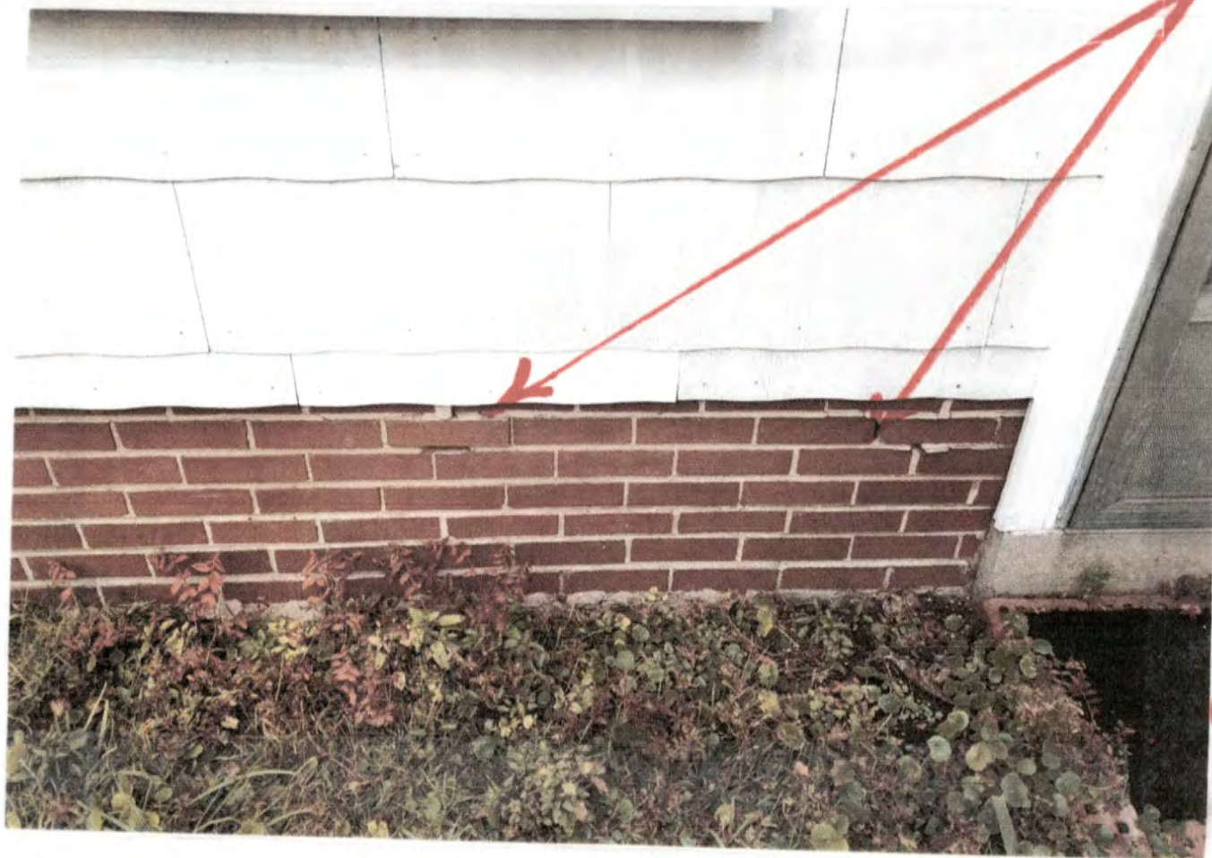
Cracked & Buckled Brick stem wall
