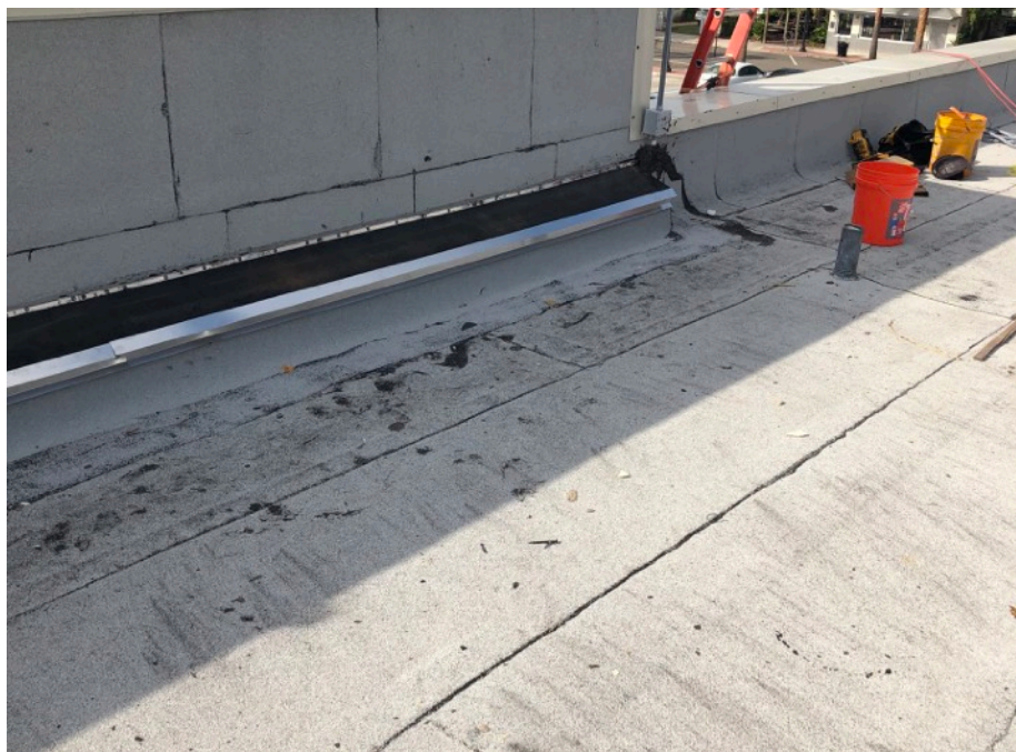
Overview of sheet metal cleat.
