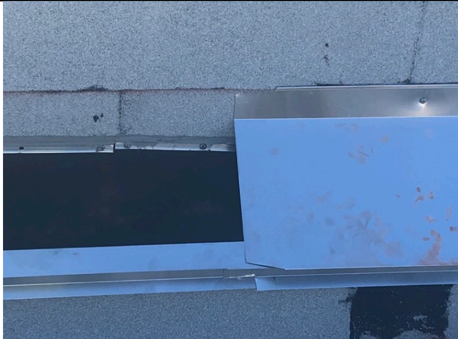
Overview of two-piece metal expansion joint.
