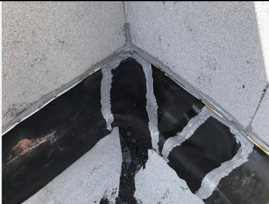
TremSeal PRO applied to transition over rubber seal.
