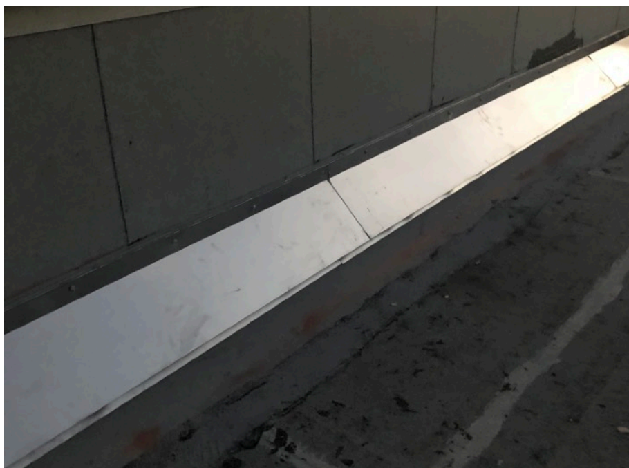
Overview of two-two-piece metal expansion joint.
