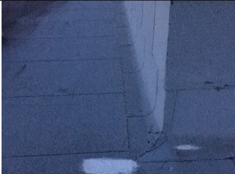
Overview of existing transition.
