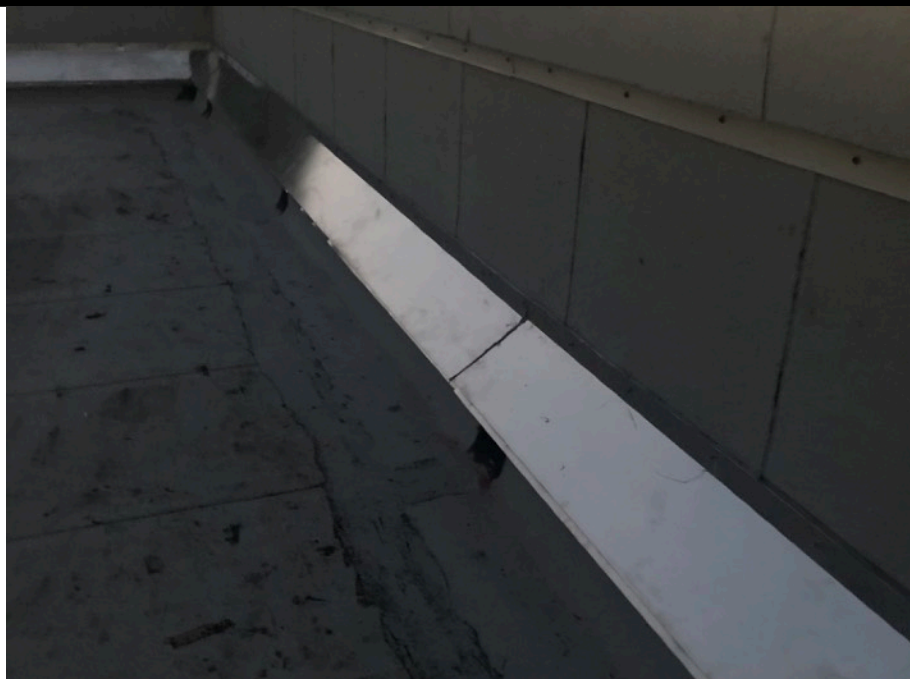
Overview of two-piece metal expansion joint.
