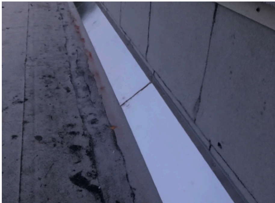
Overview of two-piece metal expansion joint.
