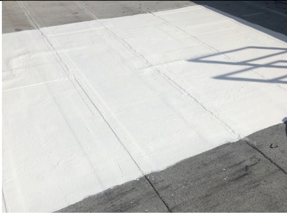
Overview of completed Alphaguard BIO Top Coat.
