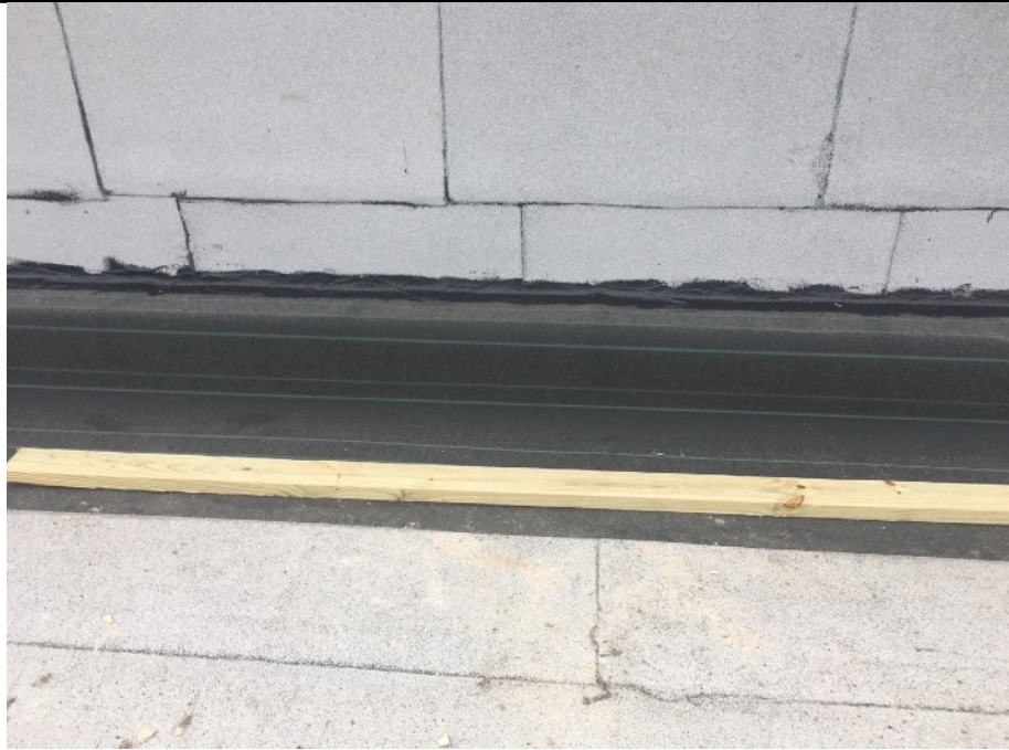
Composite ply HT installed over wood nailer.
