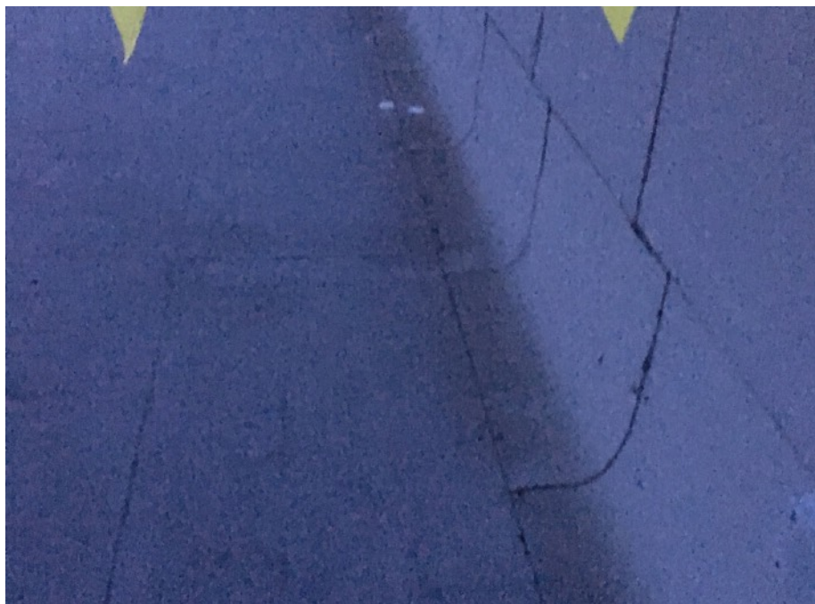
Overview of existing transition.
