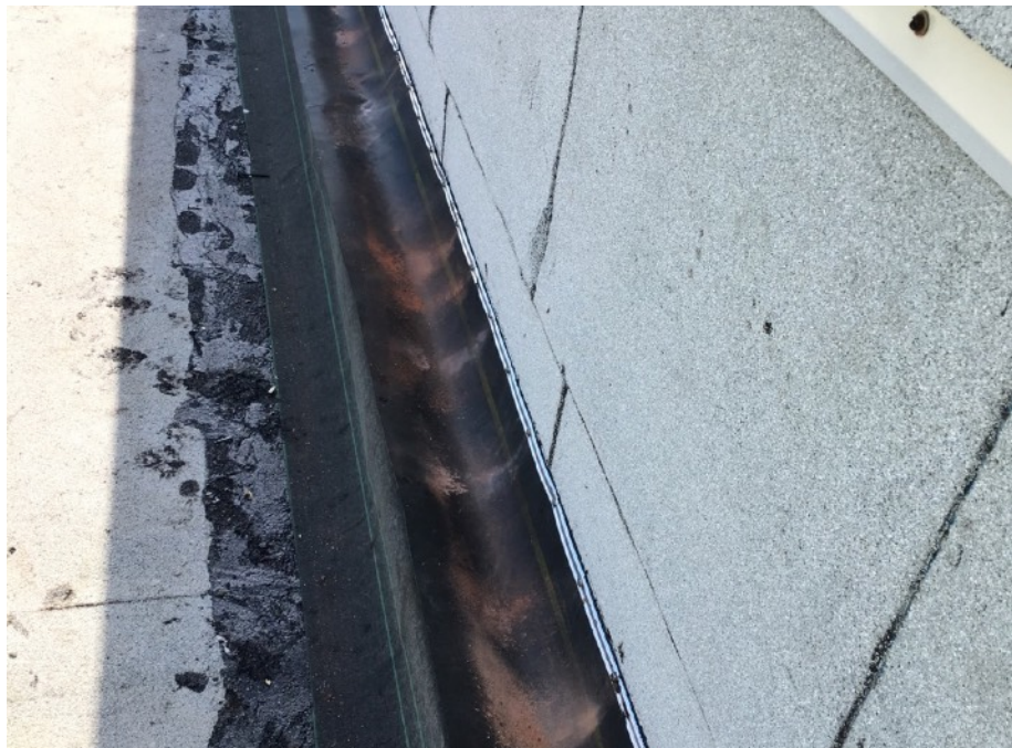
Composite ply HT installed over wood nailers.
