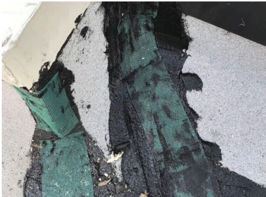
3-course mastic with mesh over PowerPly Standard Cap sheet
