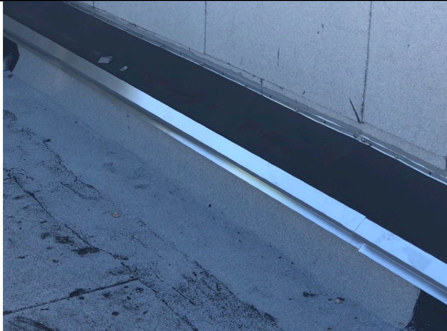
Sheet metal cleat installed 12" on center.
