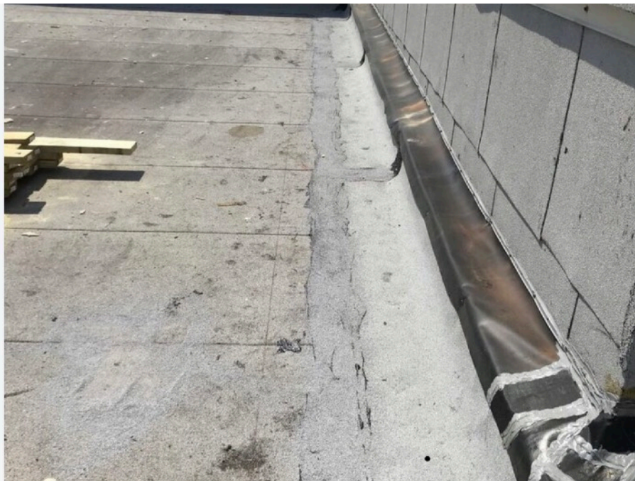
Overview of rubber seal over expansion joint.
