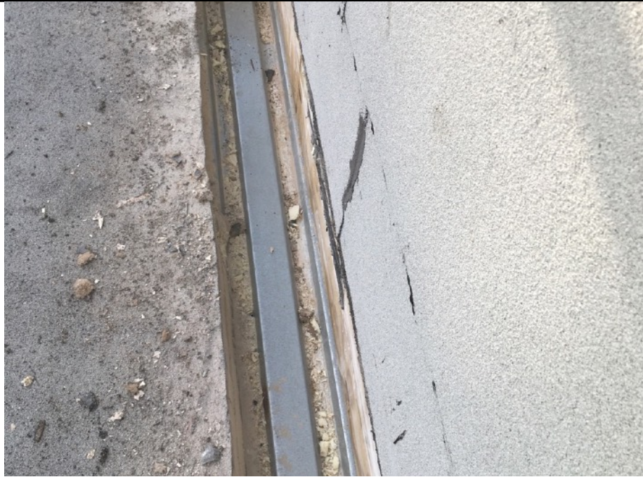
Existing roof cut out down to existing steel deck.
