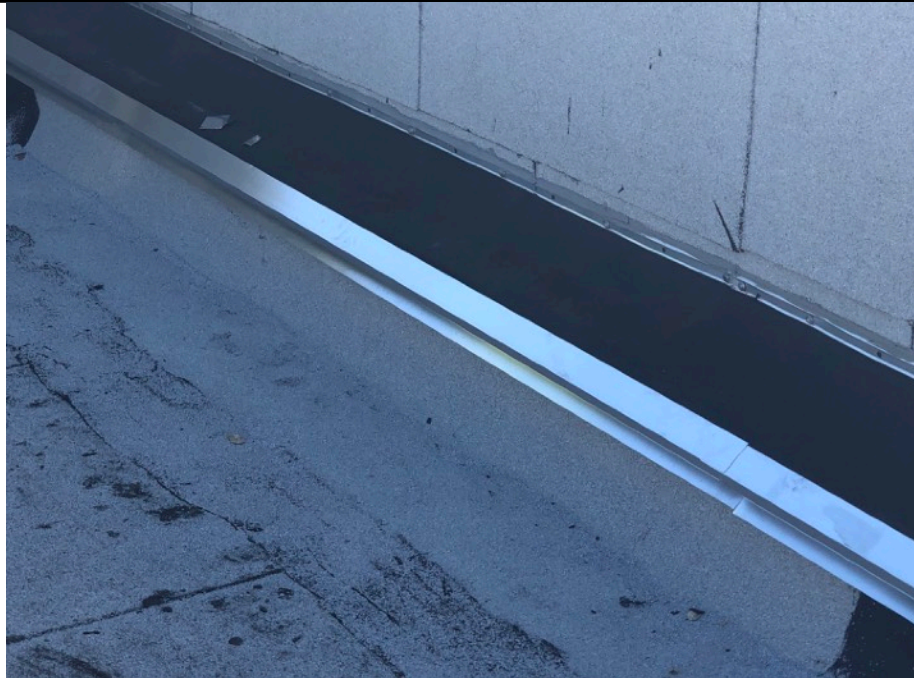
Sheet metal cleat installed 12" on center.
