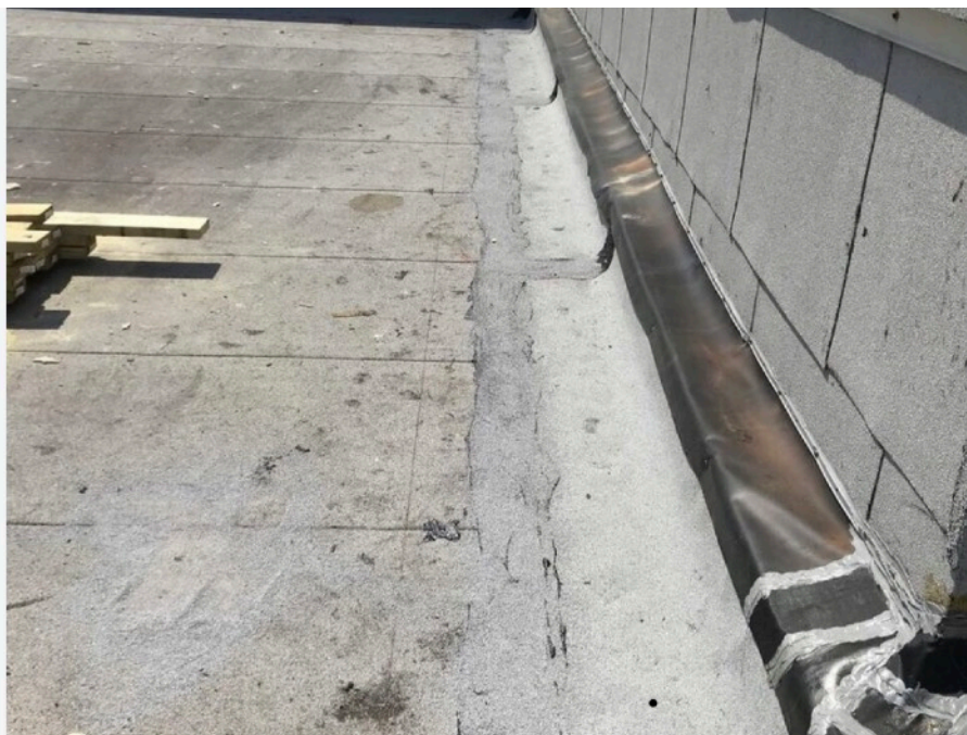
Overview of rubber seal over expansion joint.
