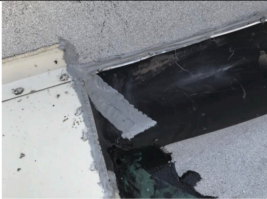
Caulk applied over termination bar at corner with 3 course mastic.
