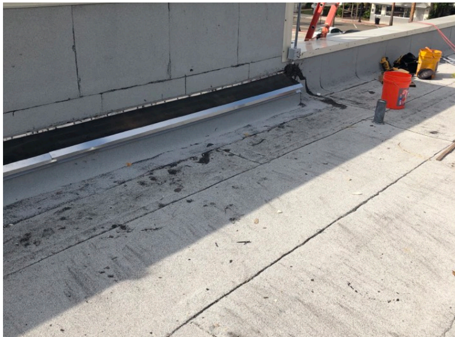
Overview of sheet metal cleat.
