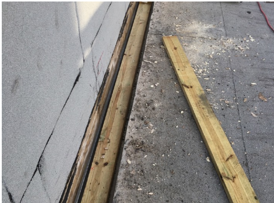
Wood nailer fastened to steel deck.
