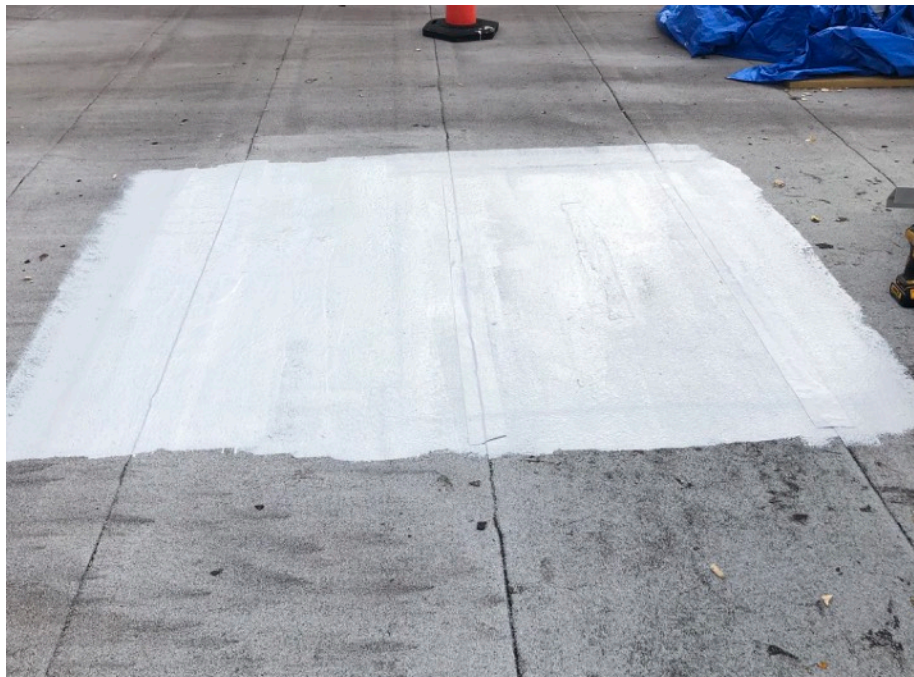
Application of Alphaguard BIO Base coat with reinforcement.
