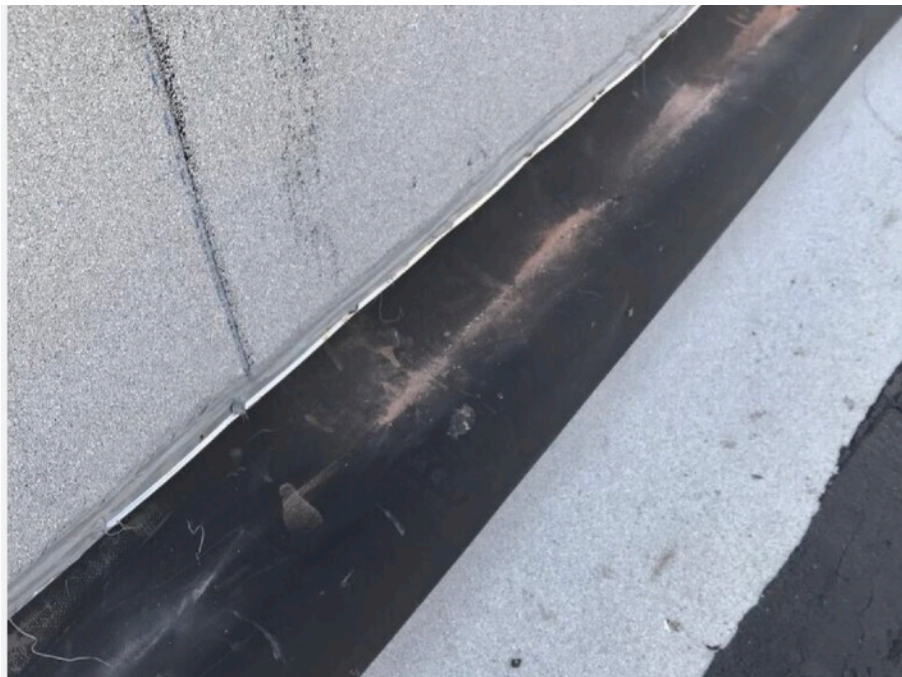
Termination bar fastened into masonry wall 6" on center.
