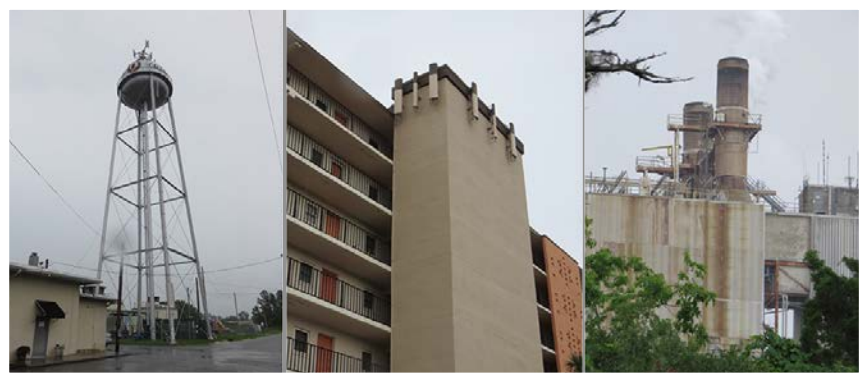
Figure 3: Water Tank, Rooftops Non-Concealed Base Stations
