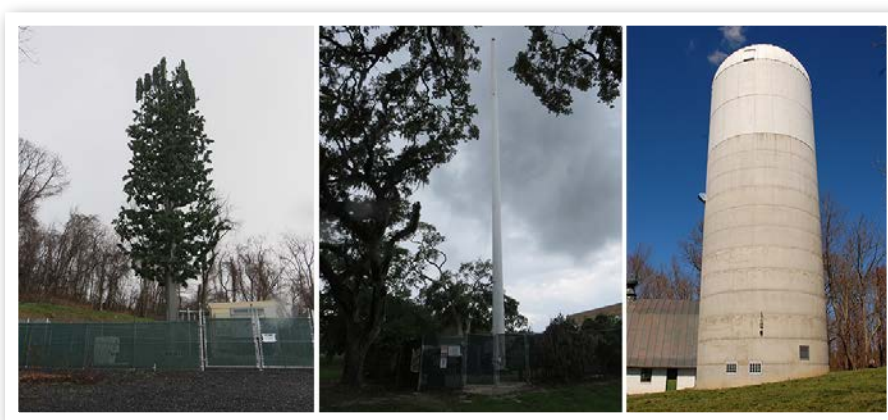
Figure 2: Faux Tree, Unipole, Faux Silo Concealed Towers
