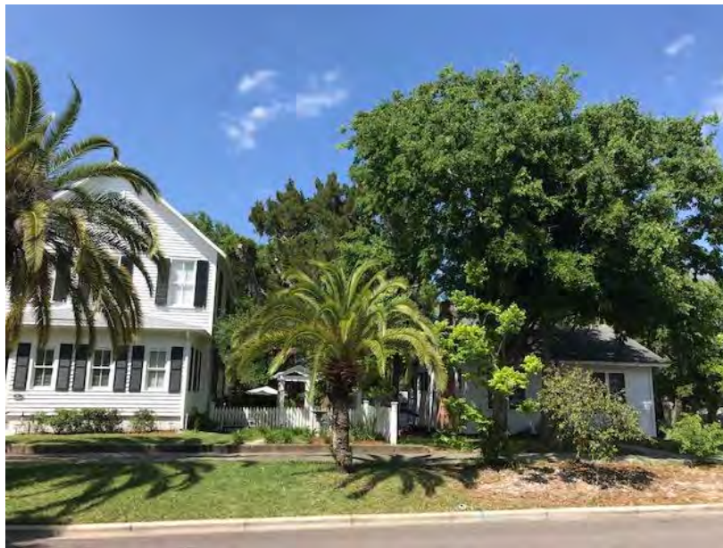
Photo 2: Broome Street looking North
