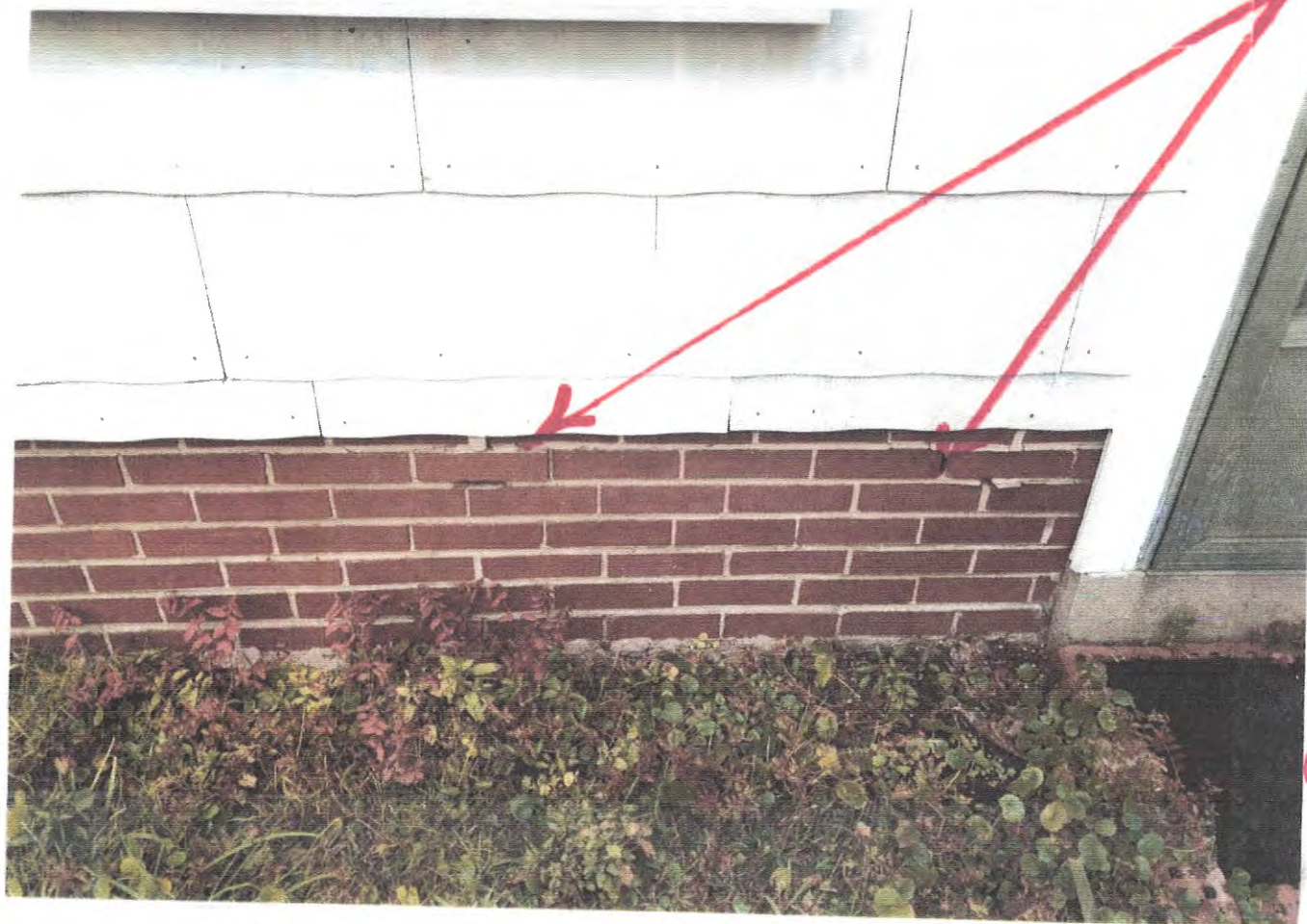
Cracked & Buckled Brick stem wall
