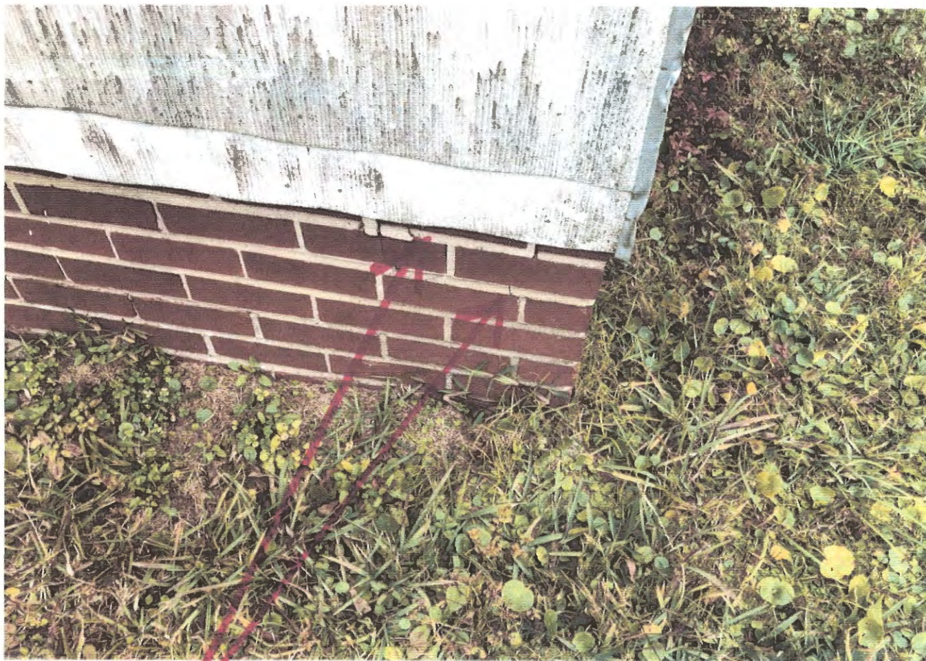
Cracked & Buckled Brick stem wall
