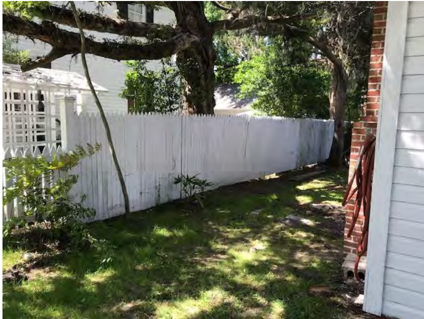
Photo 1: New 6' high P.T. Wood Privacy Fence to match adjacent fence
