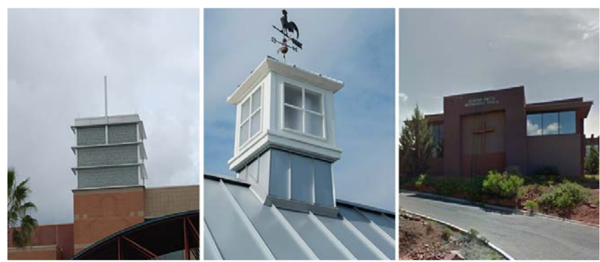
Figure 4: Faux Dormers Concealed Base Stations
