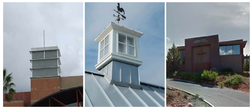
Figure 4: Faux Dormers Concealed Base Stations
