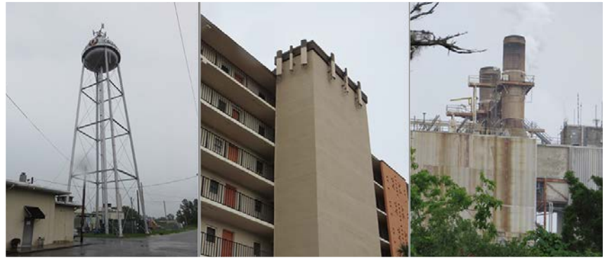
Figure 3: Water Tank, Rooftops Non-Concealed Base Stations
