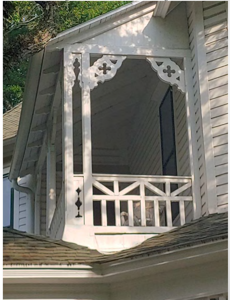
Detail Showing Side Porch Decorations. August 8, 2019
