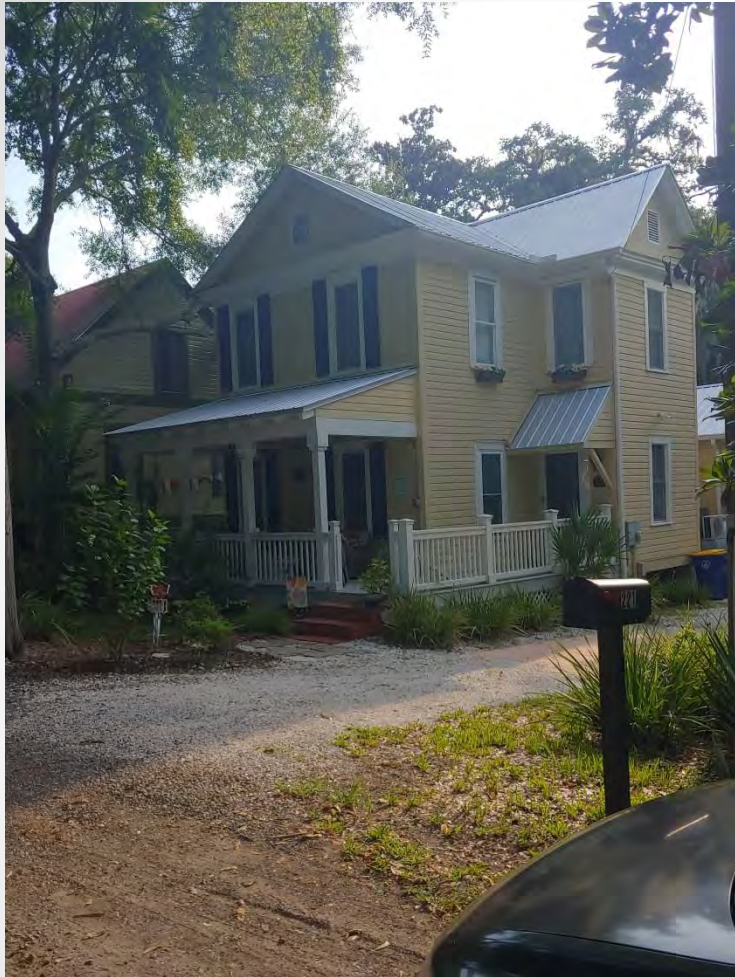
Side view of house showing uncovered section of porch. August 8, 2019
