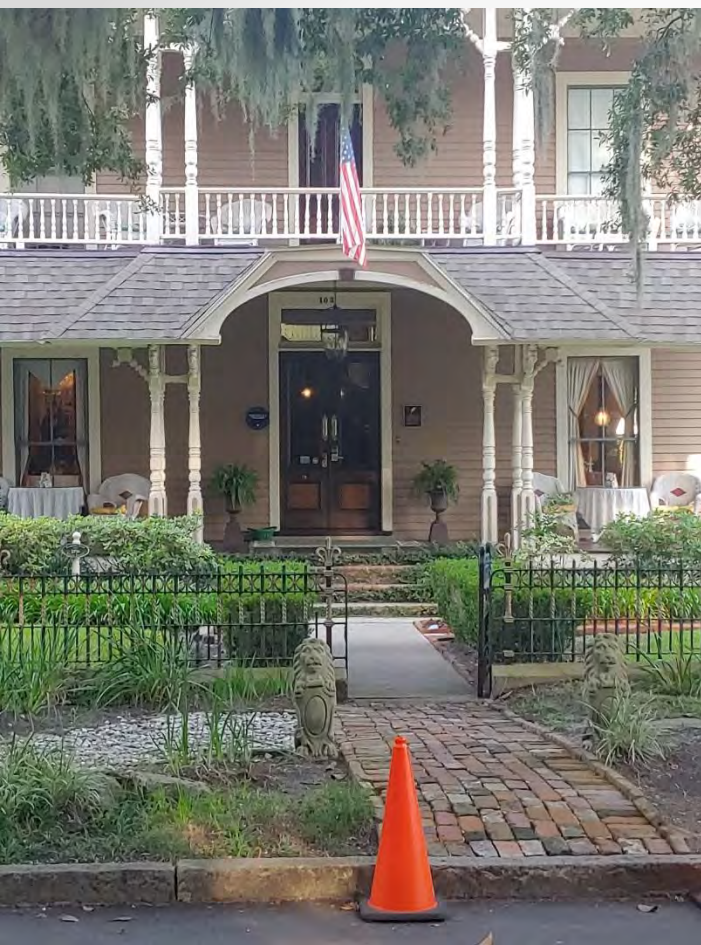
Detail showing entryway extension. August 8, 2019
