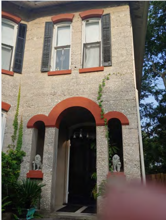
Detail showing arched entryway. August 8, 2019
