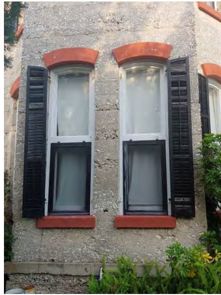
Detail showing arched decoration and shutters on windows. August 8, 2019
