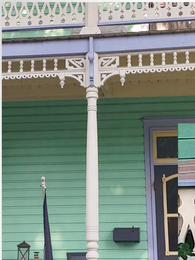
Detail showing porch decorations. August 8, 2019
