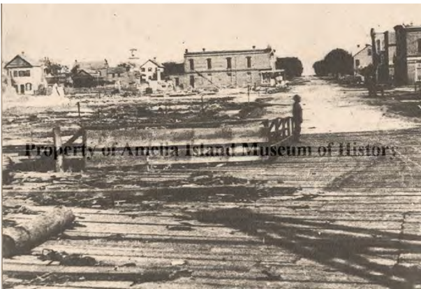
Center Street Fernandina looking west from the harbor right after the fire on March 23, 1876. The Kydd Building (center) is one of the few buildings that survived. AIMH ObjectID 2001.002.108
