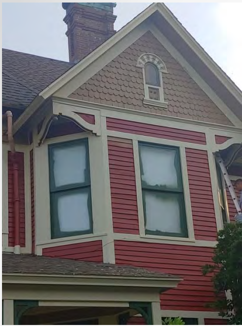
Detail showing side-facing gable and decorations on eaves. August 8, 2019
