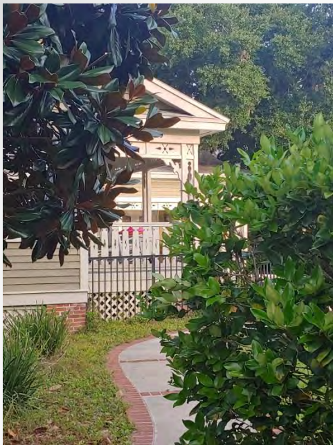
View of side porch. August 8, 2019
