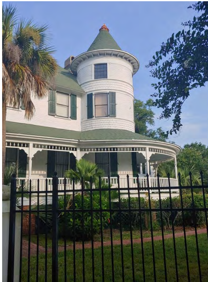
View of Tower and Wraparound Porch. August 8, 2019
