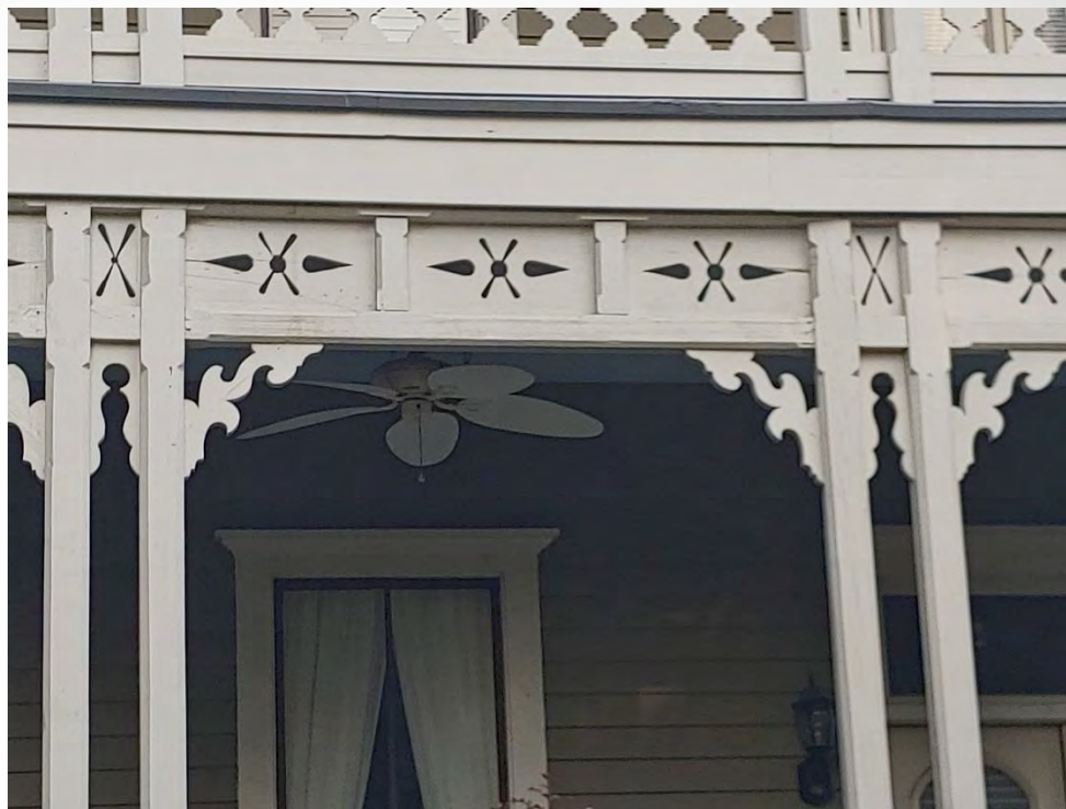
Detail showing frieze and decoration at top of porch supports. August 8, 2019
