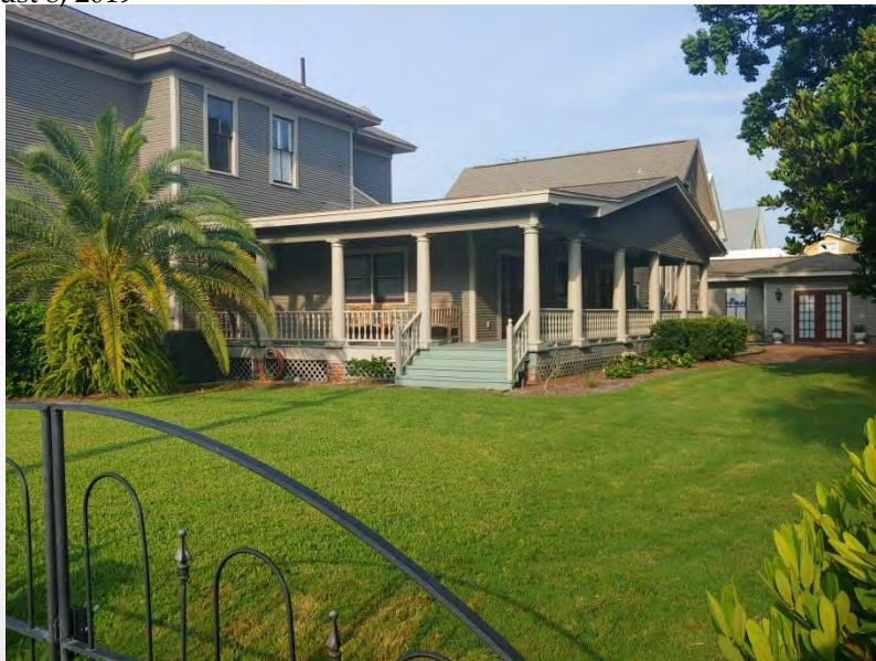
View of side porch. August 8, 2019
