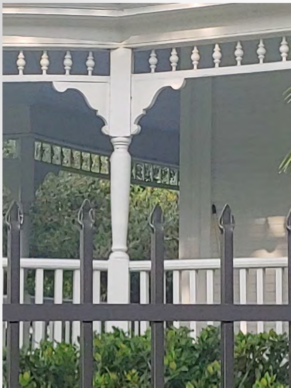
Detail Showing Porch Decorations. August 8, 2019
