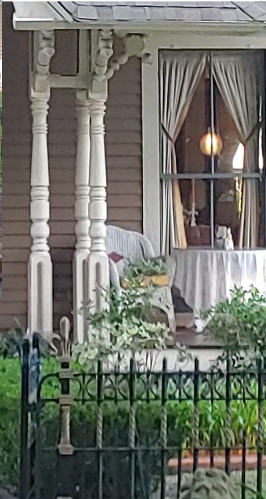
Detail showing porch supports and spandrels. August 8, 2019
