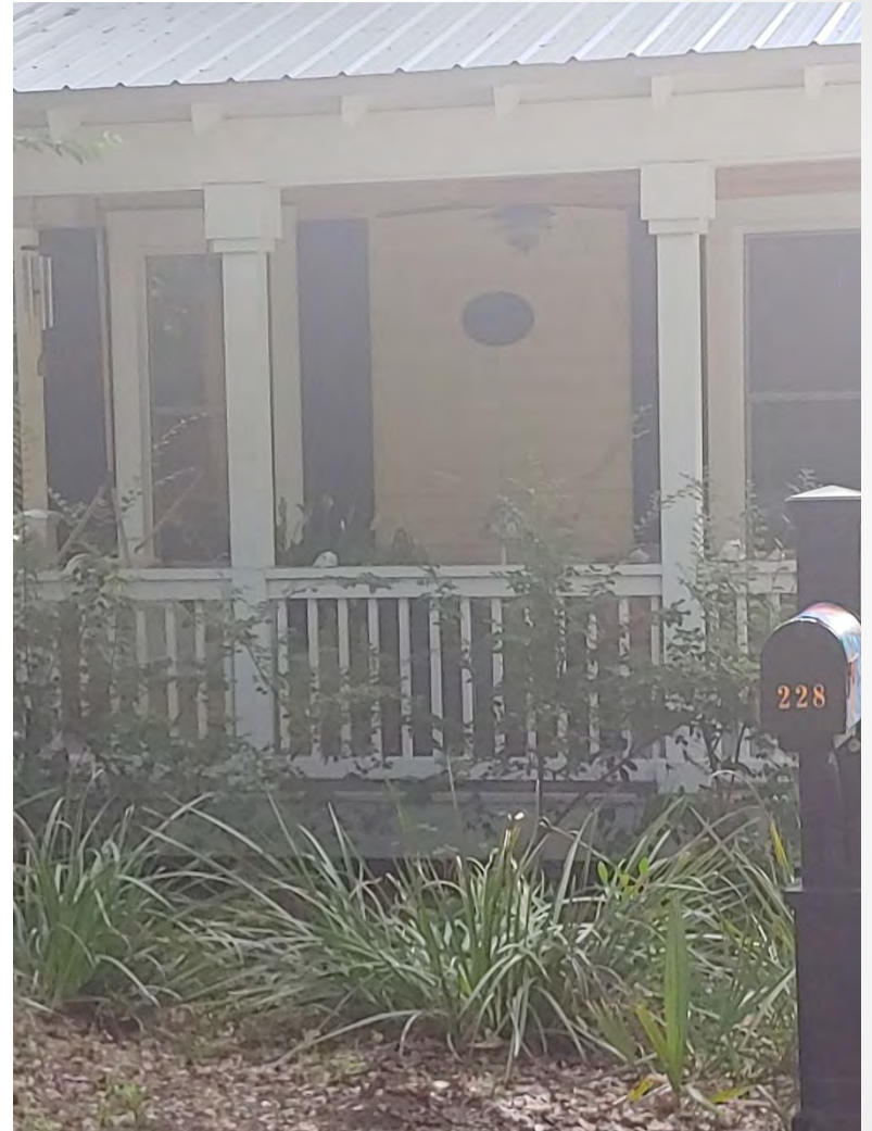
Detail showing porch supports and balusters. August 8, 2019
