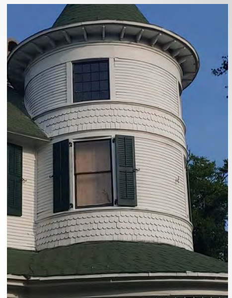
Detail Showing Tower Wall Decoration. August 8, 2019
