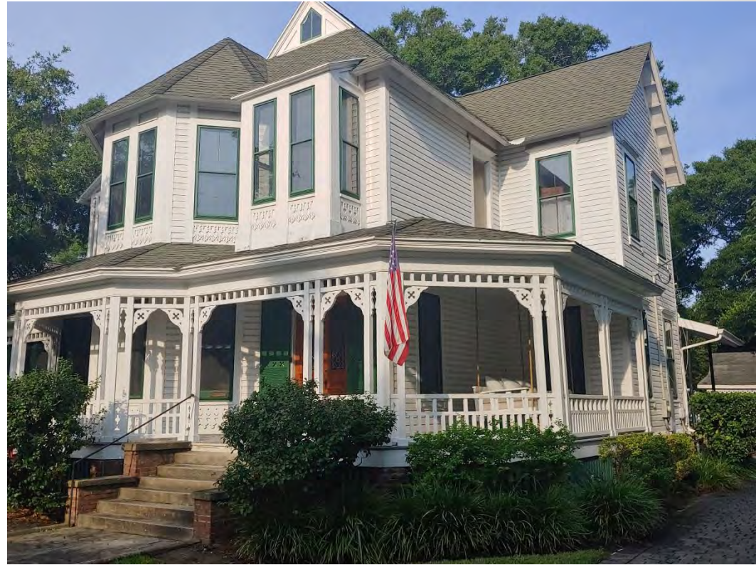
View of Front Porch and Projections. August 8, 2019
