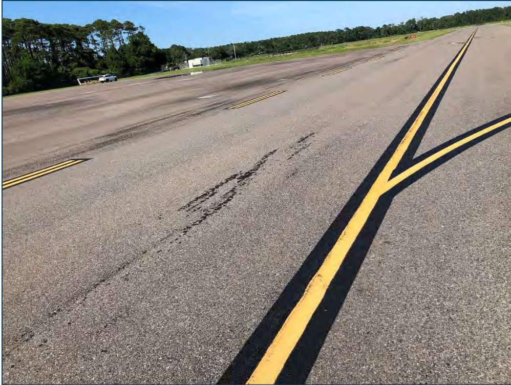
TW A, Section 325, Sample Unit 125 - (42) Bleeding Low Severity (57) Weathering
