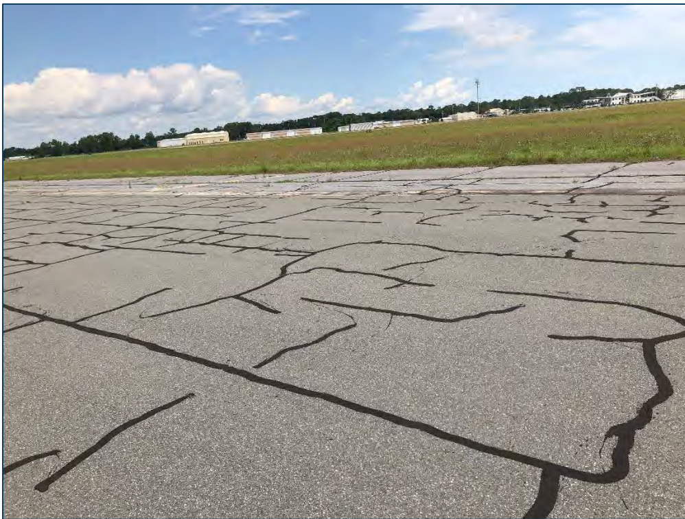
RW 13-31, Section 6215, Sample Unit 365 - Low Severity (43) Block Cracking, Low Severity (48) Longitudinal & Transverse Cracking, and Low Severity (57) Weathering
