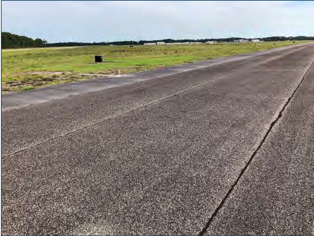
RW 4-22, Section 6105, Sample Unit 108 - Low Severity (48) Longitudinal & Transverse Cracking, Low Severity (52) Raveling, and Low Severity (57) Weathering
