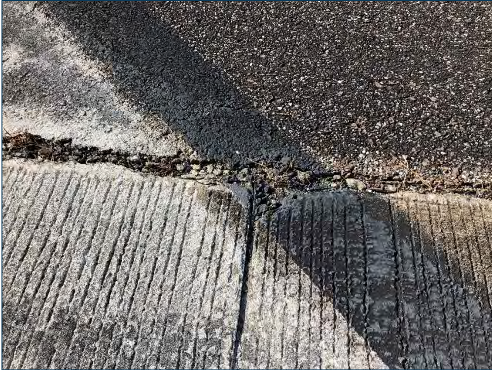
RW 9-27, Section 6305, Sample Unit 309 - Low Severity (65) Joint Seal Damage and Low Severity (75) Corner Spall
