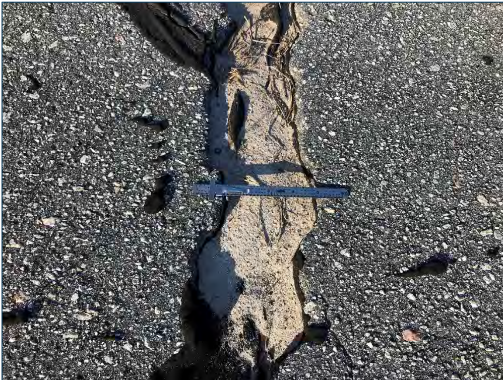
TW B, Section 230, Sample Unit 141 – High Severity (48) Longitudinal & Transverse Cracking, Low Severity (52) Raveling, and Low Severity (57) Weathering
