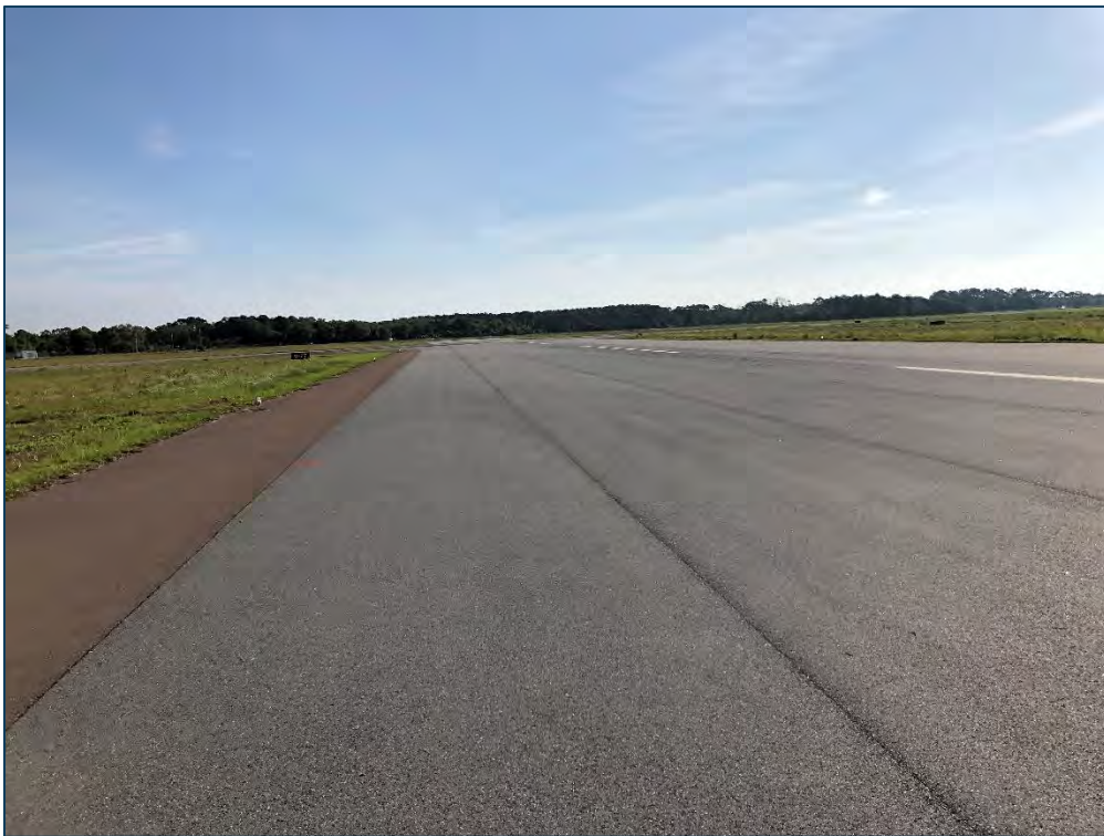
RW 4-22, Section 6110, Sample Unit 177 - Low Severity (48) Longitudinal & Transverse Cracking and Low Severity (57) Weathering
