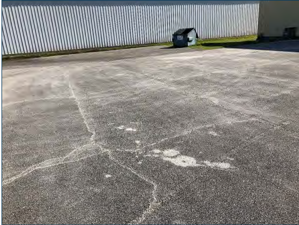
AP NW, Section 4110, Sample Unit 300 - Low Severity and Medium Severity (43) Block Cracking, Low Severity (52) Raveling, and Low Severity (57) Weathering
