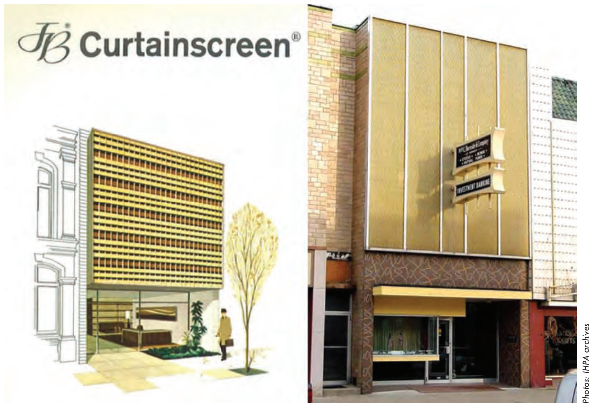
Figure 6: On the left is “The Art of Refacing the New Art in Architecture” Julius Blum & Co.’s JB Curtainscreen, 1965. On the right, Burnside and Co., in Danville, Illinois, is an excellent example of an unusually intact design with gold anodized aluminum slipcover, cantilevered display case, decoratively tiled storefront, and period signage and deserves preservation.
