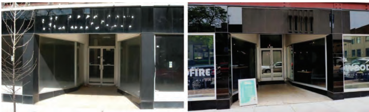
Figure 7: This black mid-twentieth century structural glass storefront was the third modernizing storefront for this mid-nineteenth century building in Rockford Illinois. The storefront was originally slated for demolition and replacement with an earlier neo-historic-style storefront. However, as part of the historic tax credit project the structural glass midcentury storefront was deemed a significant alteration and was retained, the sign damage was repaired and where necessary replaced by salvaged glass. The recessed terrazzo entrance lobby flooring was also retained. New signage was installed onto the storefront clear glass and did not damage the newly repaired structural glass transoms.
