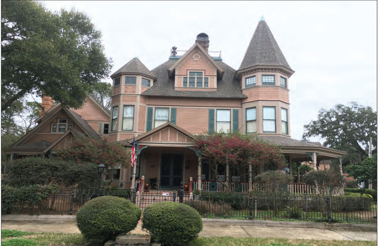
Figure 4.5 View of the Bailey House (NA00083), example of the Queen Anne style.
