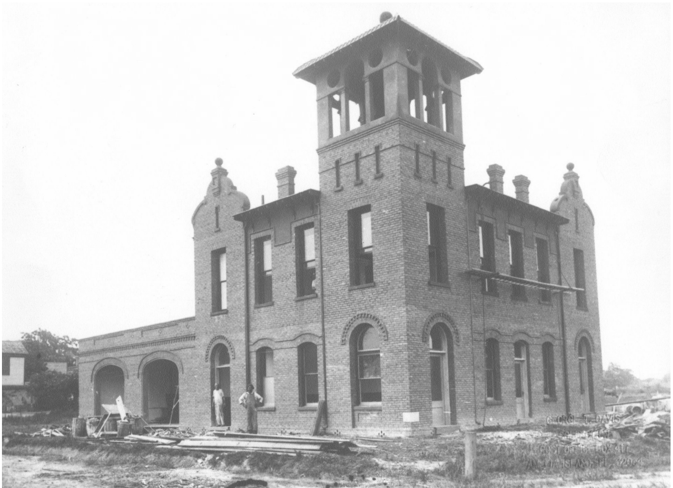
City Hall under construction. 1904
