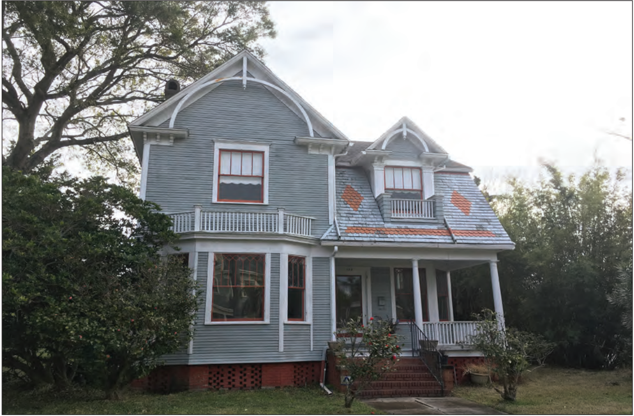
Figure 4.4 View of the Baker House (NA00100), example of the Stick style.
