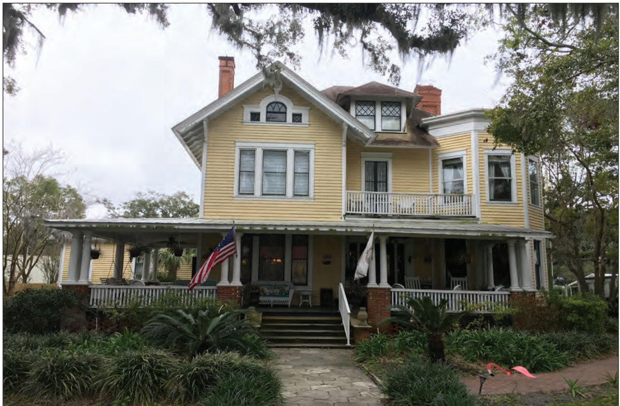
Figure 4.7 View of the Hoyt House (Resource NA00666), example of a Neoclassical style house.
