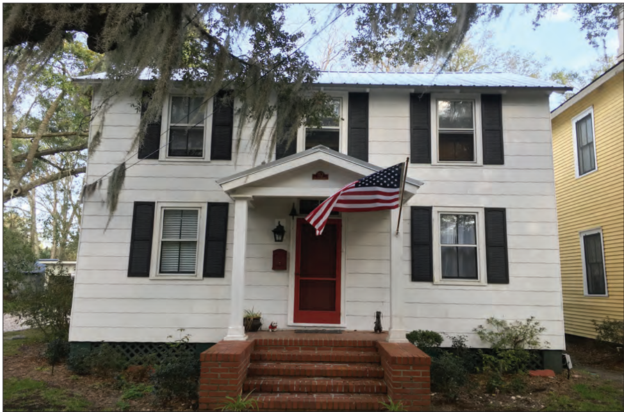
Figure 4.14 View of Resource NA00554, example of an I-house.
