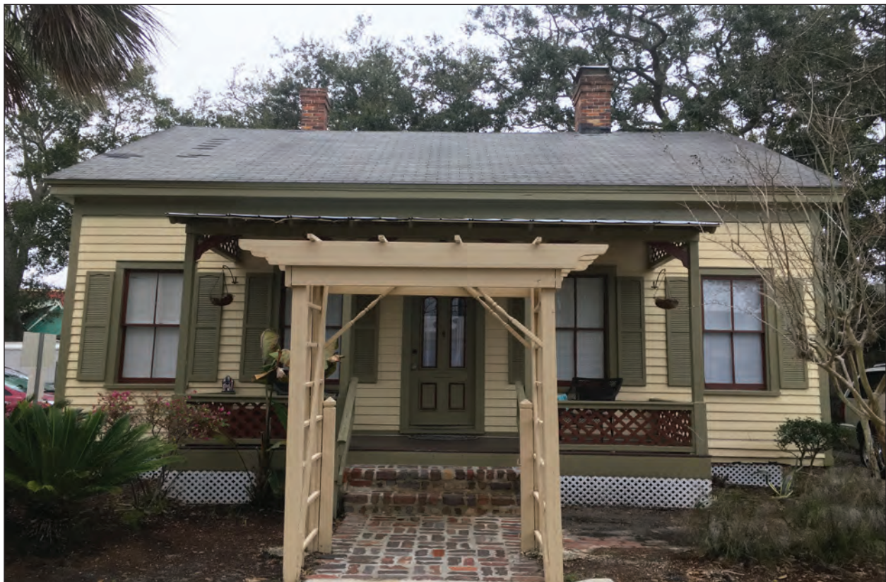
Figure 4.15 View of Resource NA00334, example of a hall-and-parlor house.
