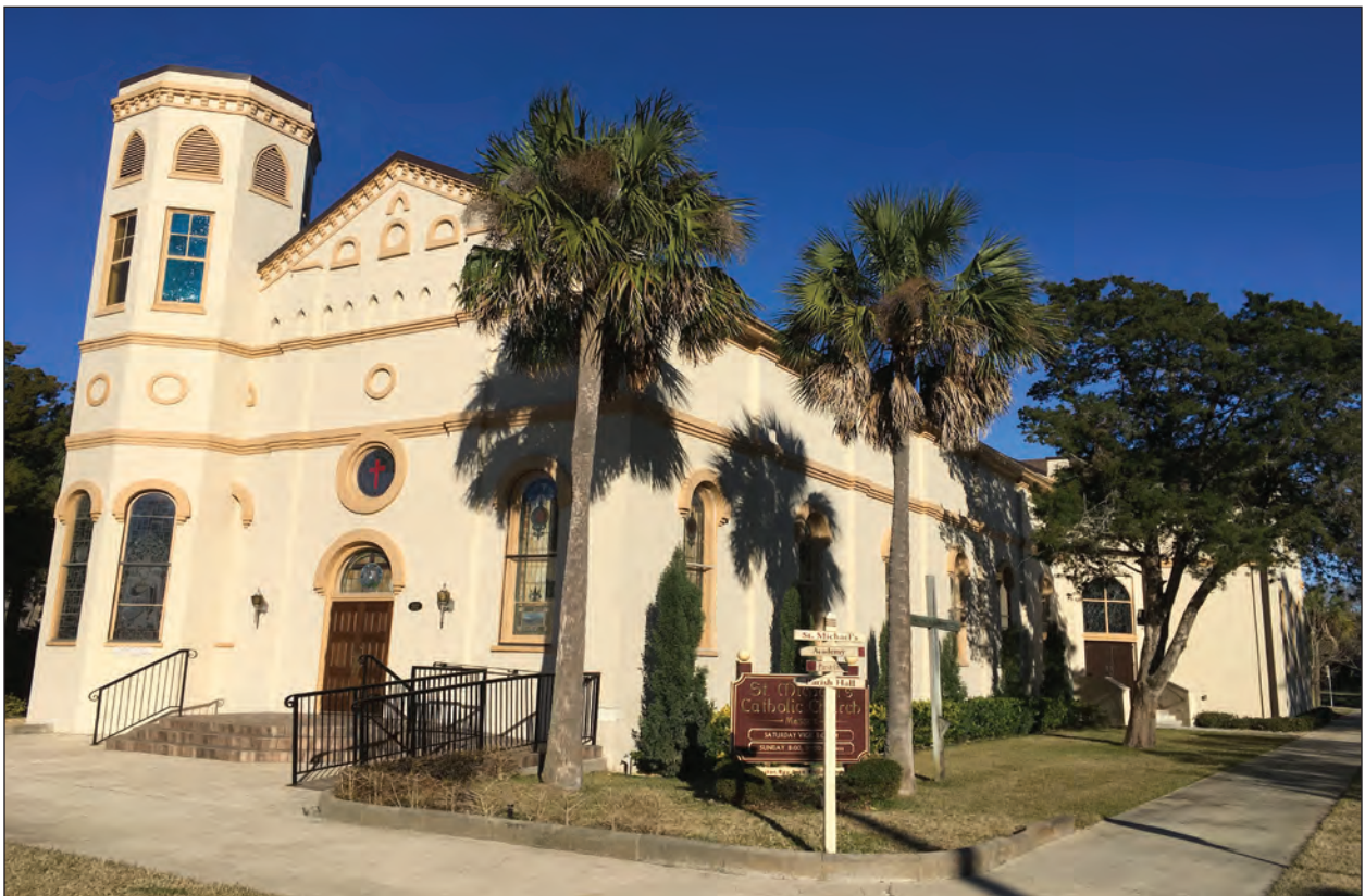
Figure 4.23 View of Resource NA00304, the Saint Michael's Catholic Church, example of Richardsonian Romanesque style.
