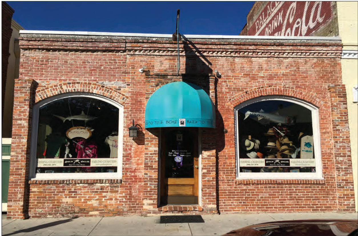
Figure 5.2 View of Resource NA01115, a building that has regained its historic integrity by removing inappropriate building materials.
