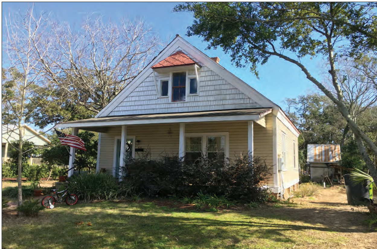
Figure 4.11 View of Resource NA00271, example of a front-gable house.
