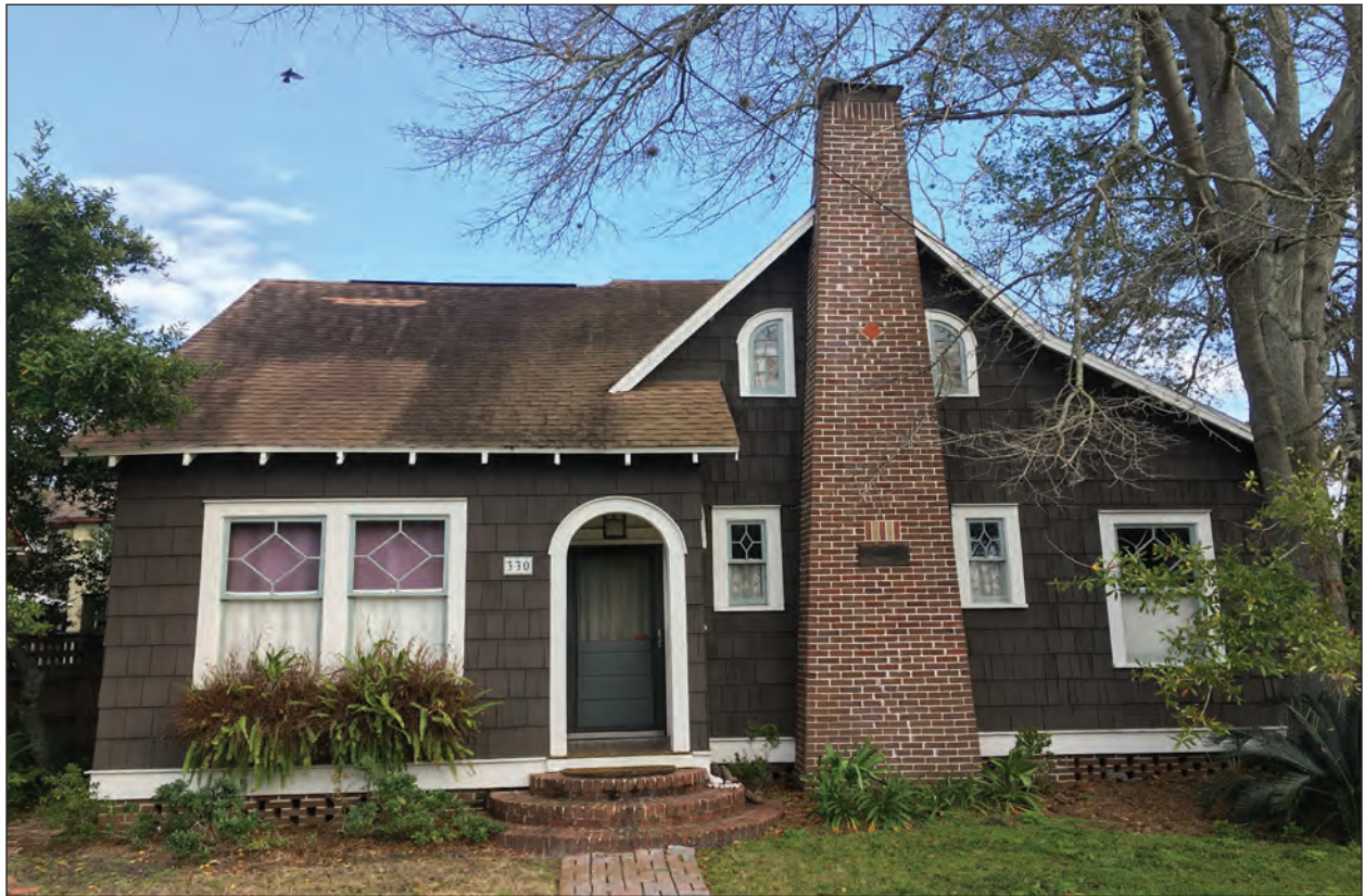
Figure 4.8 View of Resource NA00474, example of a Tudor style house.
