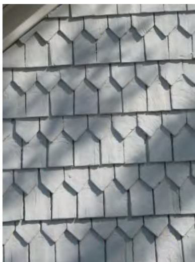
Original wood shingles at 801 San Fernando Street.
