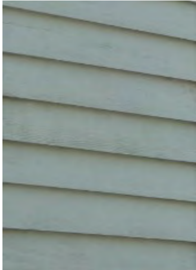
Original wood siding at 808 San Fernando Street.
