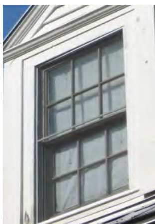
Below: The window screens are difficult to see, allowing for full view of the original six-over-six wood sash window (902 Ladies Street).
