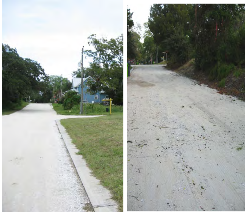
Views of shell street surfaces in 2012.
