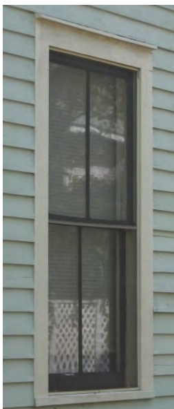
Above: Original two-over-two wood sash window (808 San Fernando Street).
