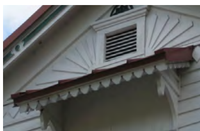
Preserve functional and decorative awnings (212 Estrada Street).
