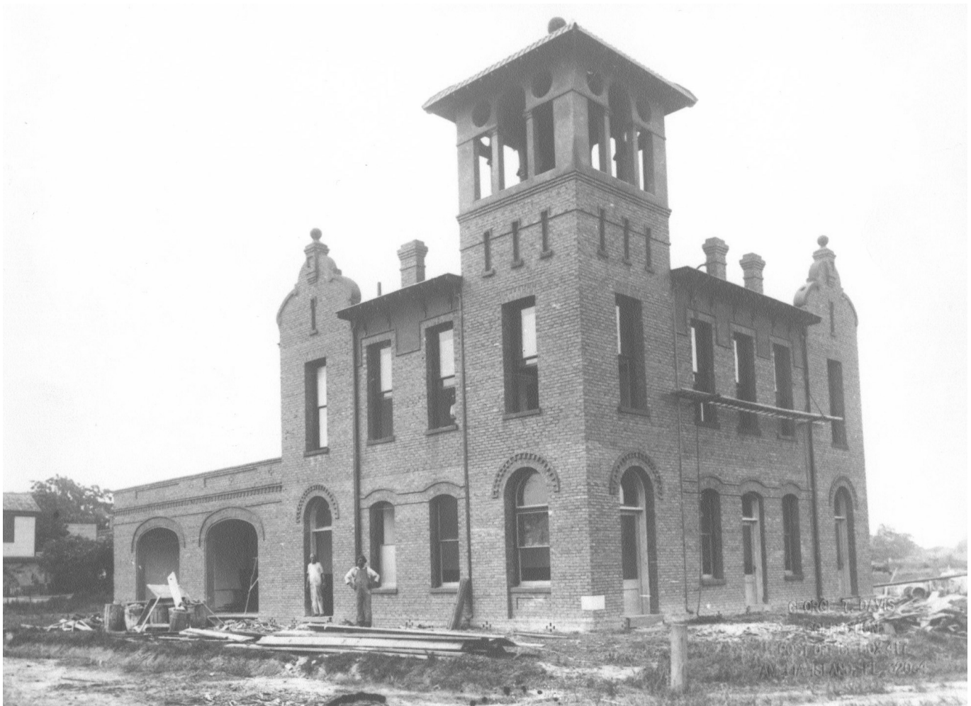
City Hall under construction. 1904
