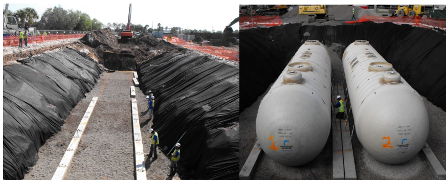
OIA QTA UST and associated Fueling piping installation
