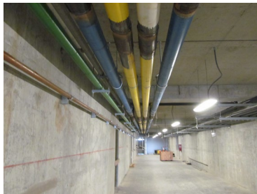
Double walled welded fuel piping installed
