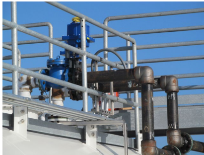
Double walled welded fuel piping installed
