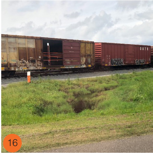
OUTFALL FROM STORM WATER CULVERT
