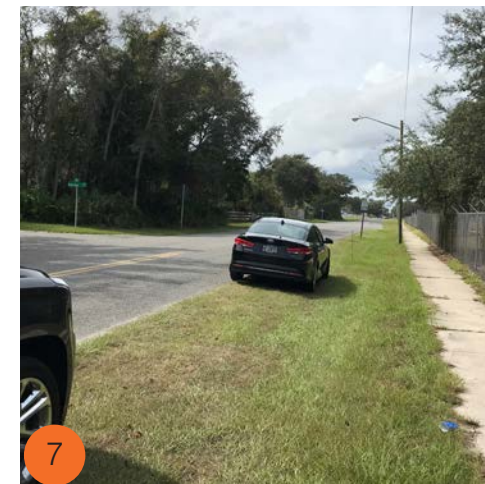
EXISTING WALK ON NORTH SIDE OF HICKORY ST.
