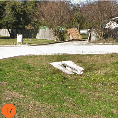
CULVERT UNDER LEGION DRIVEWAY THAT WILL NEED TO BE RELOCATED
