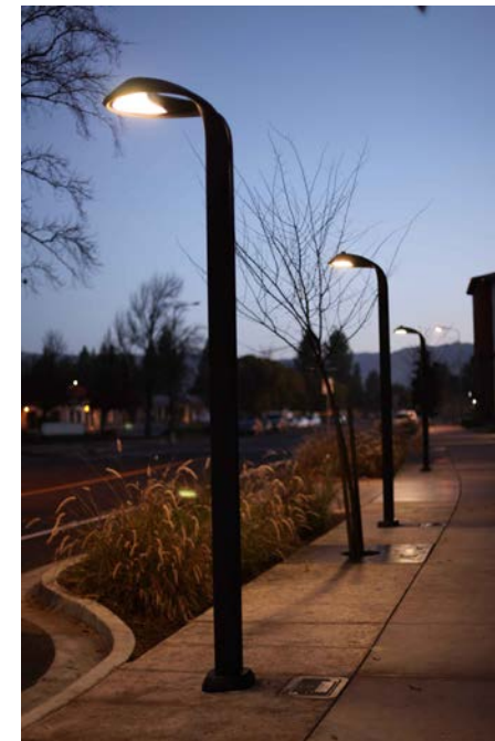
HI-GLO PEDESTRIAN LIGHTING
