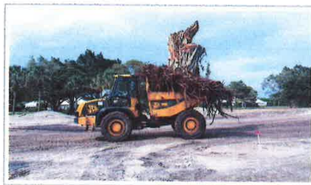
TREE REMOVAL AND STORM REPAIR
