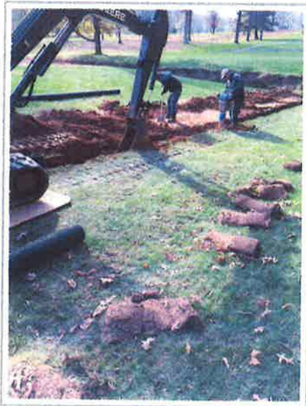
DRAINAGE FROM 2" ADS TO 60" RCP PIPE
