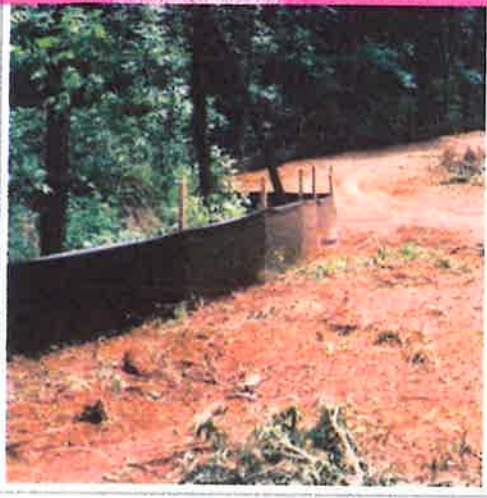
EROSION CONTROL IMPLEMENTATION
