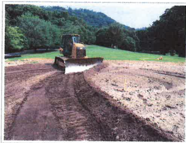
GRADING/SHAPING AND DETAILED FINISH WORK
