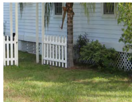
The new dwelling at 807 White Street was designed with a pier foundation infilled with lattice panels.
