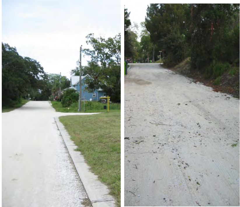
Views of shell street surfaces in 2012.
