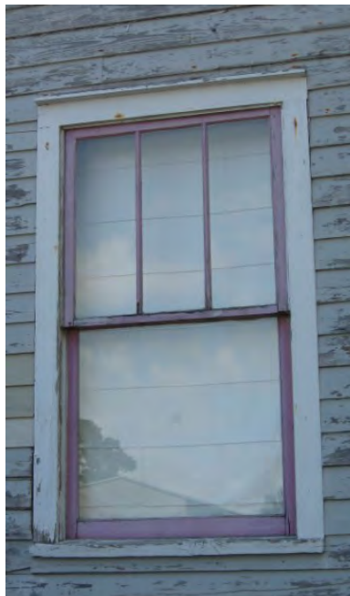
Left: Repainting the house and window trim in contrasting colors will help protect the wooden elements and accentuate the original three-over-one wood sash windows.
