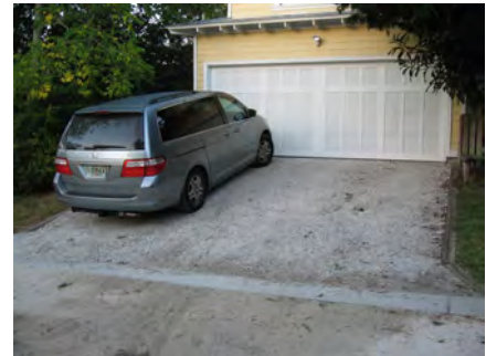
New driveways in the district should be of crushed shell or gravel such as 820 Someruelos Street.
