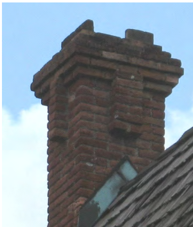
Original corbelled brick chimneys should be maintained and repaired as needed (910 San Fernando Street).
