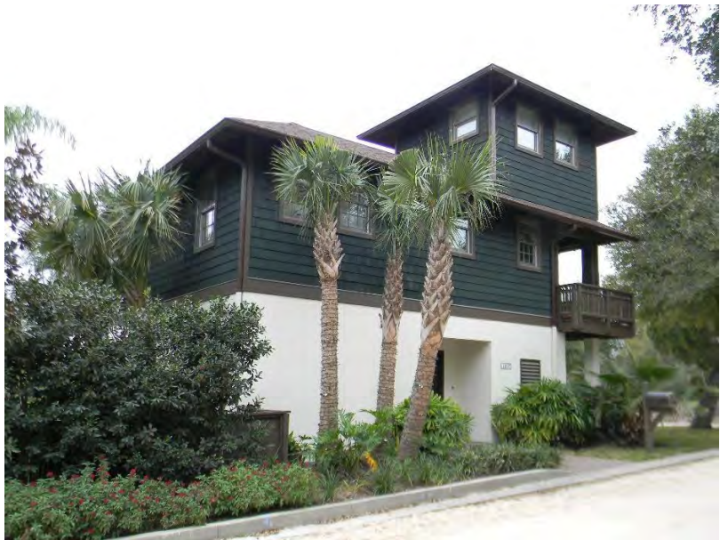
This dwelling at 1010 Someruelos was designed with a stucco and wood exterior, hipped roof and porches on the main façade. Its overall design is compatible with the historic architecture in the district.
