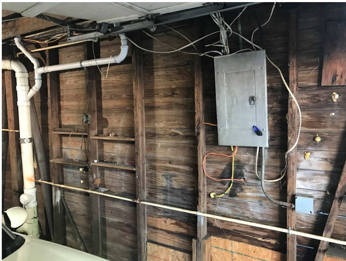
Garage framing – interior showing replacement of rot and reinforcement of framing.
