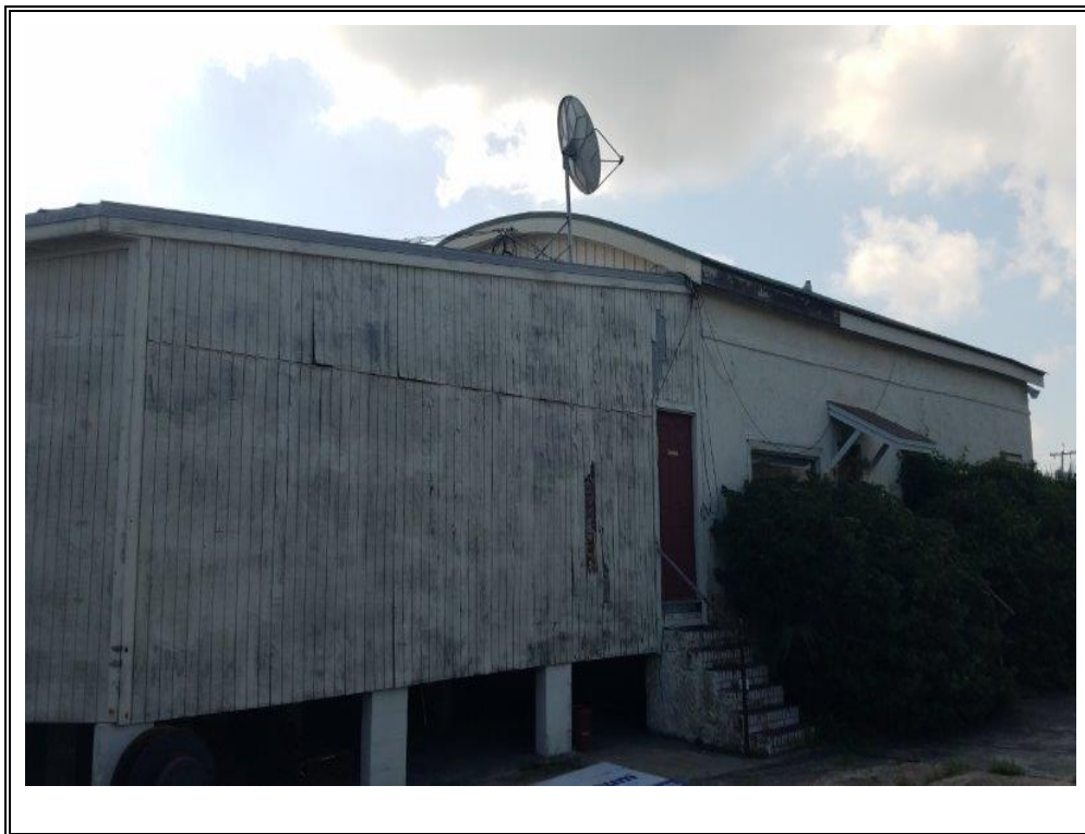
PHOTO 2: Side View: Entry to Office Area.
