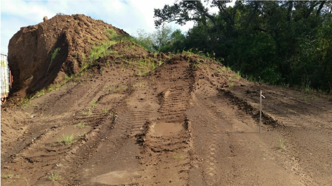
4 - Westrock CRAS backfill pile.
