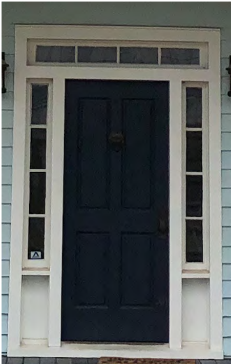
Exterior Doors Existing Wooden Front Door Remains (Painted Pure White)
