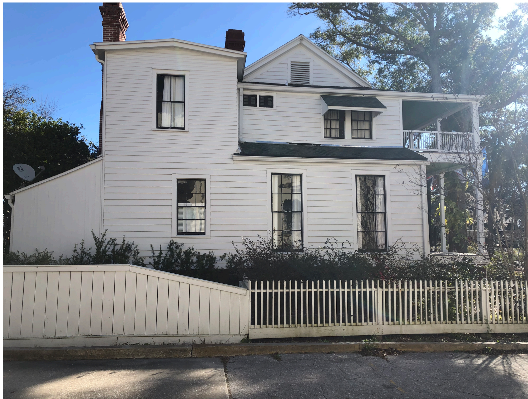
WESTERN ELEVATION – PRIMARY STRUCTURE
