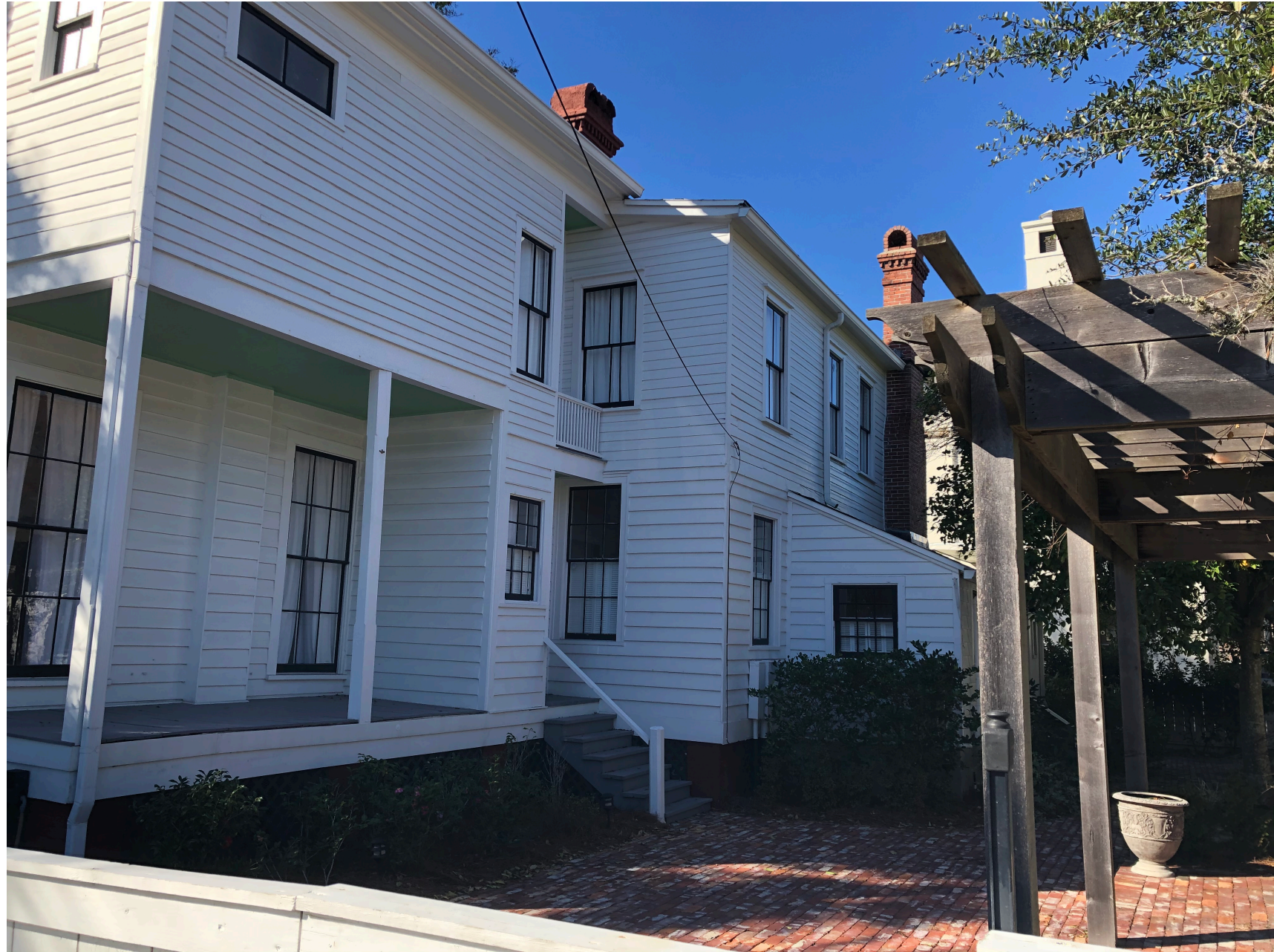
NORTHERN ELEVATION – PRIMARY STRUCTURE
