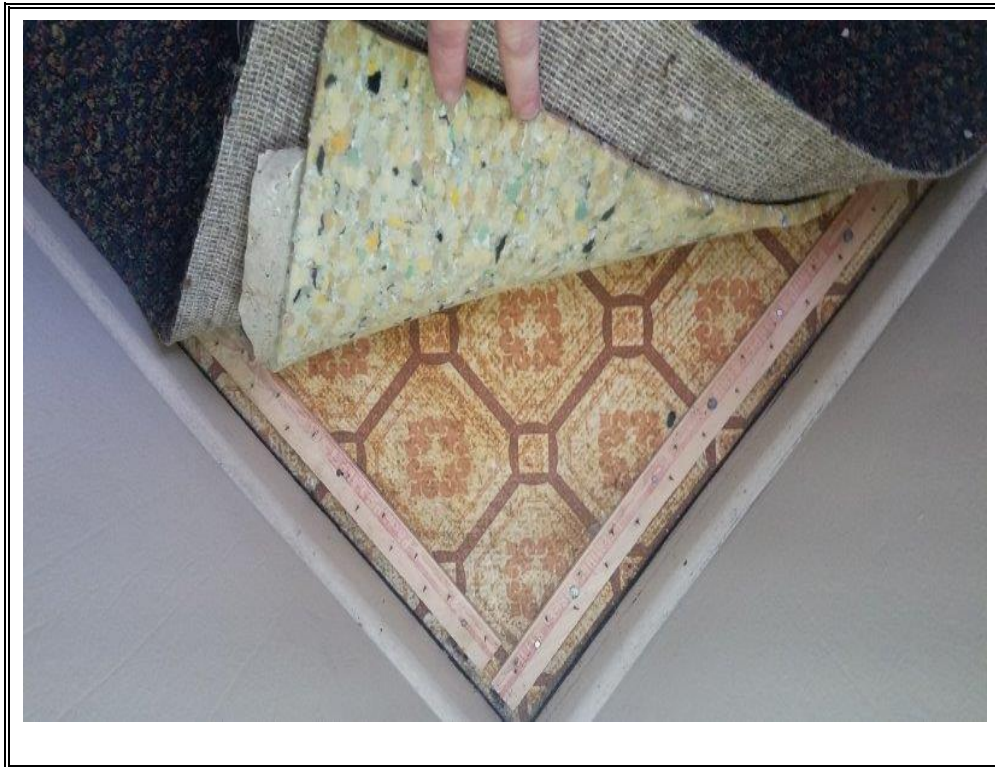
PHOTO 16: Sample 17: Brown Vinyl Sheet Flooring under Carpet.
