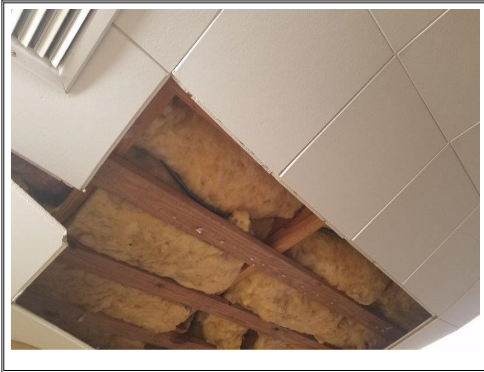
PHOTO 5: Samples 1 & 2: 1' x1' Ceiling Tiles" Smooth.
