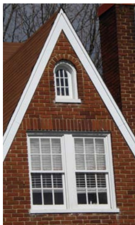
Paired Six Over Six Double-Hung Windows Under a Small Accent Window
