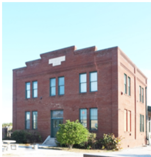
Warehouse Arts District
