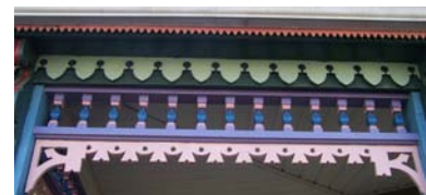
Gingerbread between Turned Posts on Spindlework Subtype
