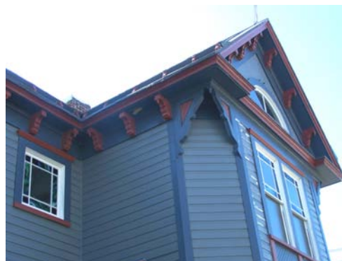
Brackets and Spandrels on a Spindlework Subtype
