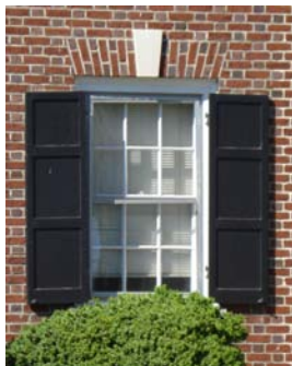
Six-Over-Six Double-Hung Window with Jack Arch and Operable Shutters
