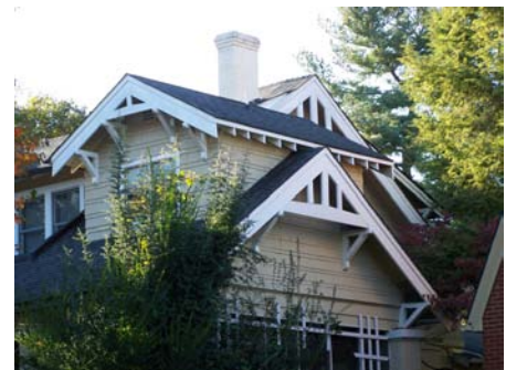
Exposed Rafter Tails and Triangular Knee Braces
