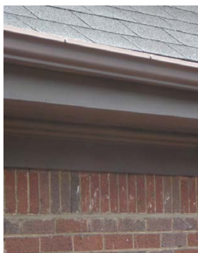
Soldier Course at the Roof Wall Junction of the Eave
