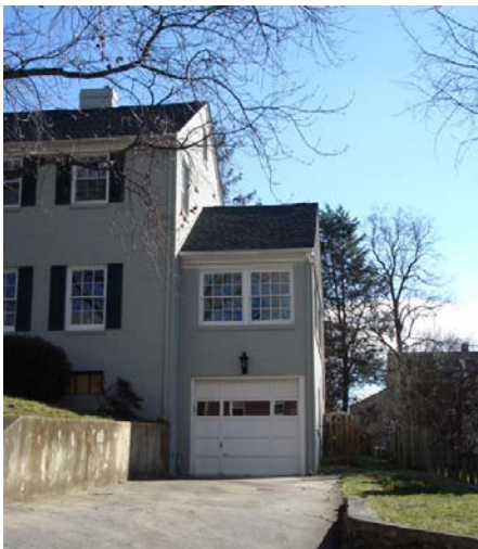
Attached Garage Below Main Level
