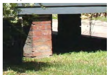
Brick foundation piers
