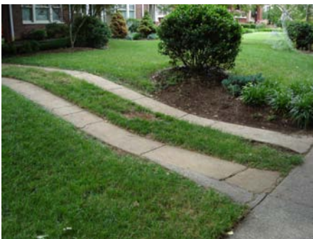
Concrete Parking Strips
