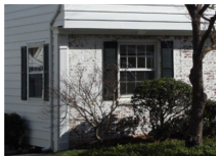
Combination of Brick and Siding with Corner Pilasters
