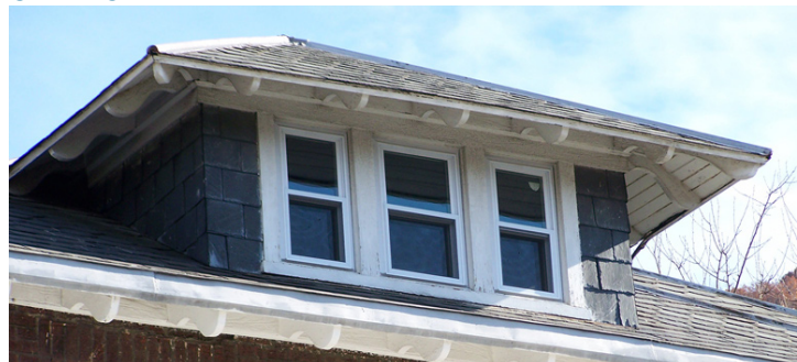
Hipped Dormer with Exposed Rafters
