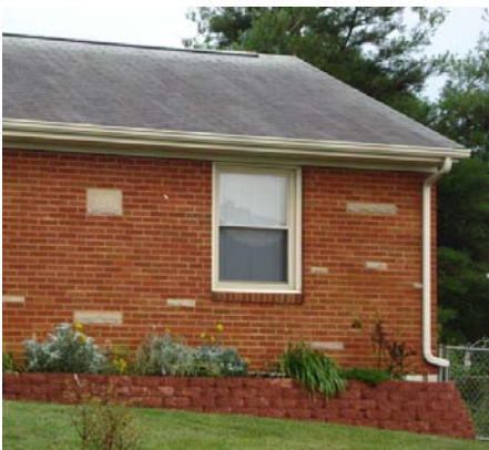
Brick Wall Cladding in Common Bond with Decorative Cast Stone
