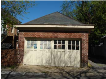
Two Bay Garage with Sliding Doors
