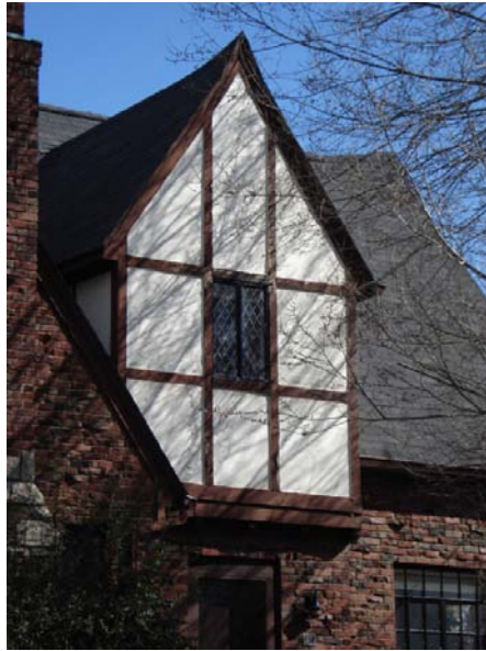
Light Stucco Offset by Dark Timbers
