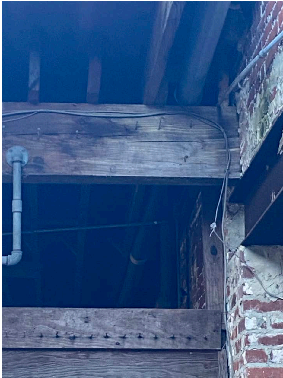
Main Structural Beam at Transition
