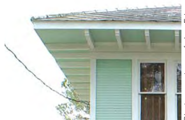
Boxed eave with shaped outriggers in hipped-roof condition
