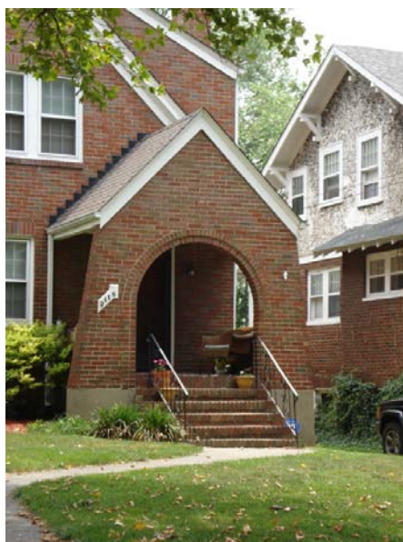
Portico with Wrought Iron Railing
