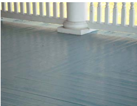
Porch Floor in Good Repair
