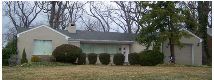
Front Loaded Attached Garage with Panel Door
