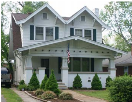
Intersecting Front Gables
