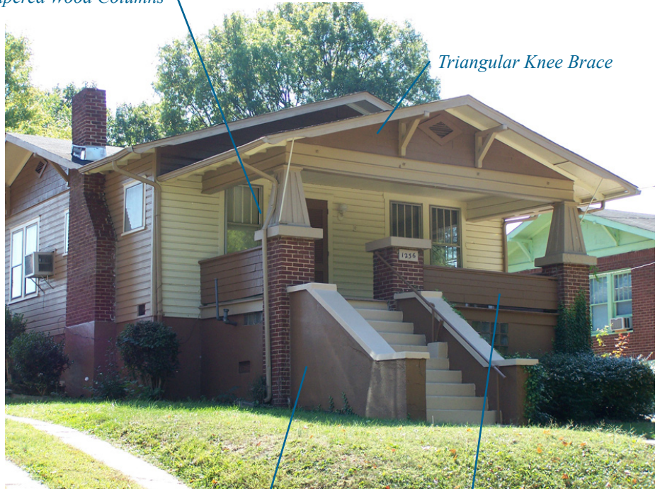
Steps with Flanking Concrete Walls
