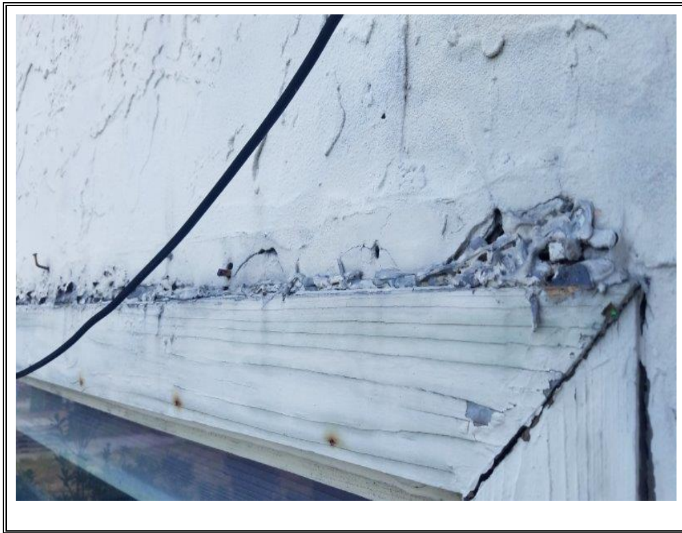
PHOTO 20: Sample 120: Exterior Window Frame Sealant.
