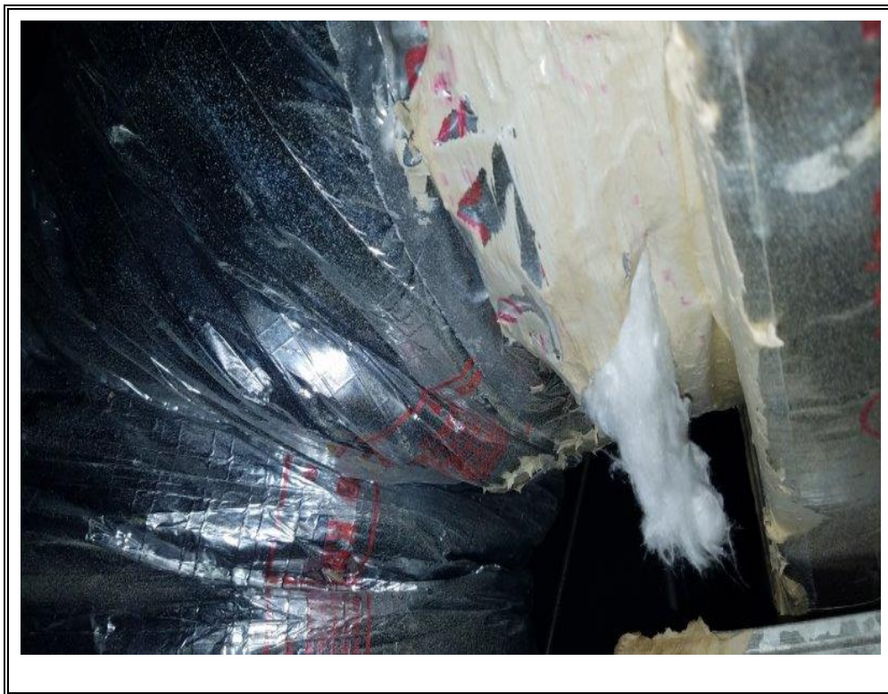
PHOTO 14: Samples 14 & 15: Attic HVAC Duct Cream Seam Sealant.
