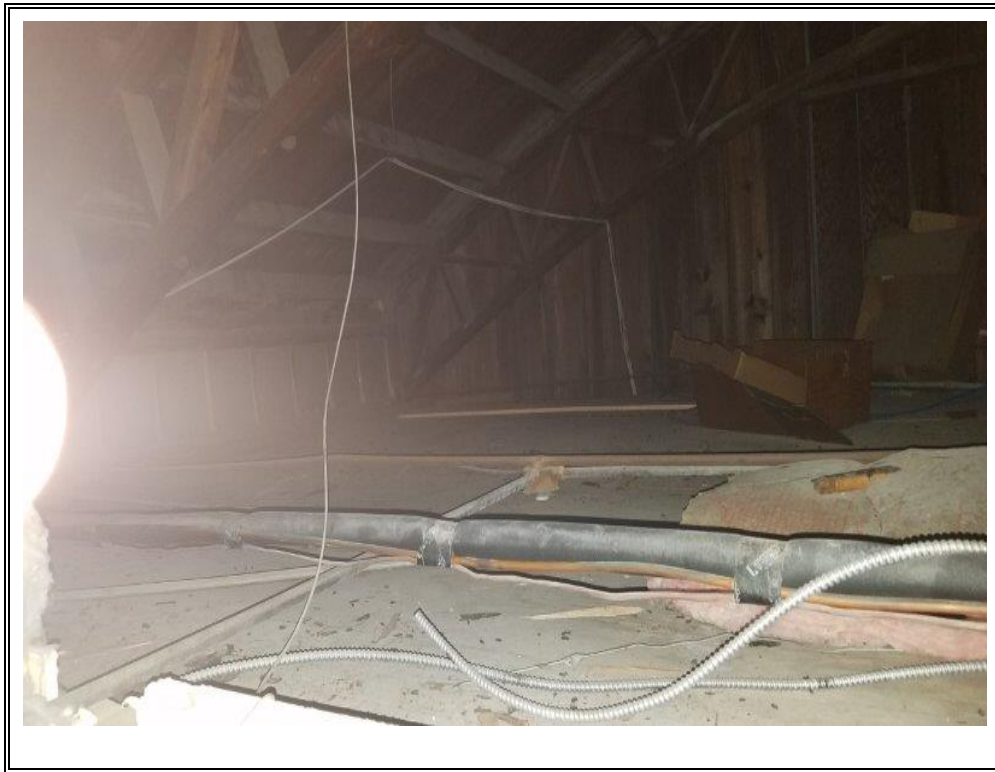
PHOTO 13: Office Area Attic View.
