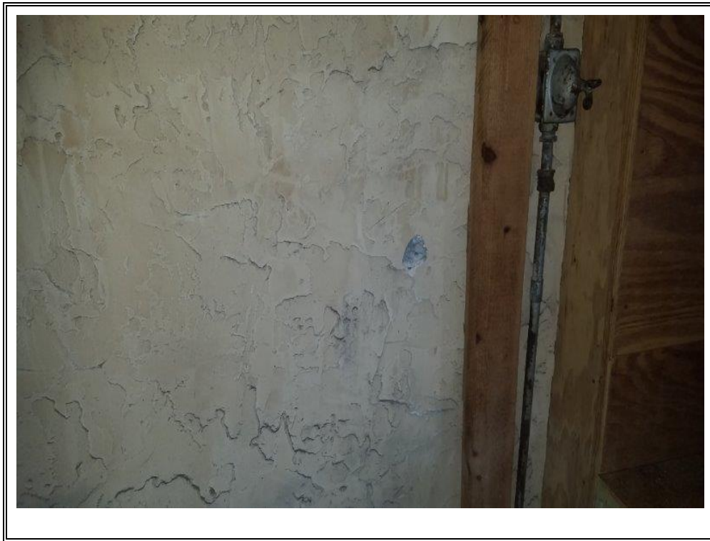
PHOTO 18: Sample 18: Wall Stucco in Warehouse.
