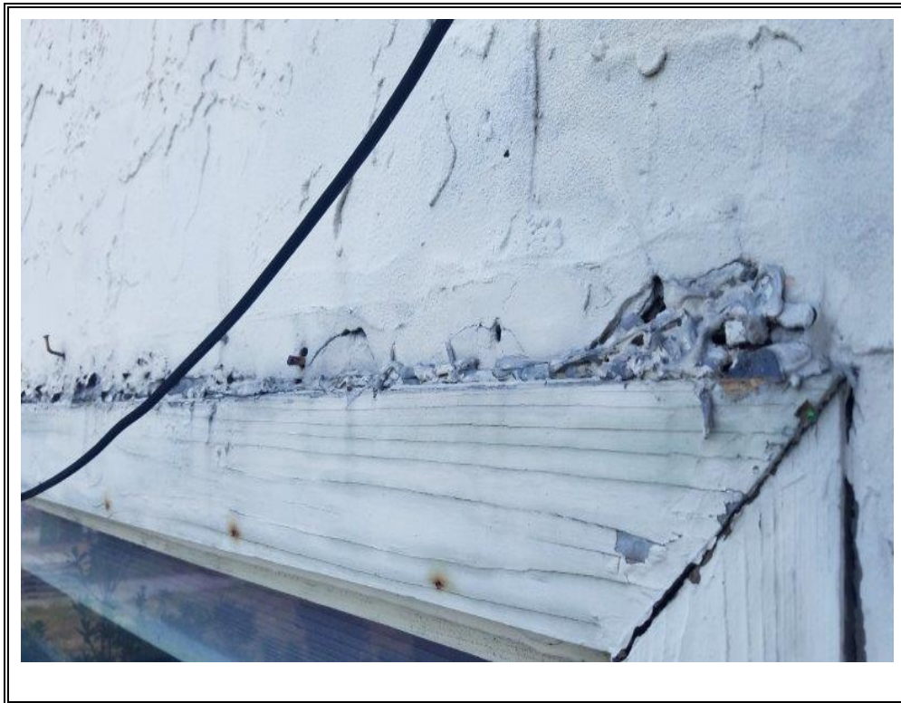
PHOTO 20: Sample 120: Exterior Window Frame Sealant.
