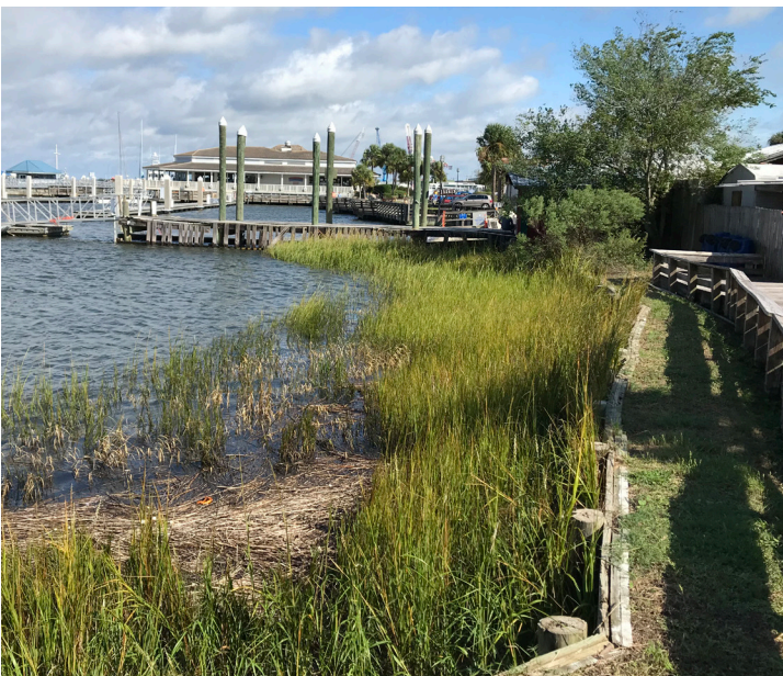
*Below image of existing timber bulkhead
