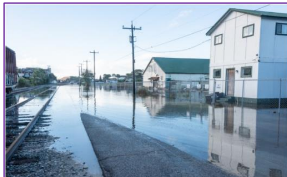
Figure 3: Photograph showing the effects of sunny-day flooding on the Downtown Waterfront Project Area. Tidally influenced flooding is an example of a chronic “stressor” on upland assets. Photo source: City of Fernandina Beach - Downtown waterfront Flooding Assessment (Desilet, 2019) 2
