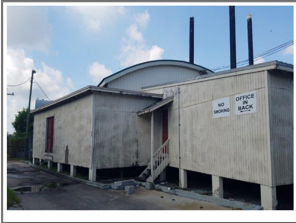
PHOTO 1: Front View: Warehouse side of Structure
