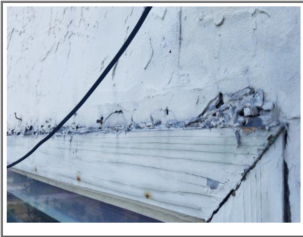
PHOTO 20: Sample 120: Exterior Window Frame Sealant.
