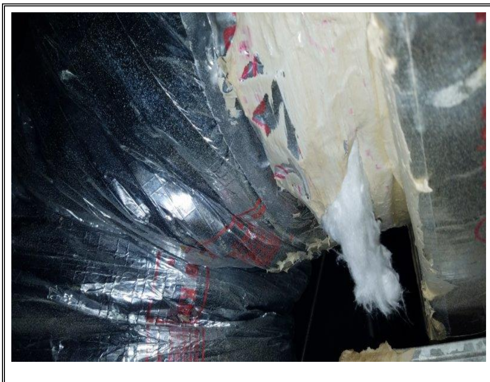
PHOTO 14: Samples 14 & 15: Attic HVAC Duct Cream Seam Sealant.
