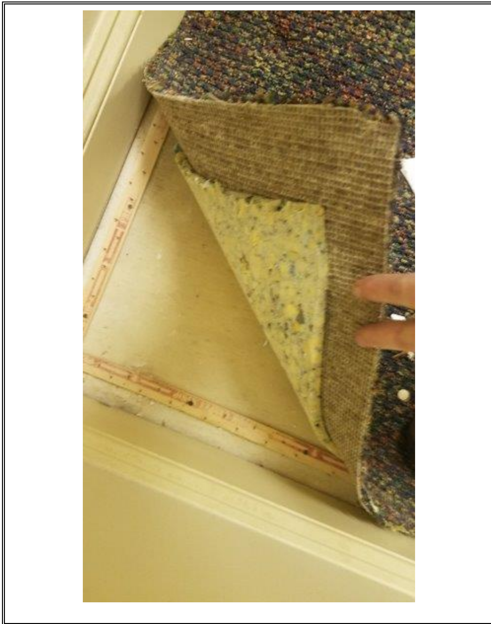
PHOTO 15: Sample 16: Tan Vinyl Sheet Flooring under Carpet.
