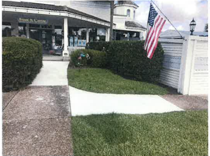
*Above Photo 2367 Repaired Sidewalks After Filling in Voids (January 2020)
