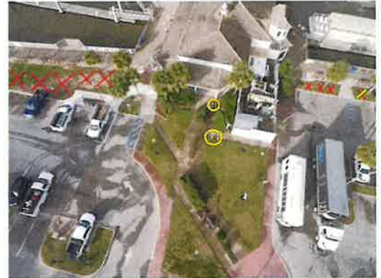
*Above Site Voids (January 2020)
