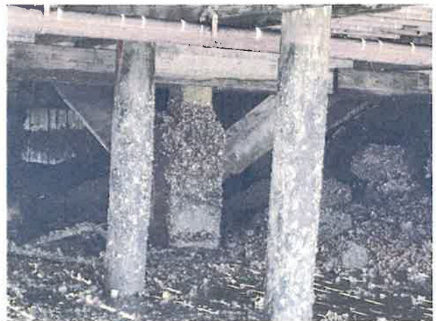
*Above Collapsed Double-T: Below Brett's Waterway Cafe (June 2020)
