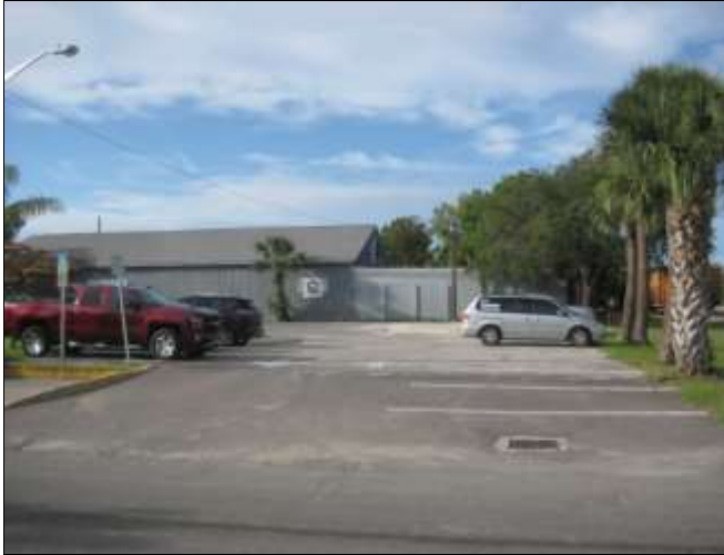
Subject parcel's driveway off Ash St.
