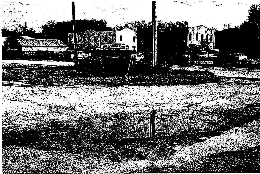
Exhibit F. Unimproved and deteriorating parking facilities in the proposed district.
