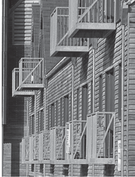
(fig. 4.52) Steel balconies projecting from wood shiplap siding wall.
