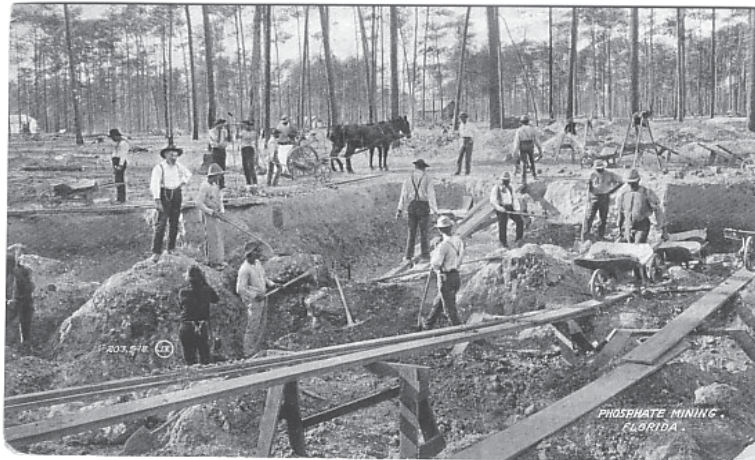
(fig. 2.19) Excavating phosphate in the Peace River area.
