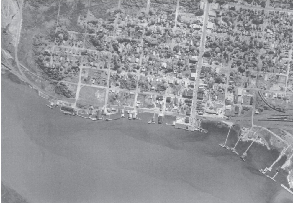
(fig. 3.2) Aerial view of Fernandina showing waterfront development before the advent of the port.
