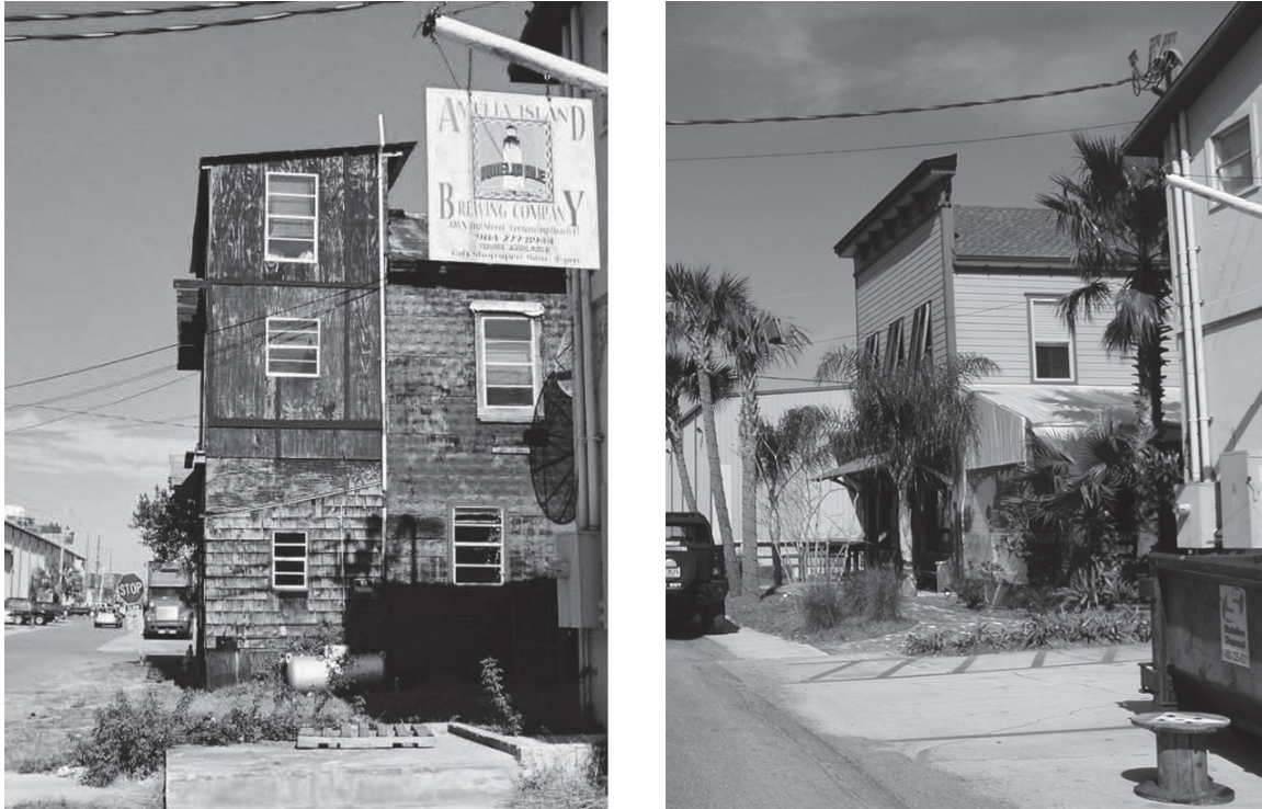
(fig. 3.8) View north along Second at Calhoun (before and after renovation).
