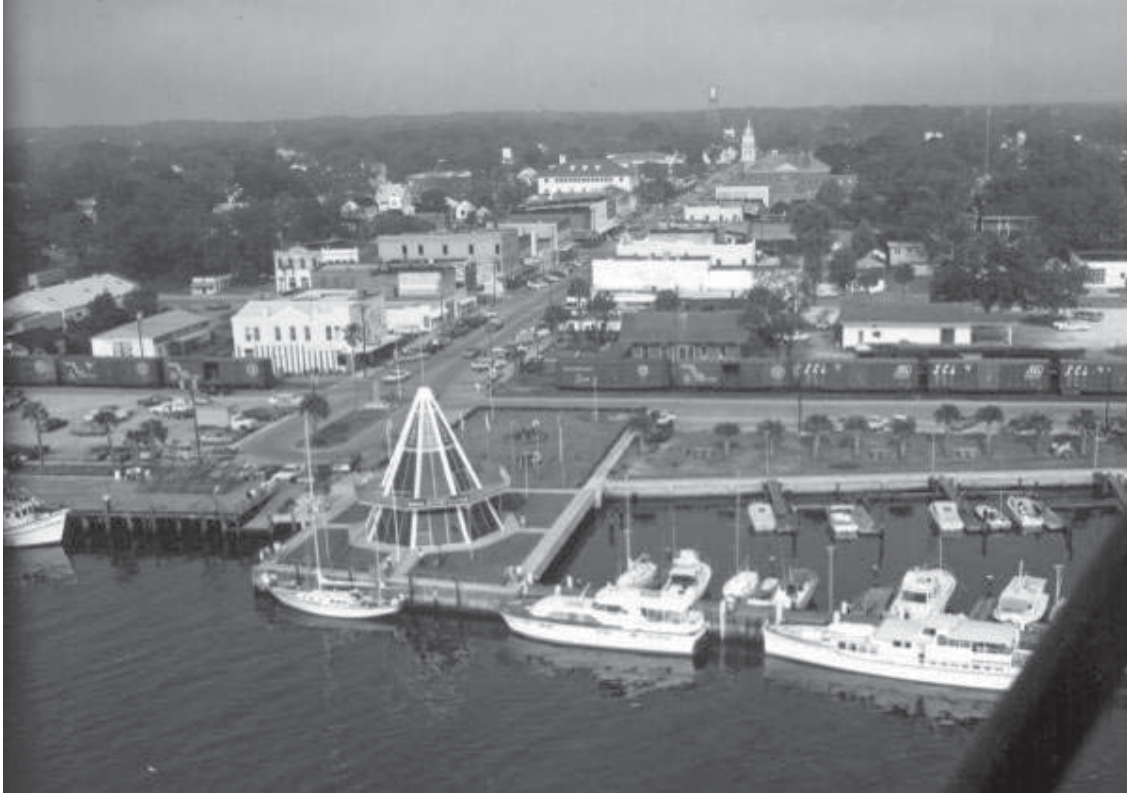
(fig. 2.29) Aerial view of the Welcome Station at the base of Centre Street.
