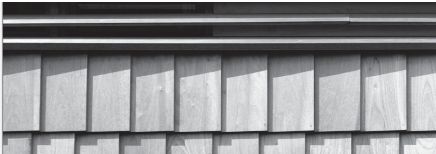
(fig. 4.33) Wooden lap siding detail (Machado+Silvetti).
