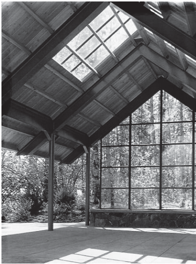
(fig. 4.9) Park pavilion with exposed structural system.
