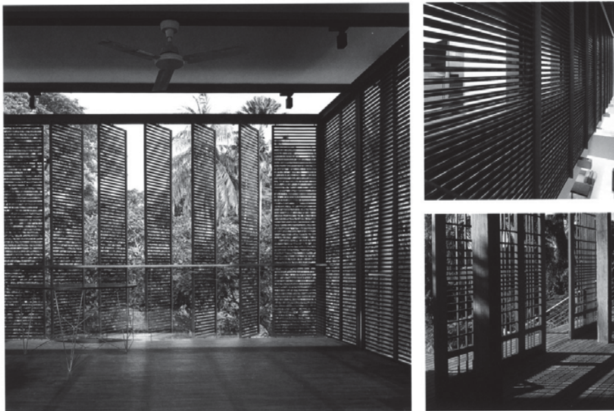
(fig. 4.68) Operable wooden louvers on these covered porches afford sun and privacy control without need for air conditioning.
