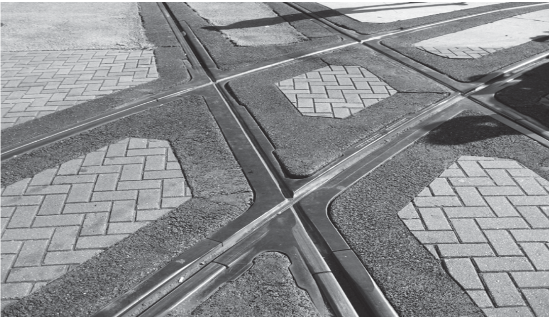
(fig. 3.16) Porous concrete-brick system providing transition between pedestrian surface and railroad (photo by Kevin Sullivan).
