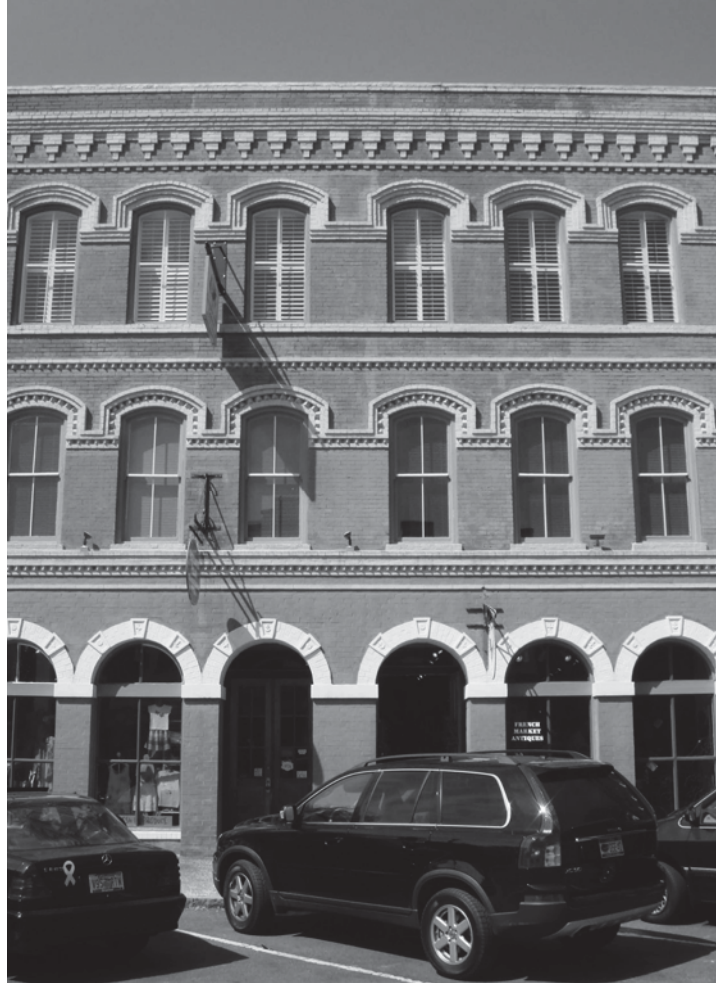
(fig. 4.64) Building façade in the Historic District along Second Street showing modulation of fenestration and depth of surface, as well as simple roof form.
