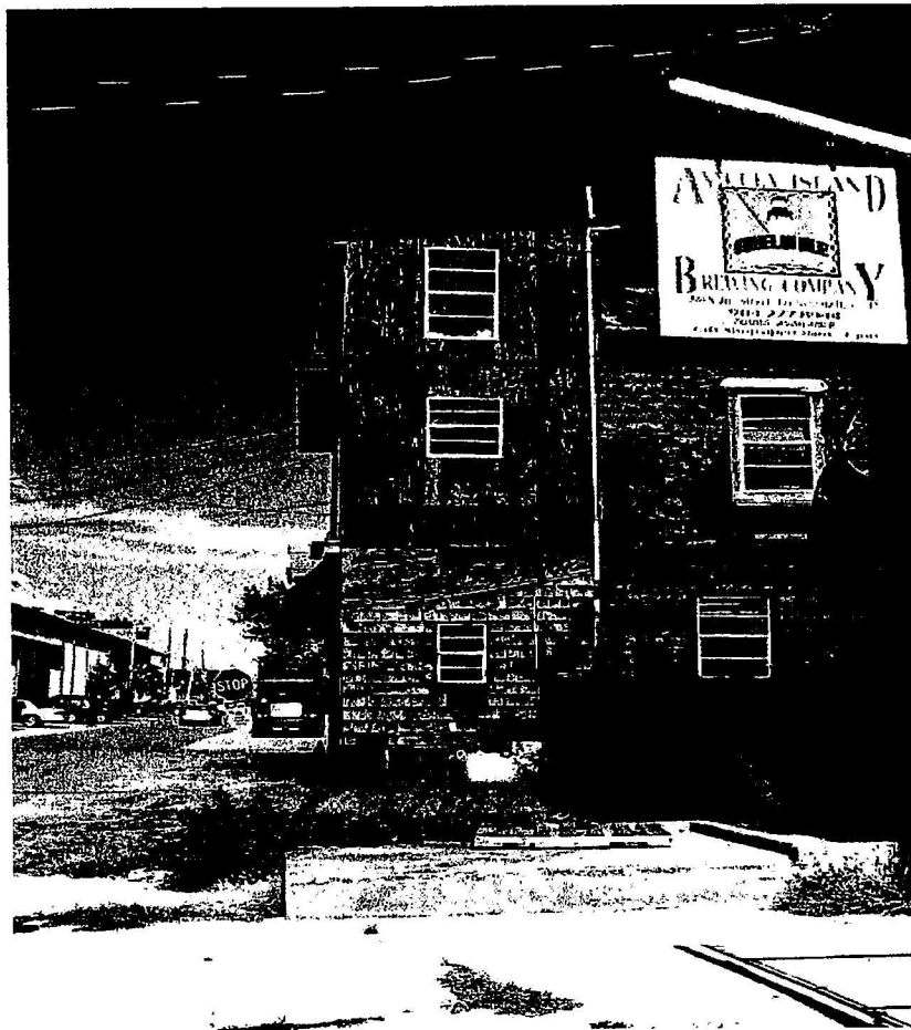
Exhibit G. Lack of sidewalks and other amenities do not promote a safe environment. Coupled with heavy industrial traffic, the residential use is not compatible with surrounding land uses. Dilapidation of structure is evident. (North 3 rd Street)
