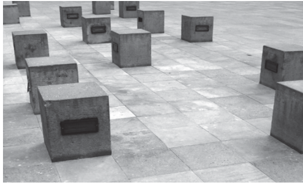
(fig. 5.15) Cast stone bollard-seats with integrated lighting in a public space.
