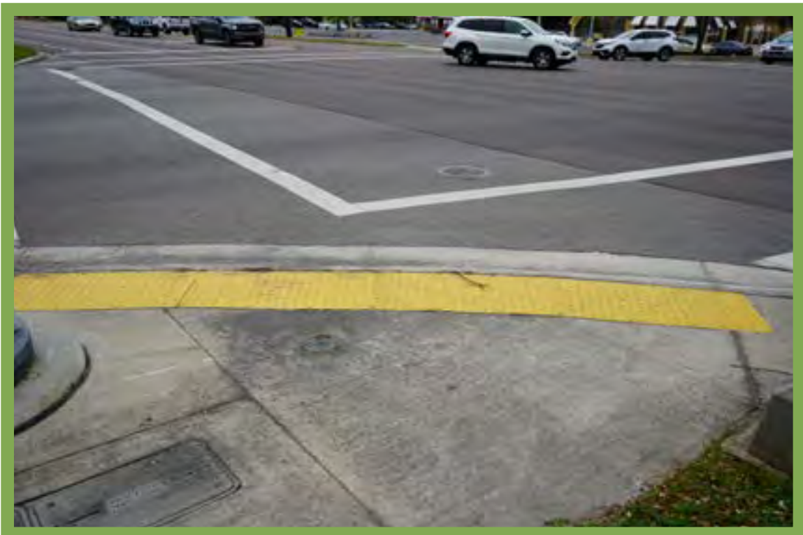
Sidewalk ramp on the southeast corner
