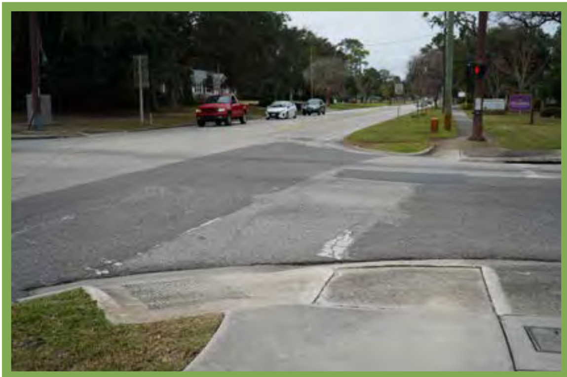
North crosswalk is not marked (westbound)
