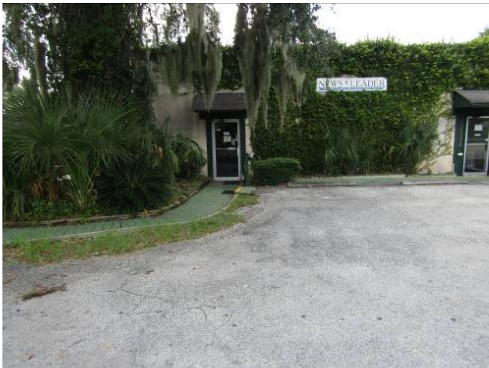
Photo #4. Between the building, the parking lot and Ash St., the feeder root system of the tree was almost completely covered.
