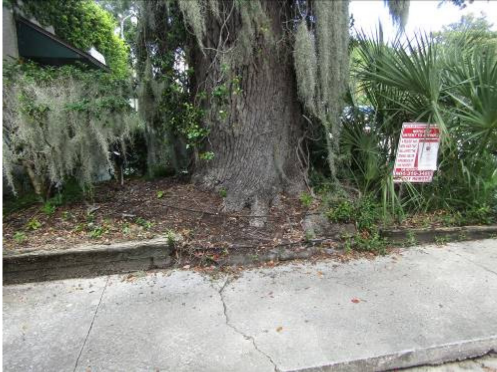
Photo #3. The tree was very close to the sidewalk in the front along Ash St. and was probably responsible for some breaking of the sidewalk. The sidewalk did not appear to be raised enough to be a trip hazard.
