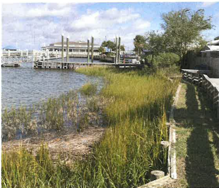
*Below image of existing timber bulkhead
