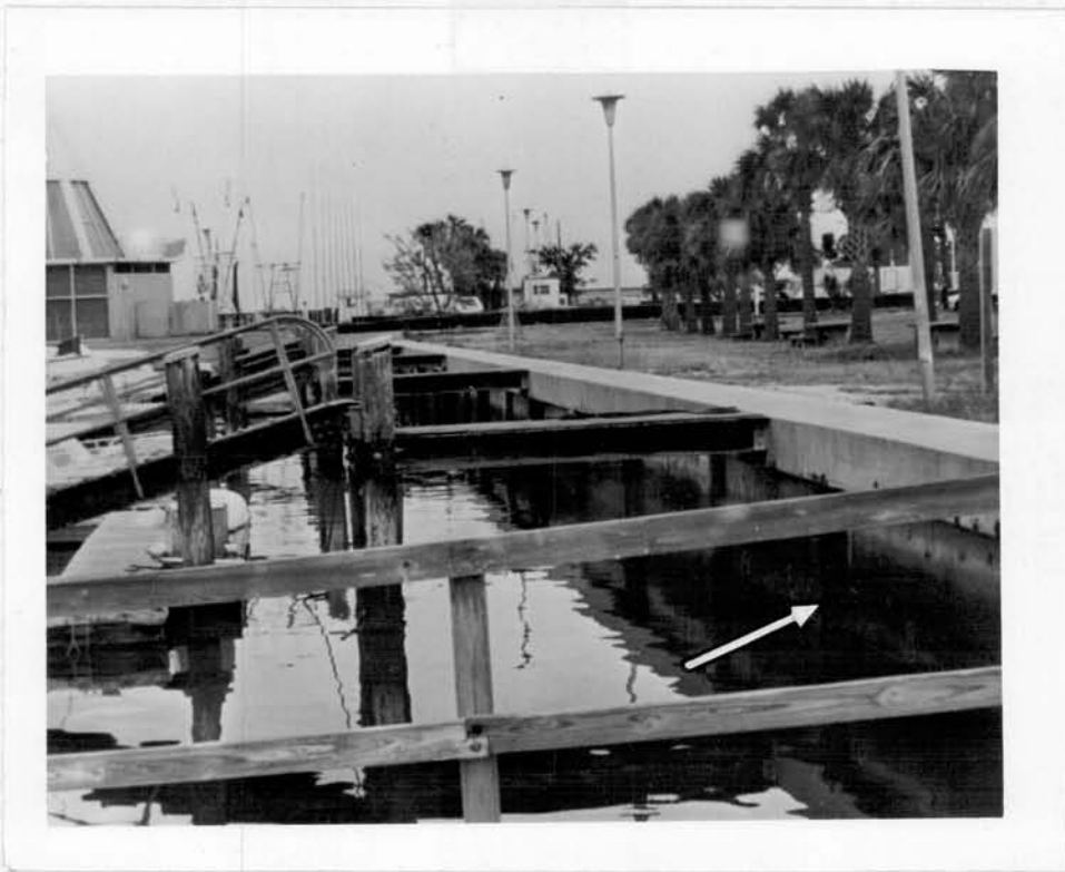
Fig. 4 Capped Bulkhead with King Piles (arrow) and Tee Sheeting
