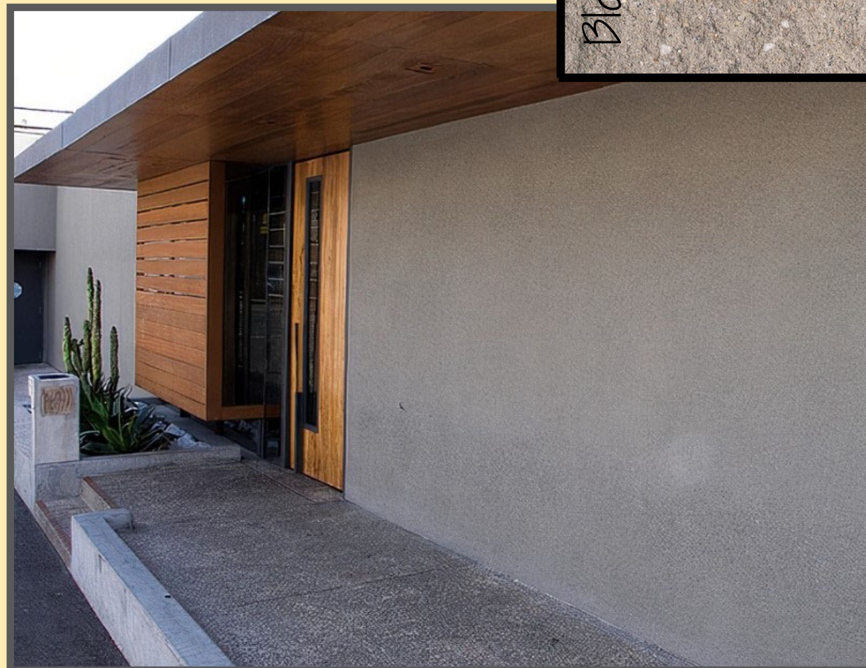
Kitchen / Bride Building Walls and Facia
