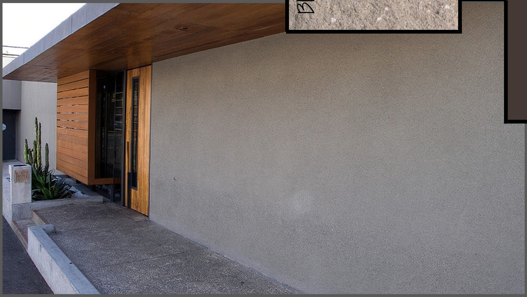
Kitchen / Bride Building Walls and Facia
