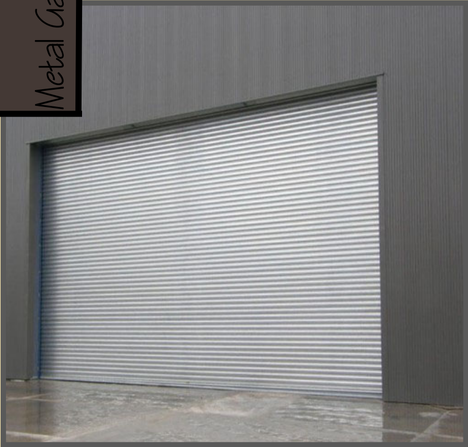
Adjacent Garage Building Walls & Door
