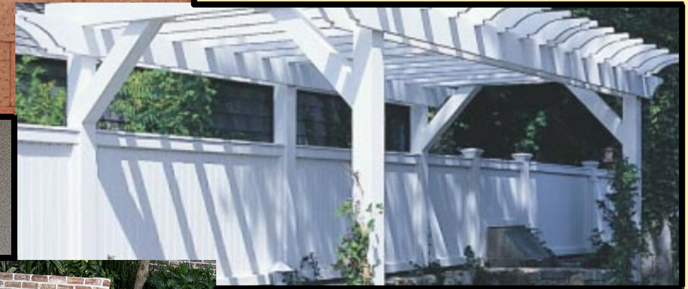
Pergola & Wood Fence
