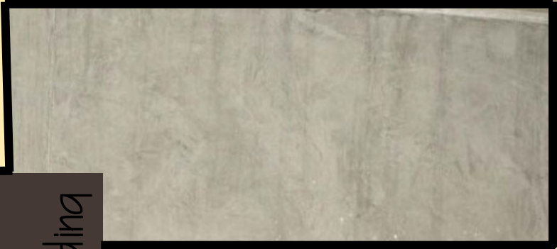
Concrete Kitchen Wall
