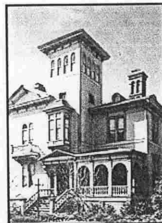
The Fairbanks House, built in 1885, was designed as an Italianate mansion, complete with piazzas and fountains.
