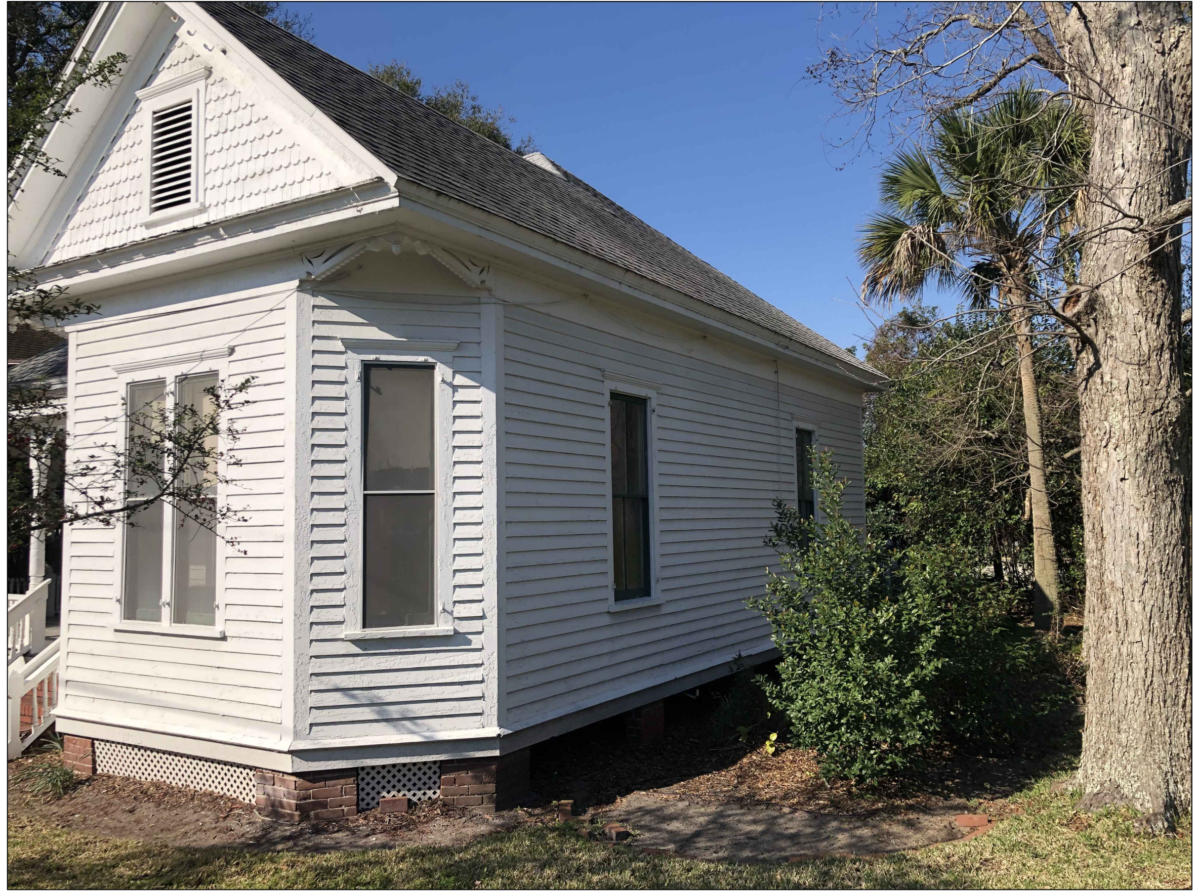
3 EXISTING NORTH VIEW OF 121 N 3RD ST.
