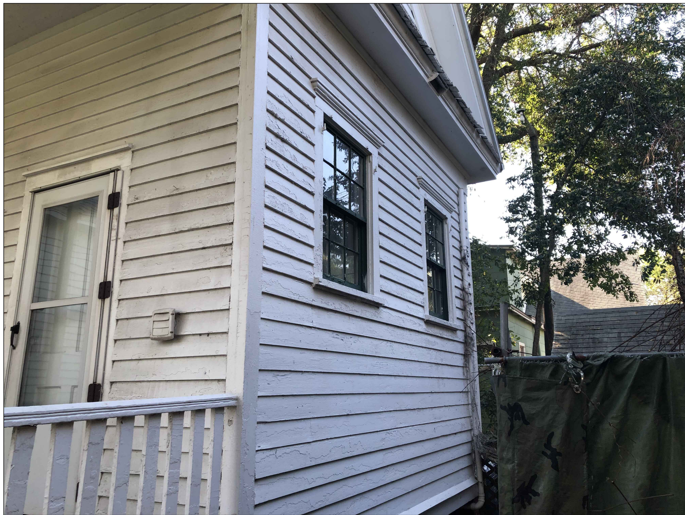
2 EXISTING WEST VIEW OF 121 N 3RD ST.
