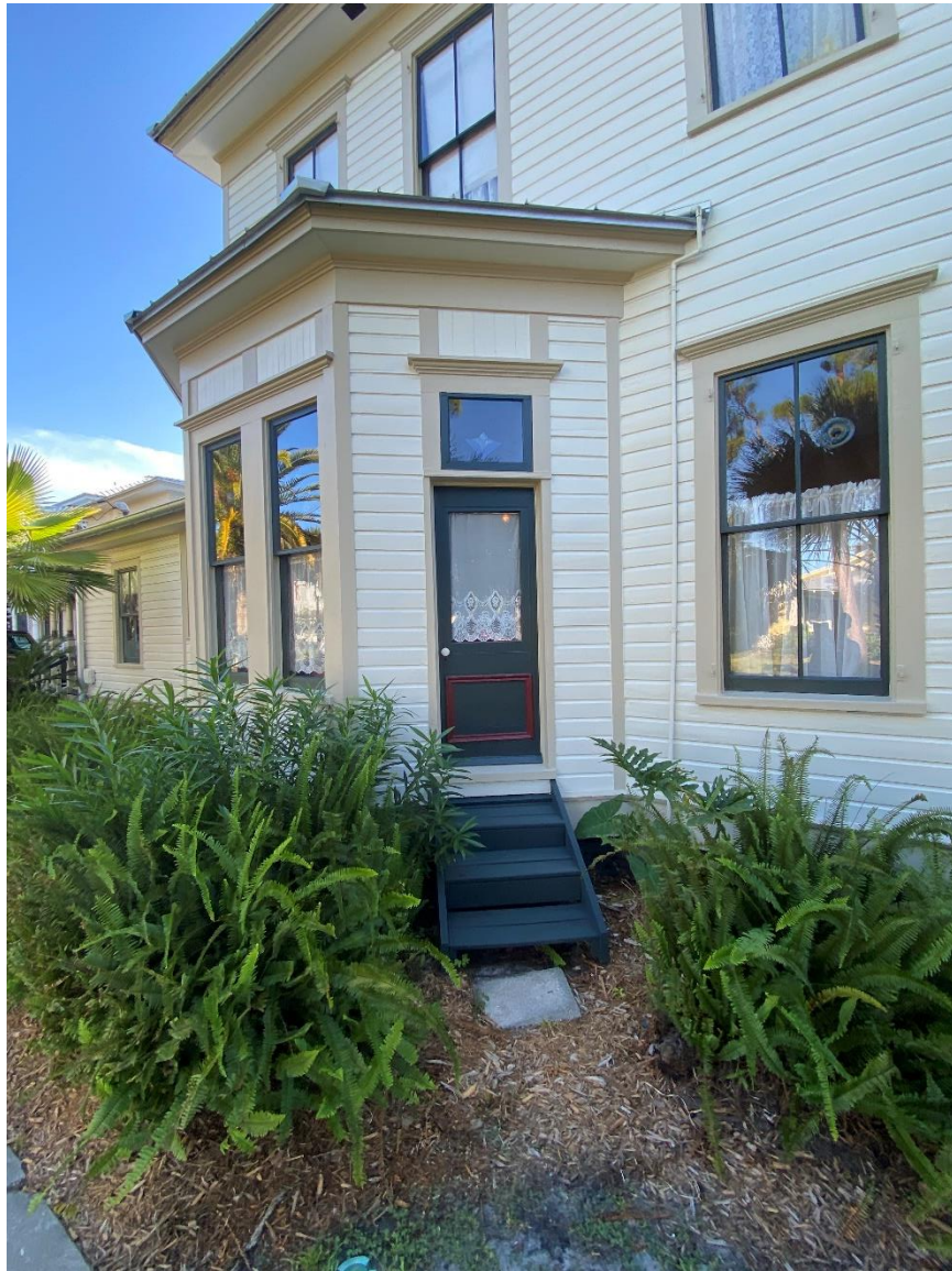
East side elevation at bay – door access to new porch
